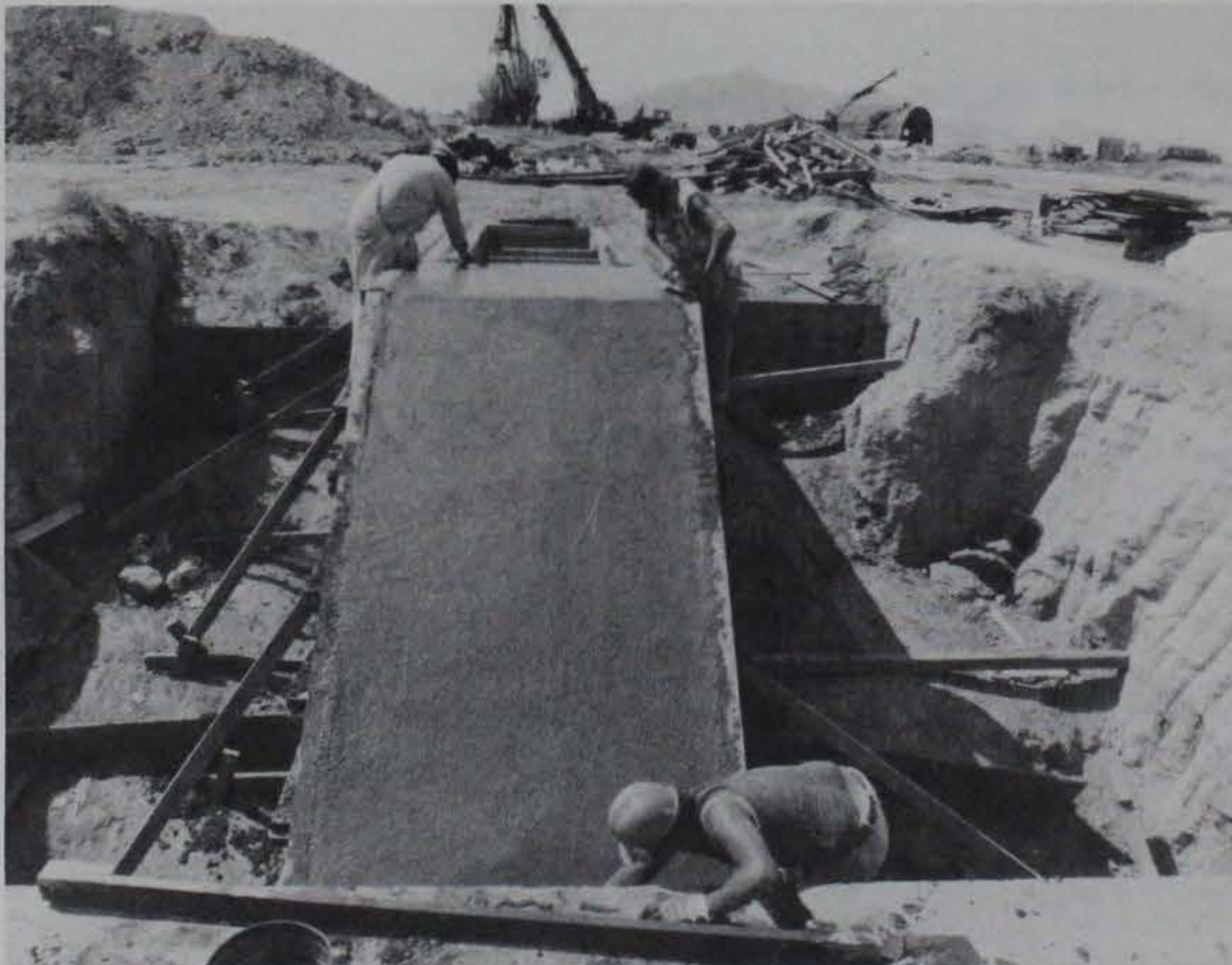
Figure 2.9. Finishing concrete in stairwell roof.
