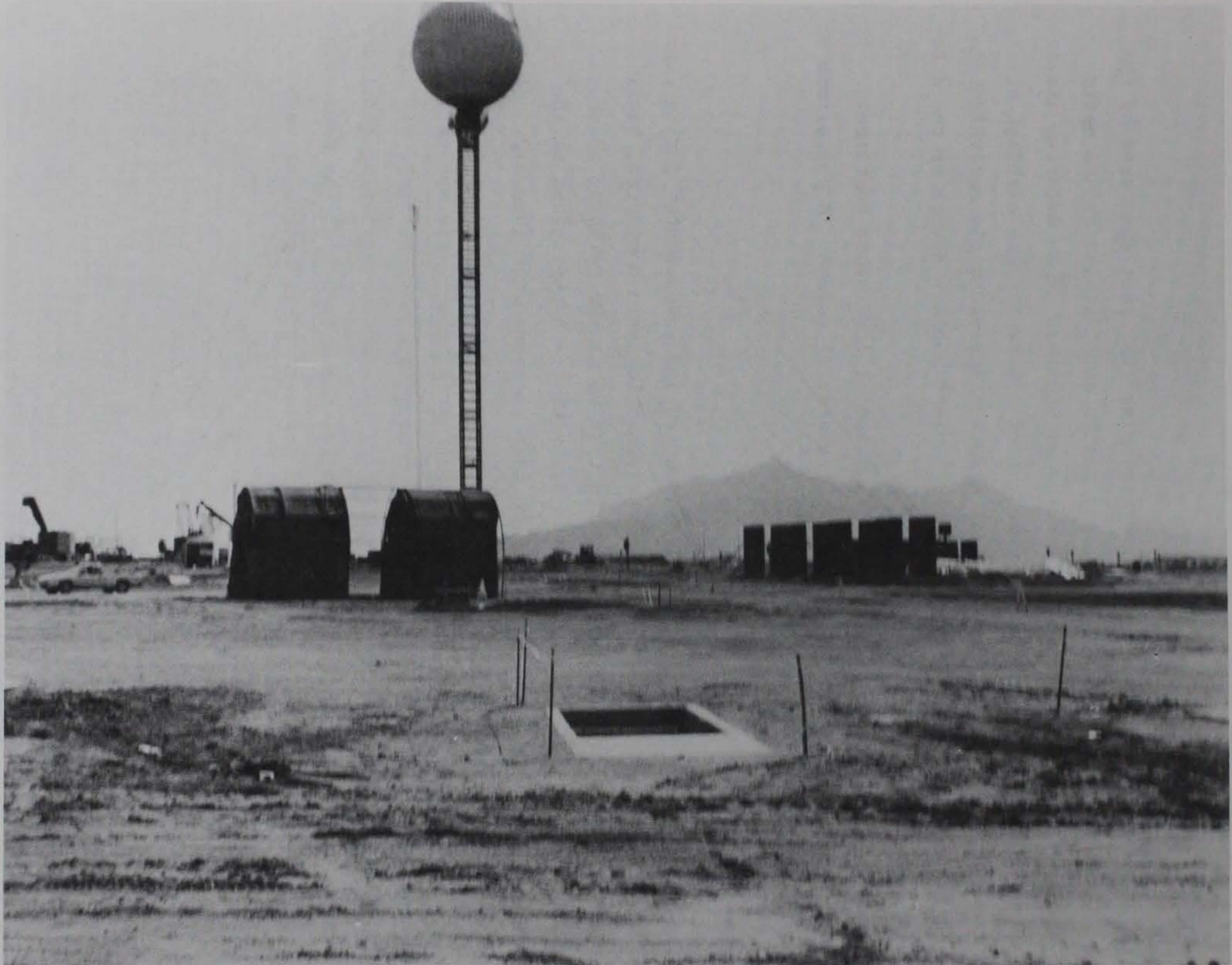
Figure 3.1. DIRECT COURSE charge tower assembly (closure and entryway test in foreground).
