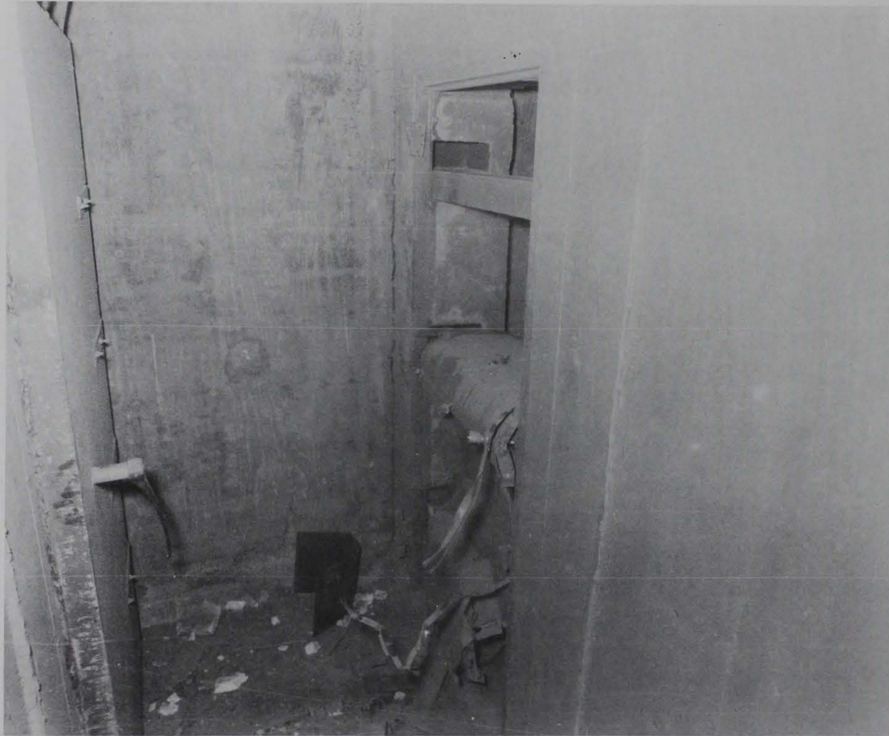
Figure 4.5. Closures, reinforced concrete blast door on left, commercial door on right.
