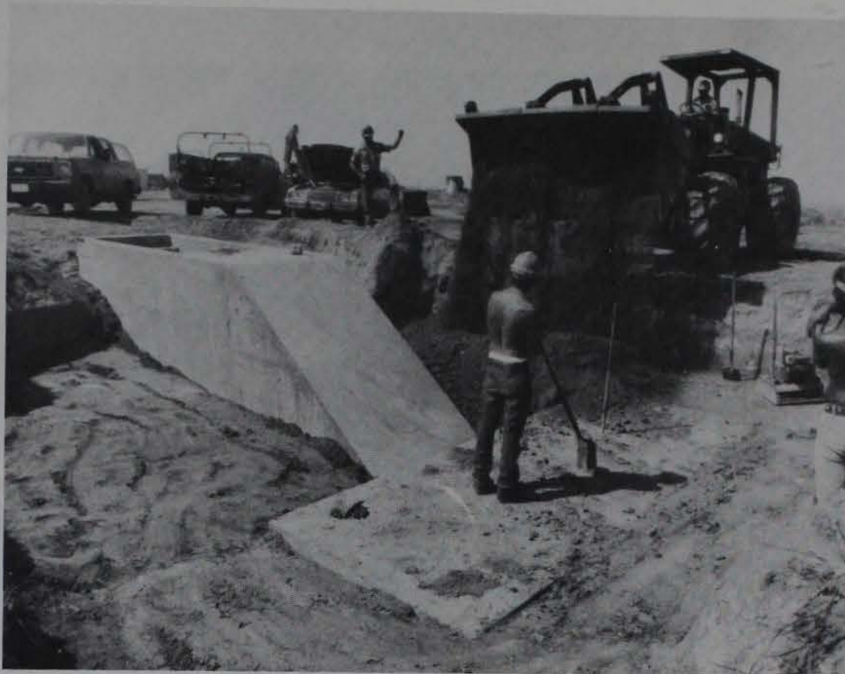
Figure 2.10. Backfill placement around completed structure.
