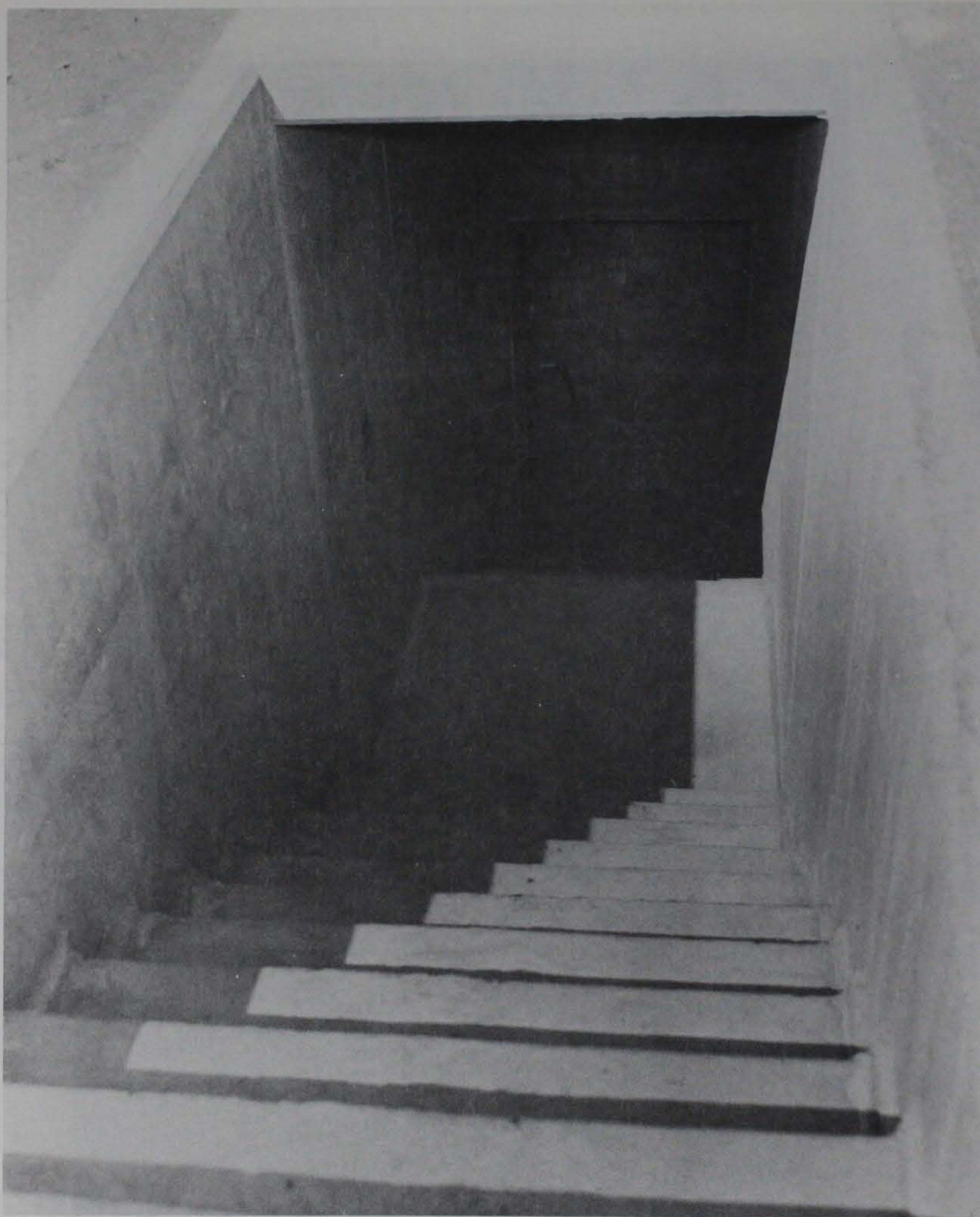
Figure 3.3. Surface view of full-scale entryway (closures on left and right at bottom of tunnel).
