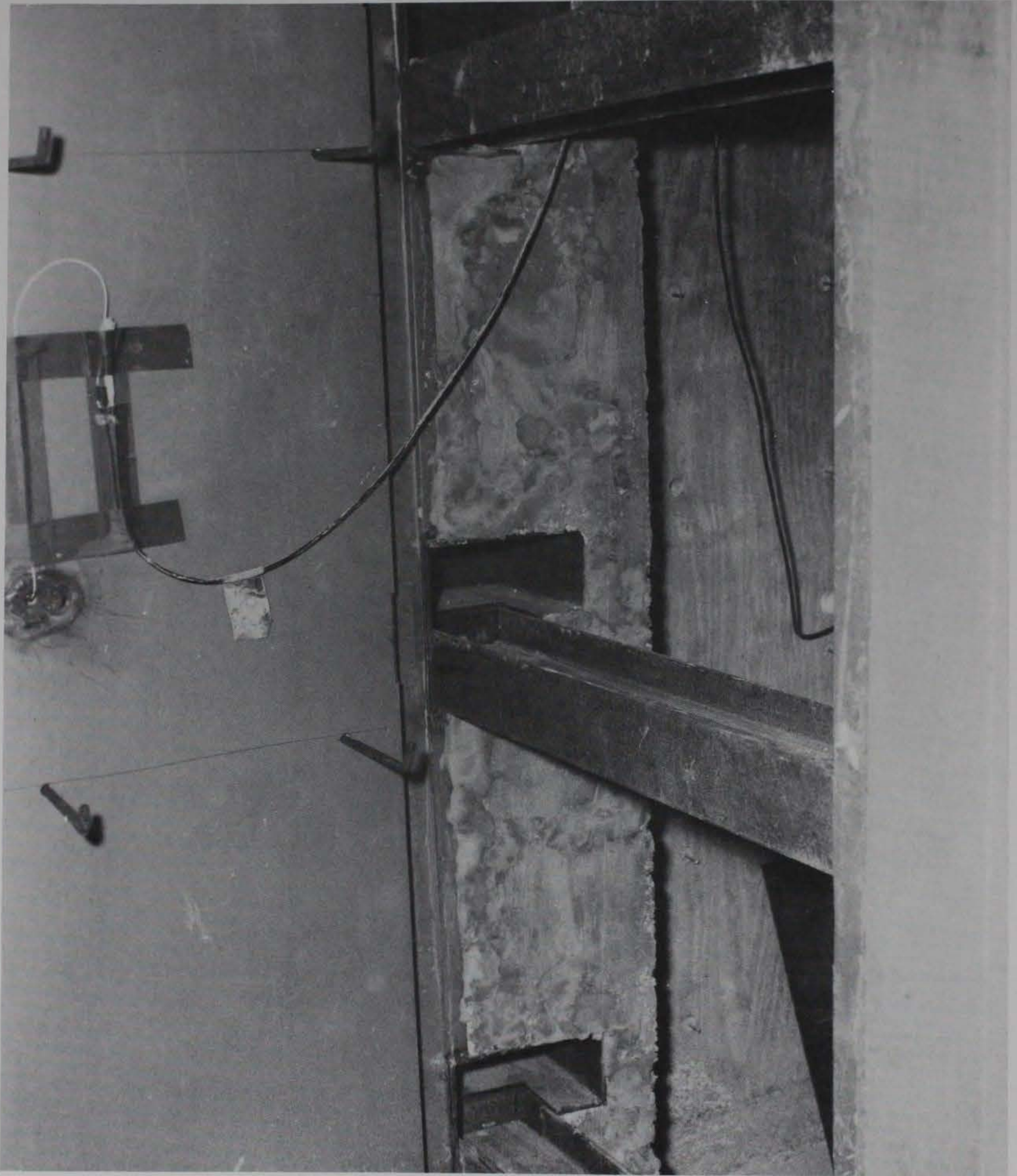
Figure 2.16. Commercial door (on left, open) with support beams in place.
