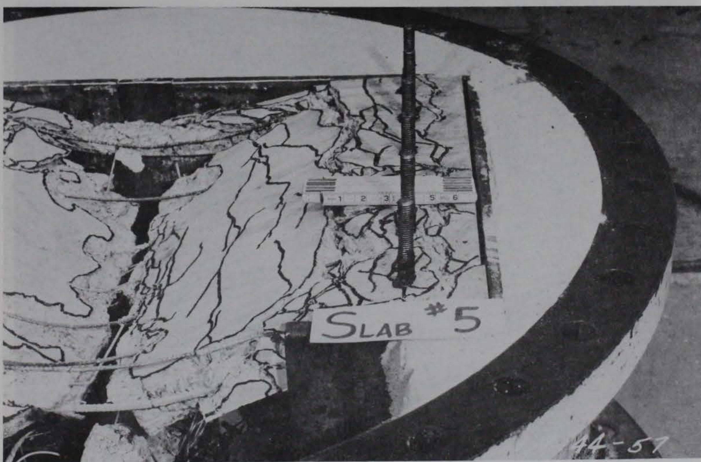
Figure 4.13. Closeup view of Slab 5, posttest.
