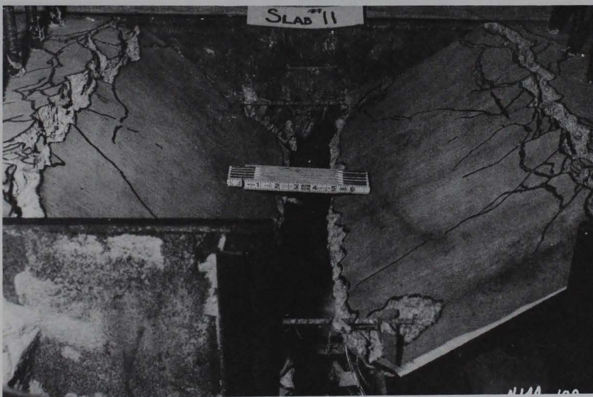
Figure 4.25. Closeup view of Slab 11, posttest.
