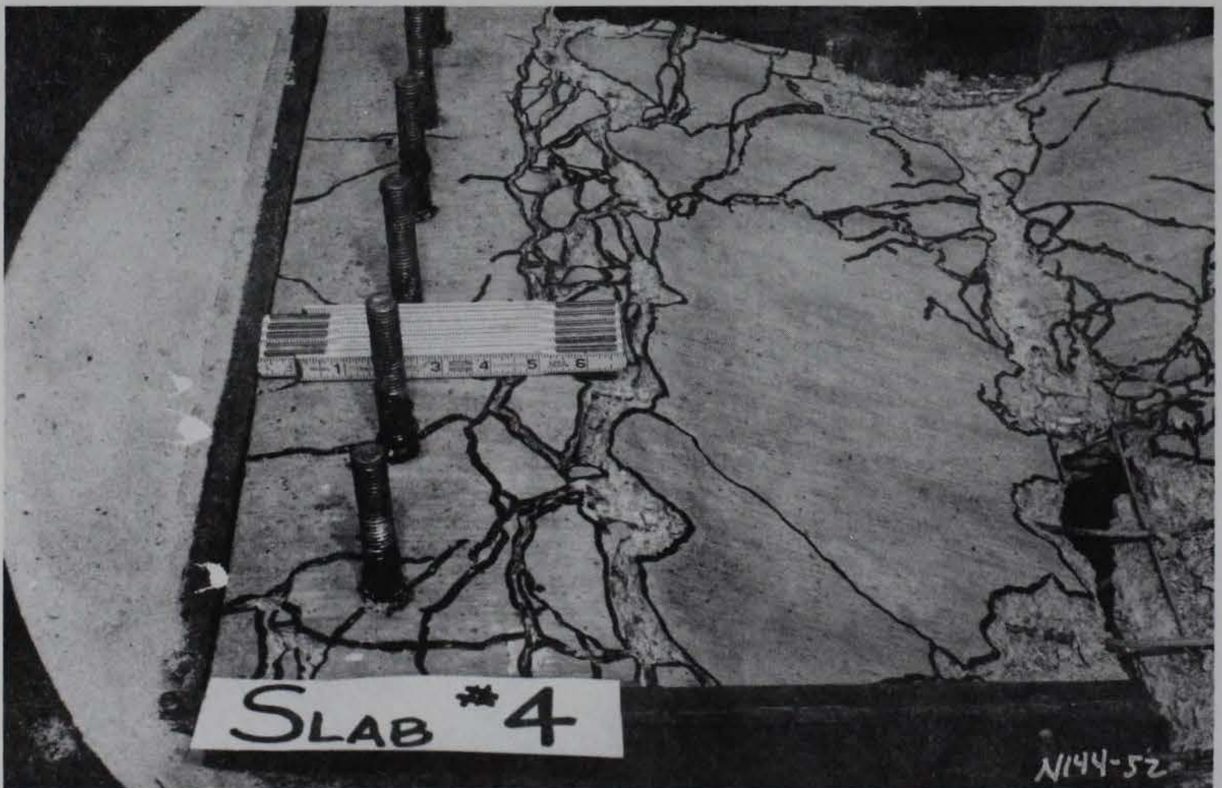
Figure 4.11. Closeup view of Slab 4, posttest.
