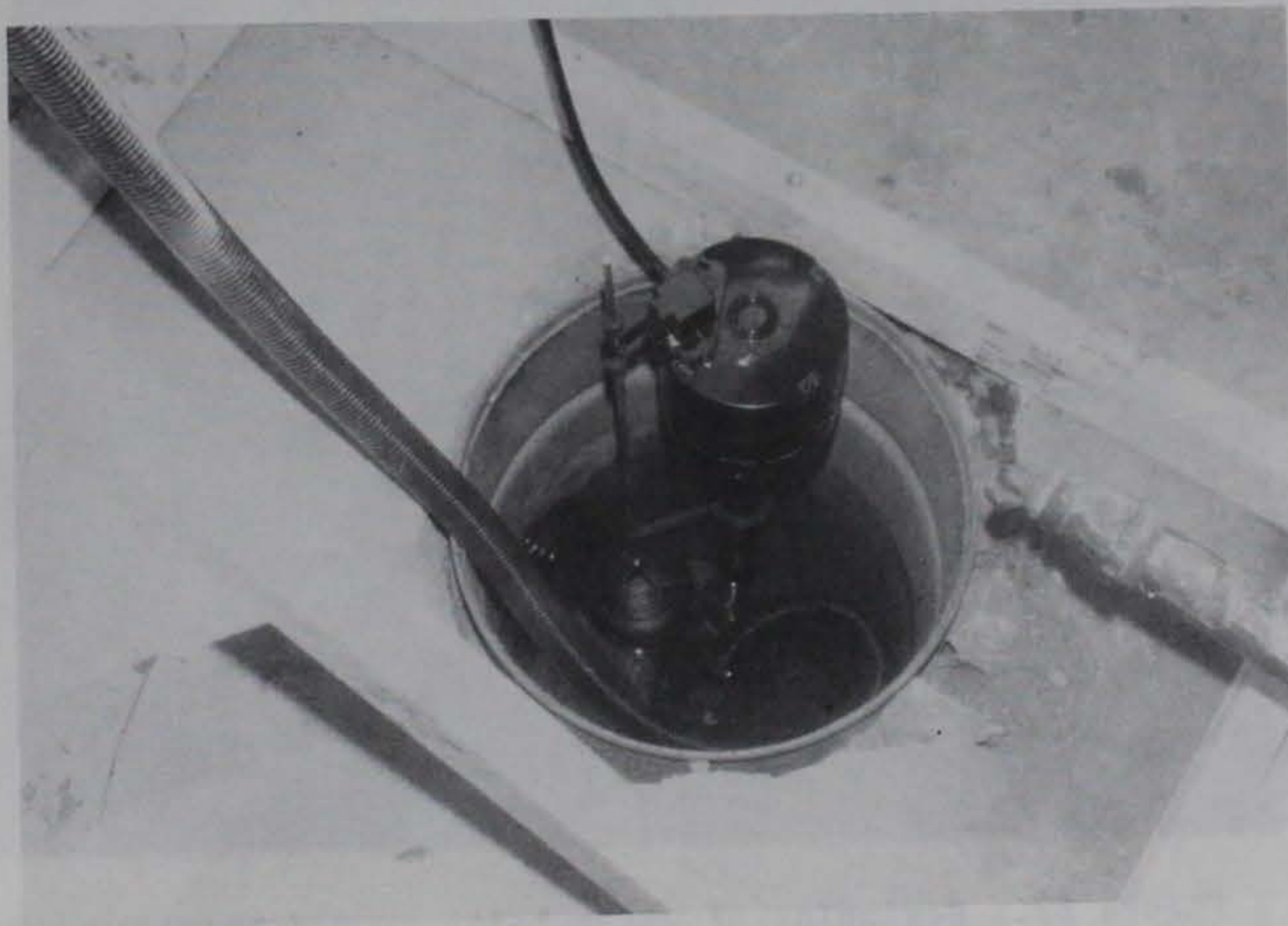
Figure 60. Sump which collects underseepage
