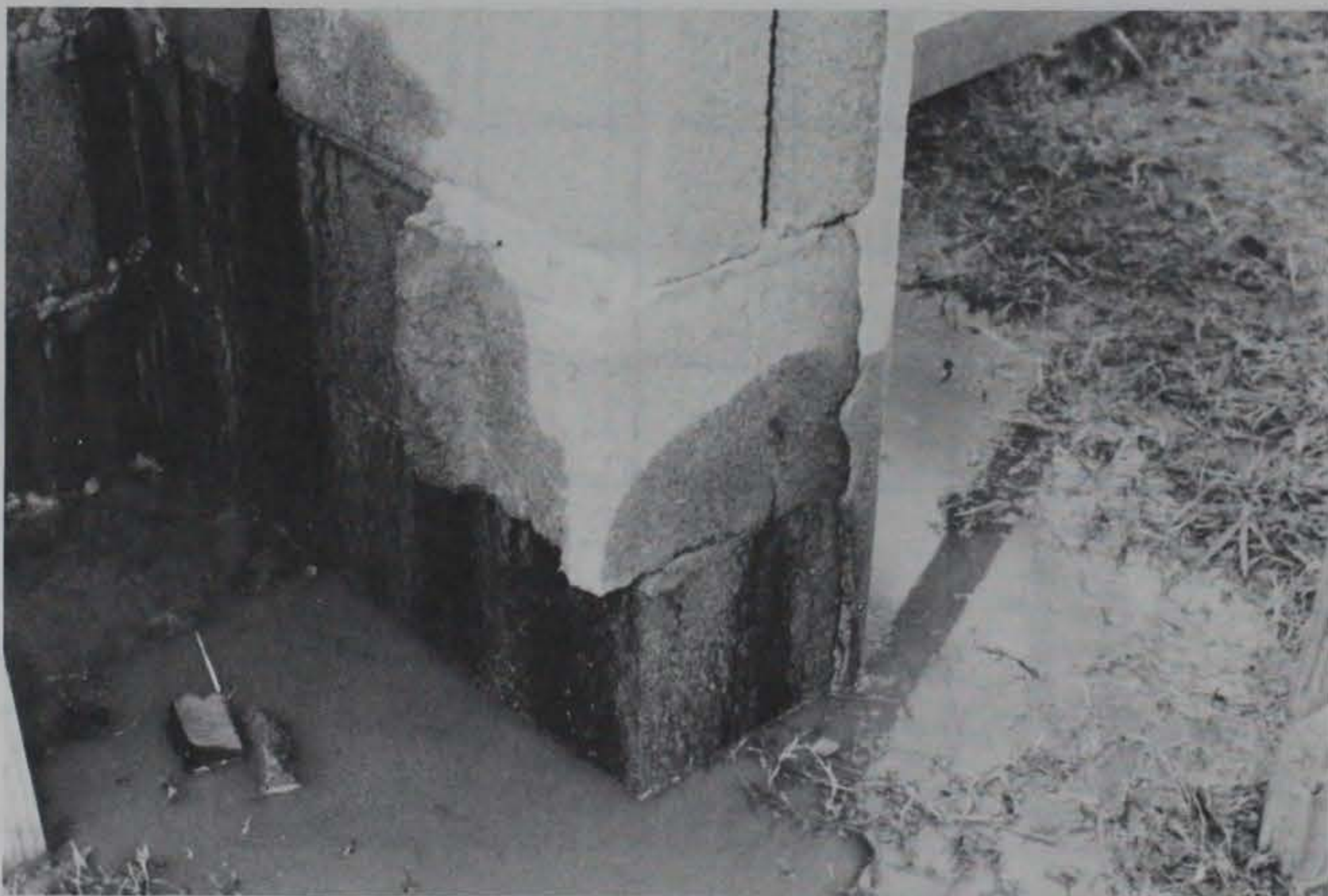
b. Base of wall
