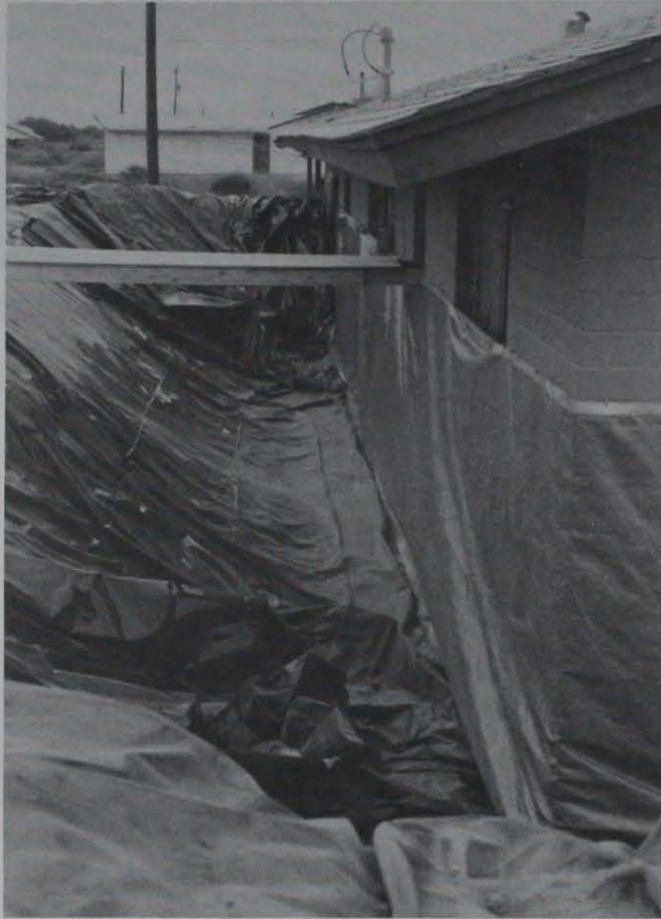
Figure 29. Plastic-over-earth berm extending down and under aluminum sealing strip
