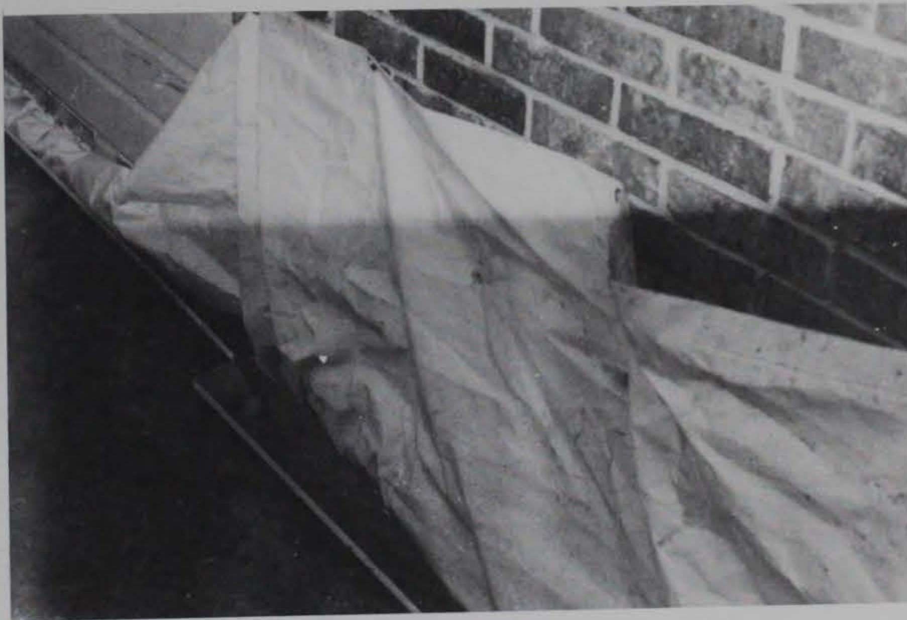
b. Membrane being pulled up and connected to house
