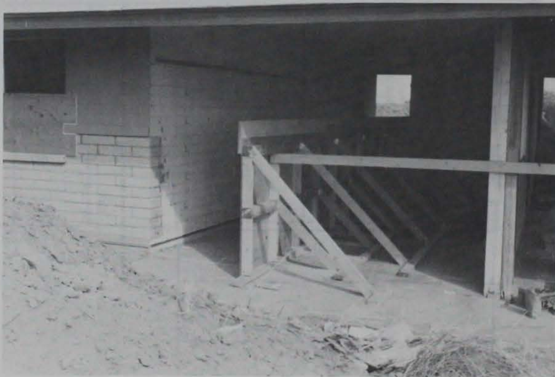
Figure 27. Plywood bulkhead
