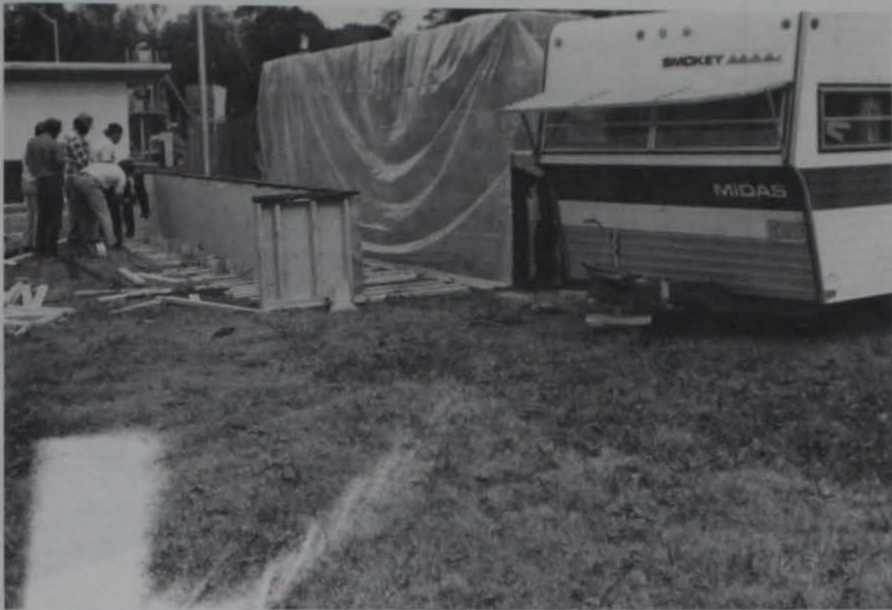
a. Being prepared for testing
