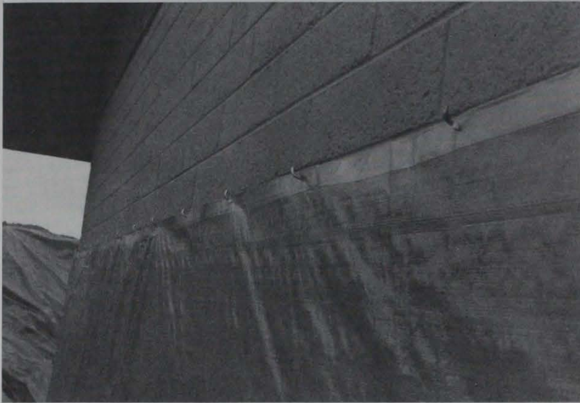
Figure 31. Hooks holding reinforced plastic sheeting
