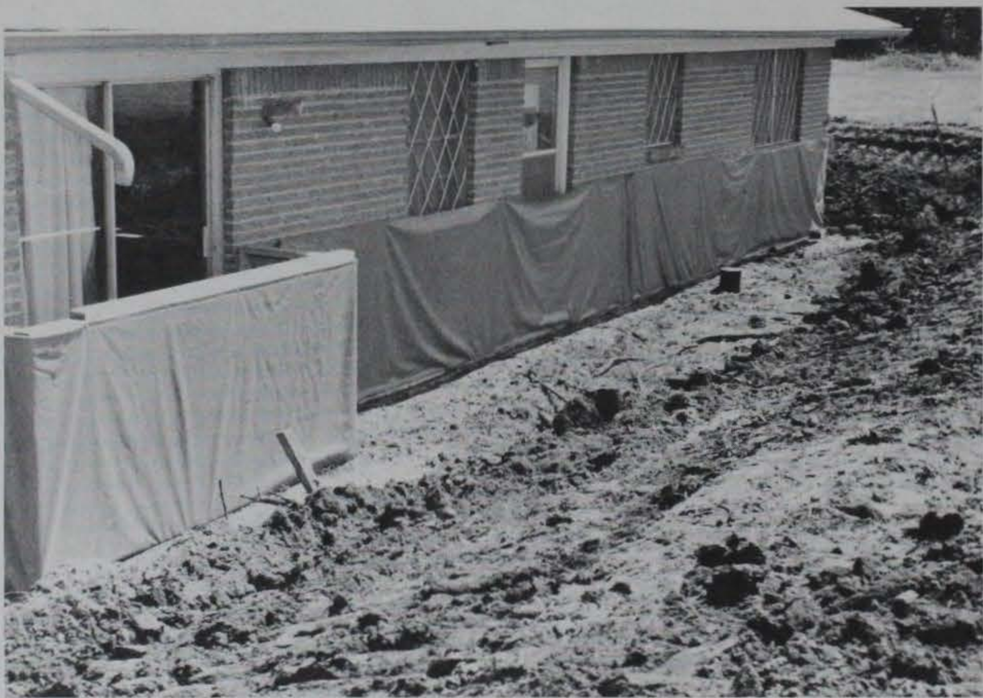
Figure 55. Vinyl-coated nylon fabric used in preparing house to resist floodwaters
