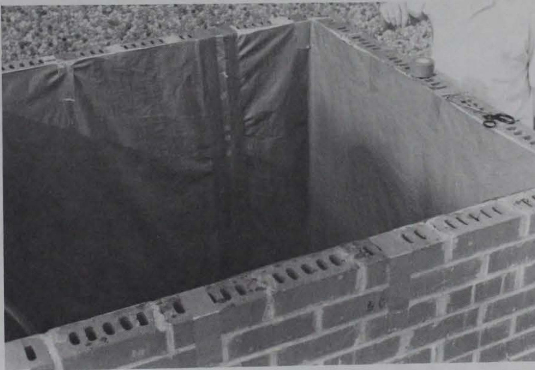
b. Plastic sheeting covering brick wall
