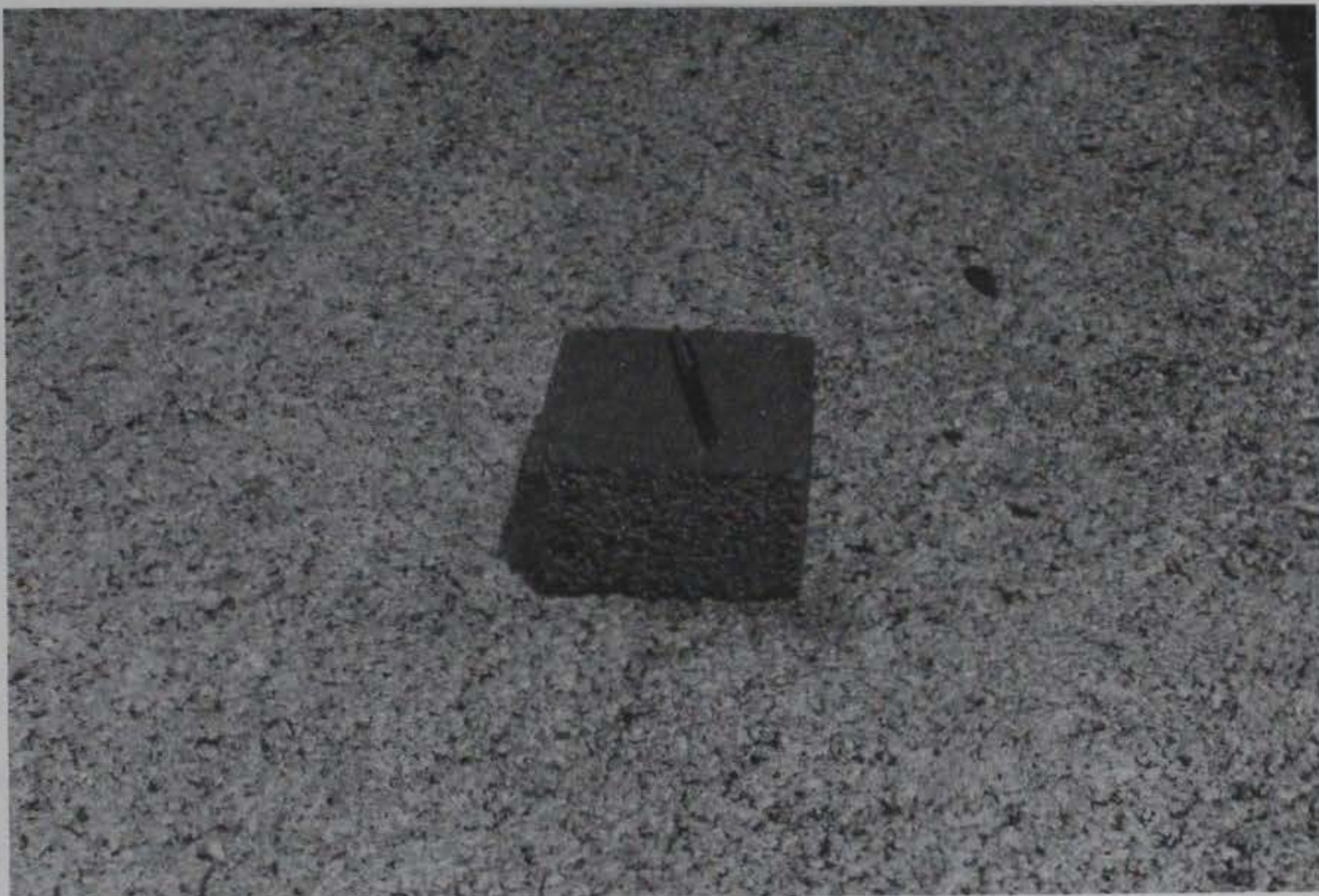
Figure 5. Smoother surface textures resulting from overlays of finer aggregate mixtures (as shown by block)
