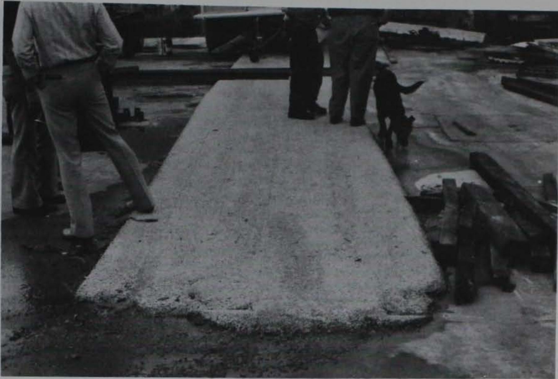
Figure 6. Overall view of skid resistance test strip of pervious concrete
