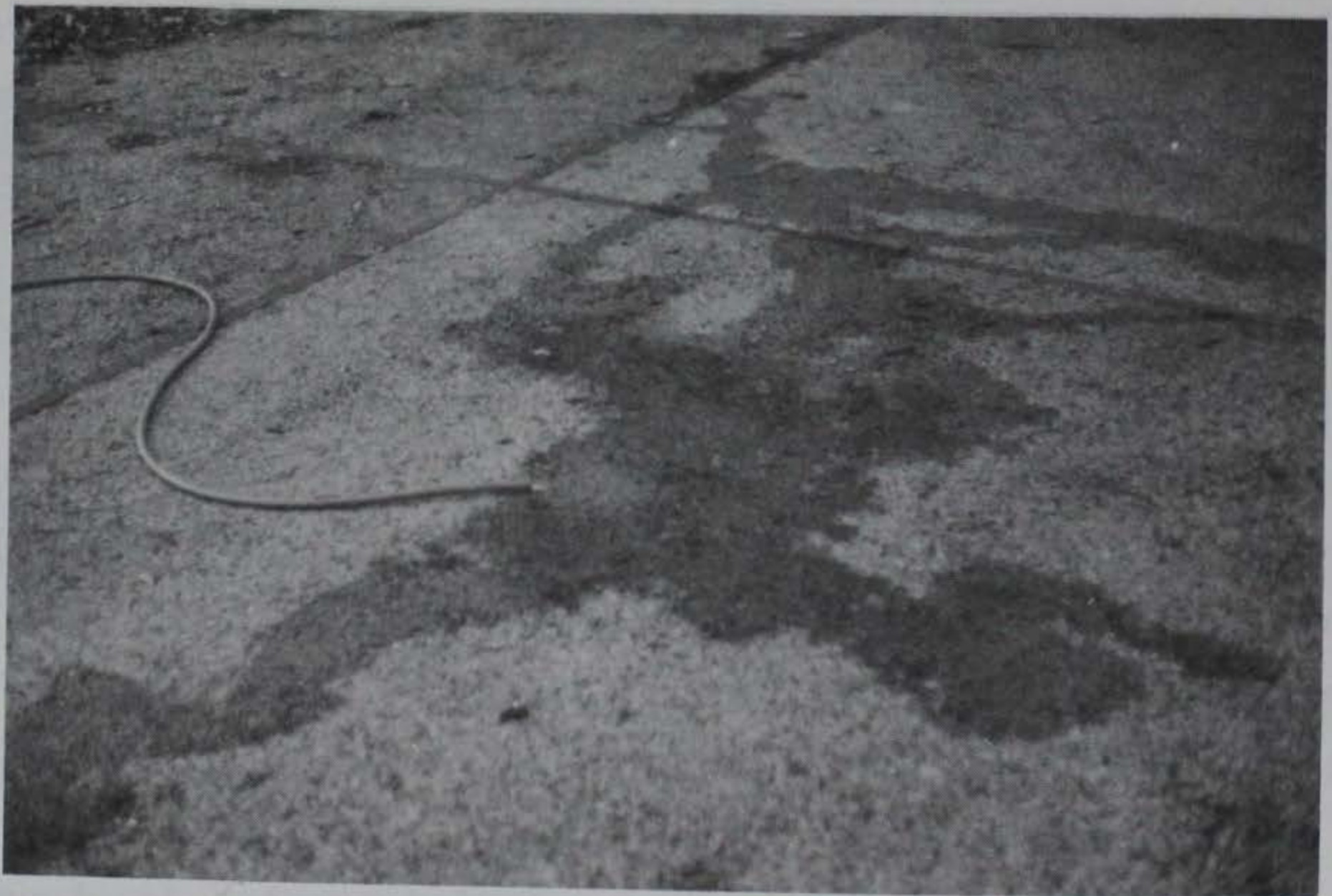
Figure 3. Drained surface of parking lot shortly after flooding
