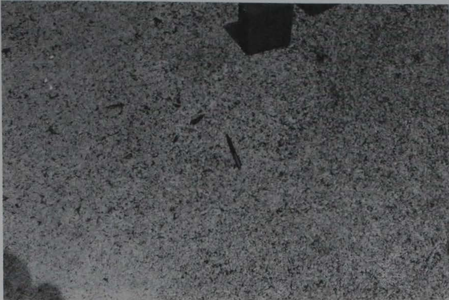
Figure 4. Reasonably smooth, open texture on parking lot
