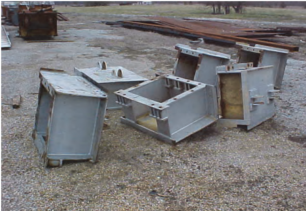
Figure 7. Stop log extensions used for the Little Sunflower Flood Control Drainage Structure. (Furnished by USAED Vicksburg.)
