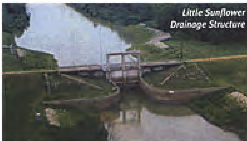
Figure 5. The Little Sunflower Flood Control Drainage Structure (from Mississippi Levee Board 2012).
