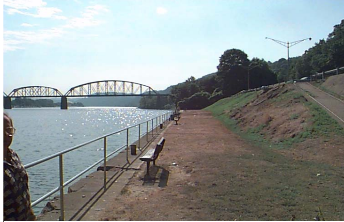
Figure 4. Old Lock 2 guide wall and portion of lock chamber wall, looking upstream
