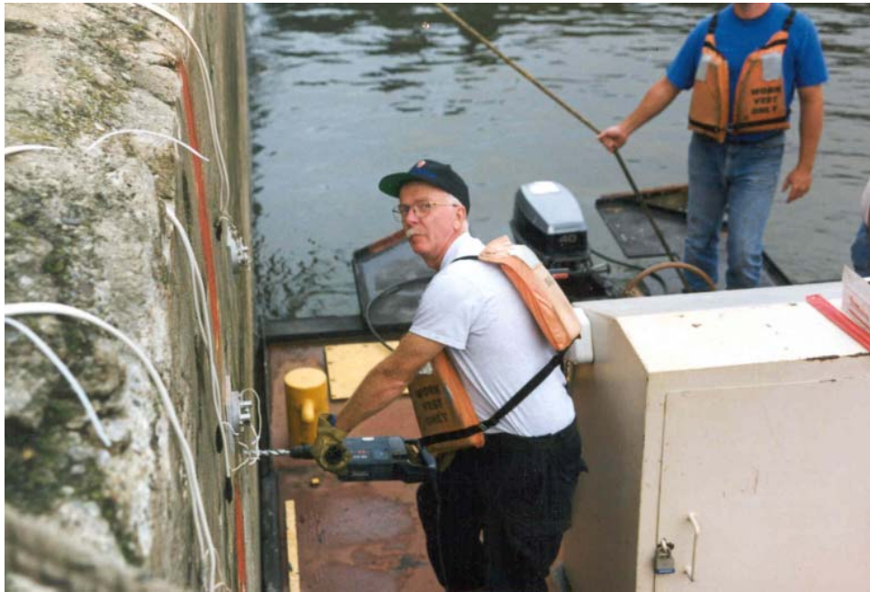
Figure 19. Installation of bumpers on lock wall
