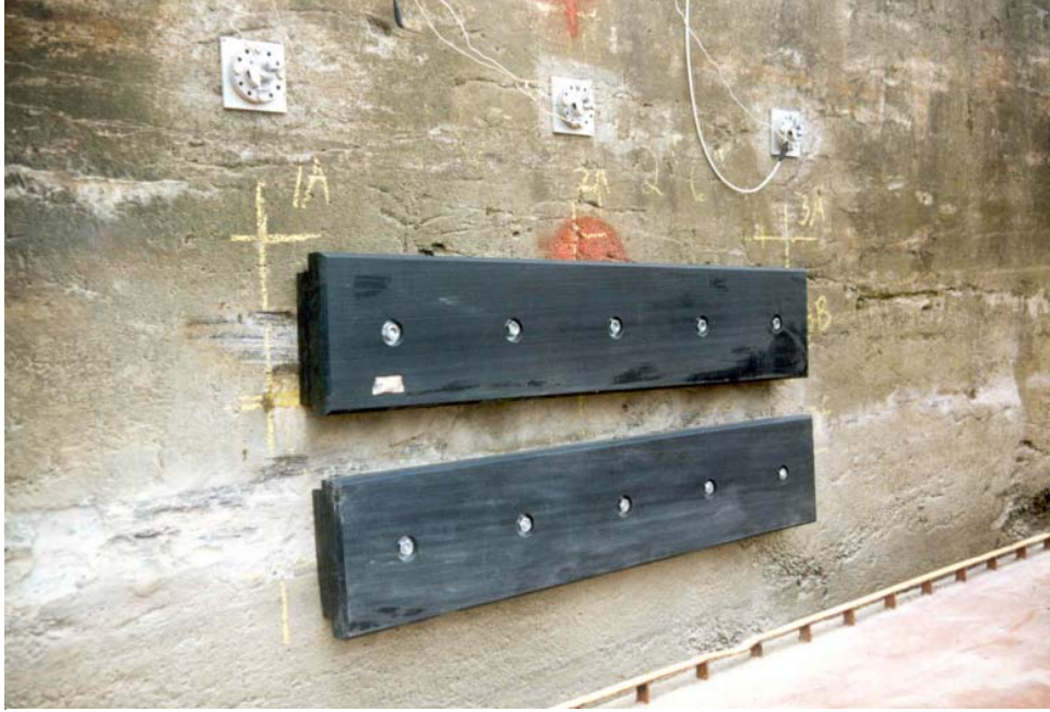
Figure 20. Final setup of UHMW bumpers
