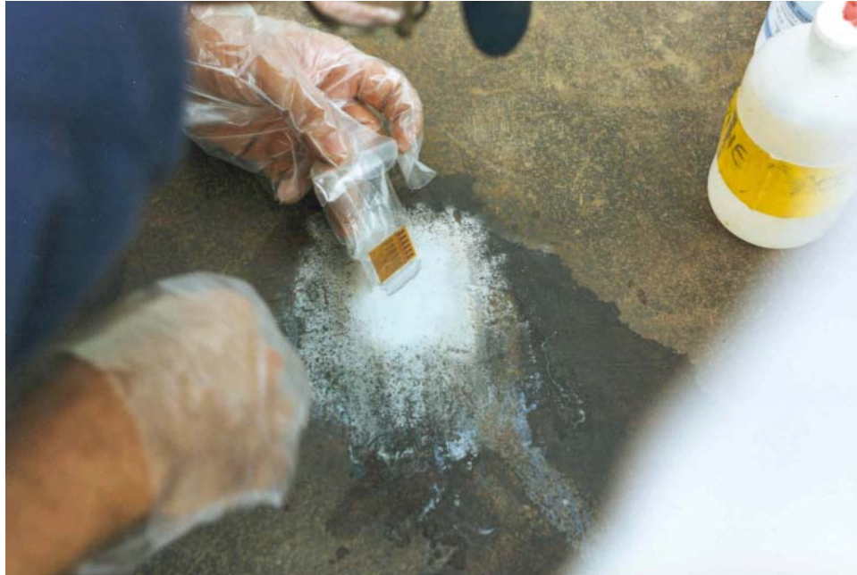
Figure 13. Installation of strain gages on top of deck
