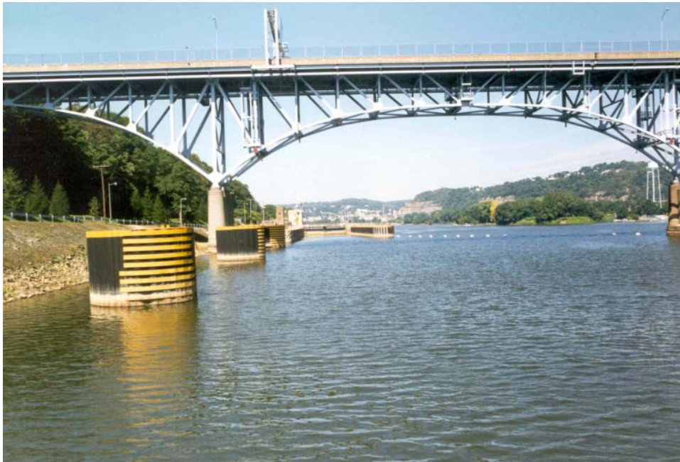
Figure 1. Looking downstream from Old Lock 2 to Lock and Dam 2
