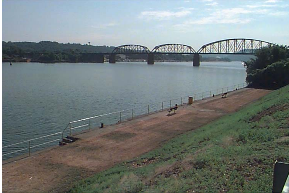
Figure 2. Old Lock and Dam 2, Allegheny River
