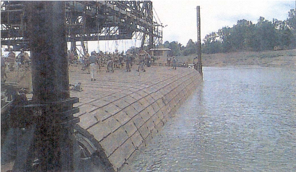
Figure 22. Machinery for laying articulated mattresses on riverbanks
