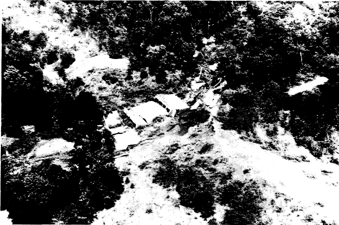
Figure 11. Unsatisfactory performance of a box culvert structure
