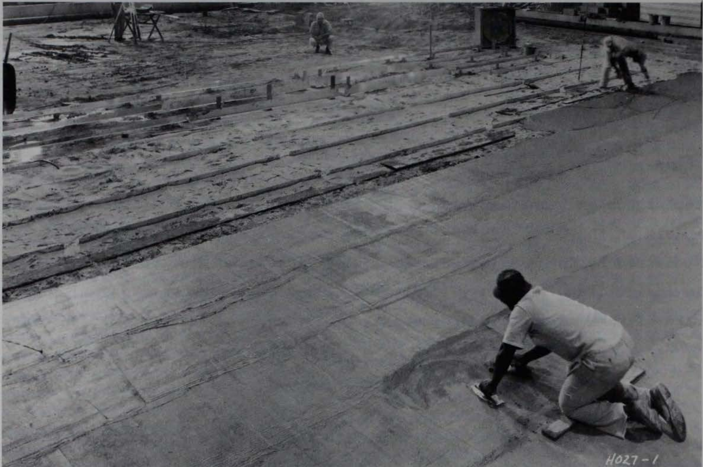
Figure 1. Cement paving to sheet-metal templates
