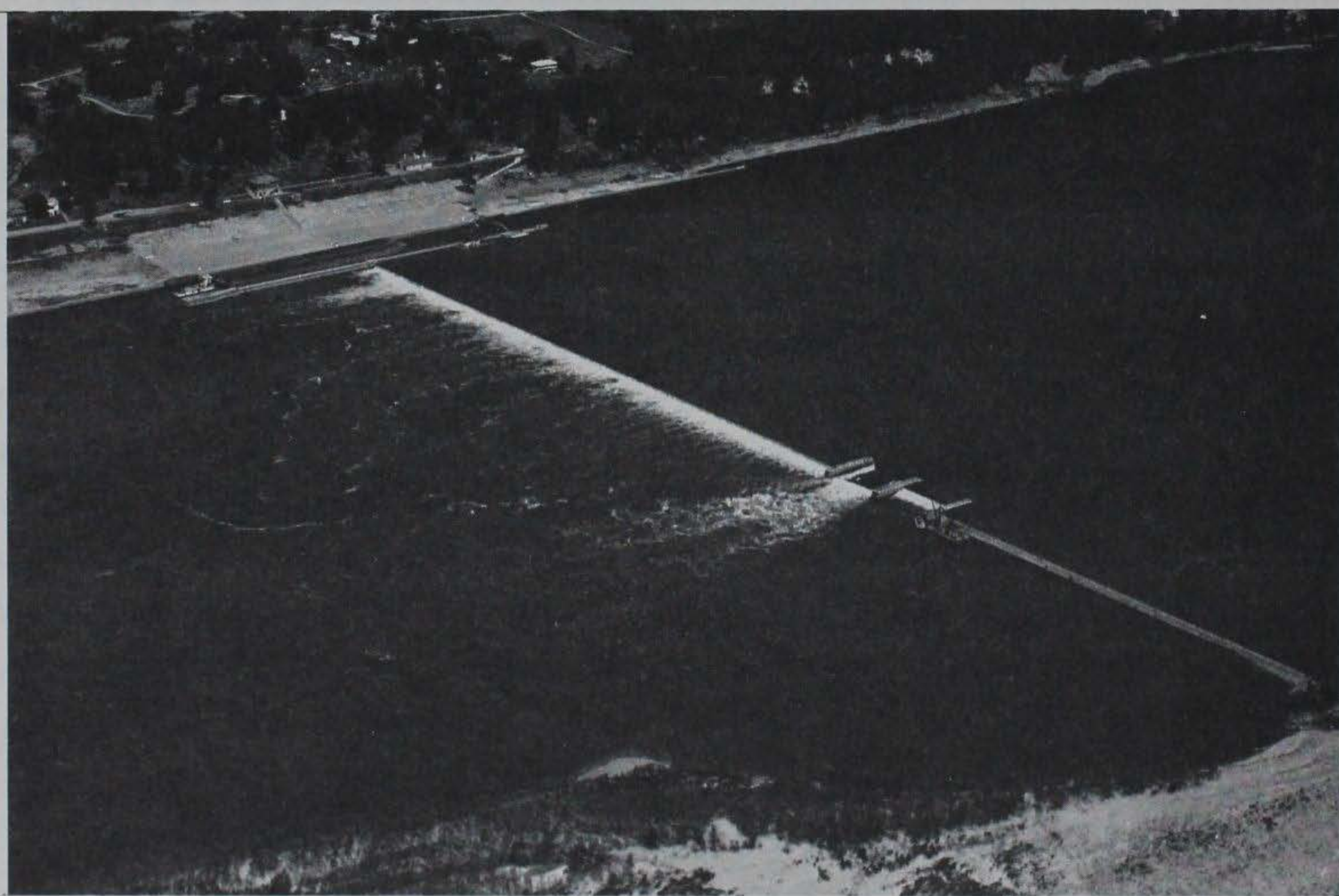
Fig. 1. Lock and Dam 51 on the Ohio River near Golconda, Illinois
