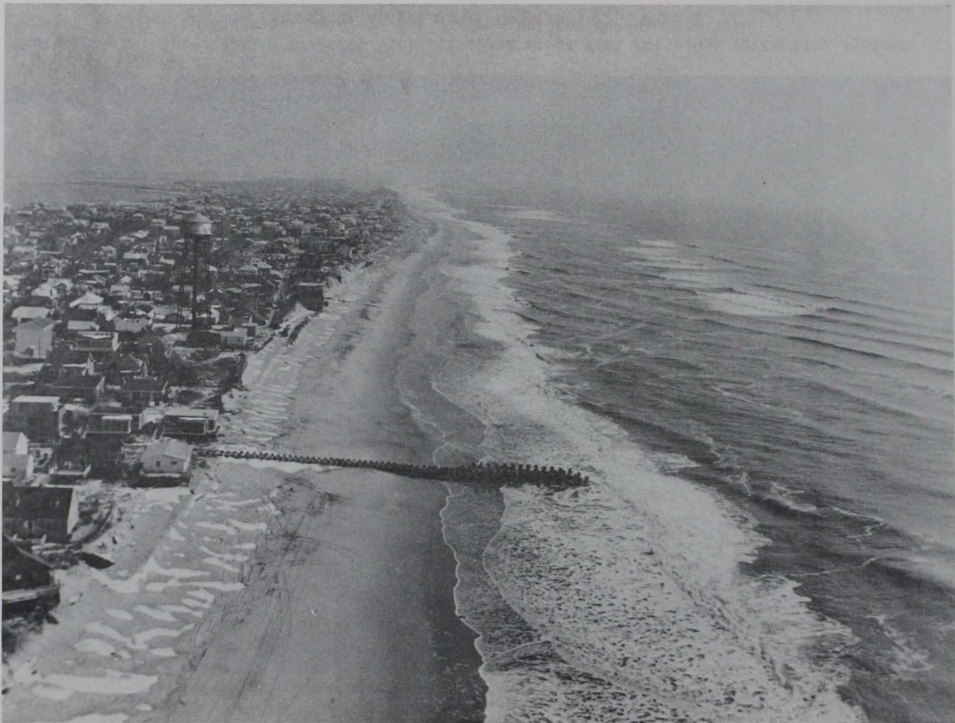
Photograph 2. Two- and five-ton STA-PODS used to stabilize the beach at Fire Island, New York (From Marine Modules, Inc.)
