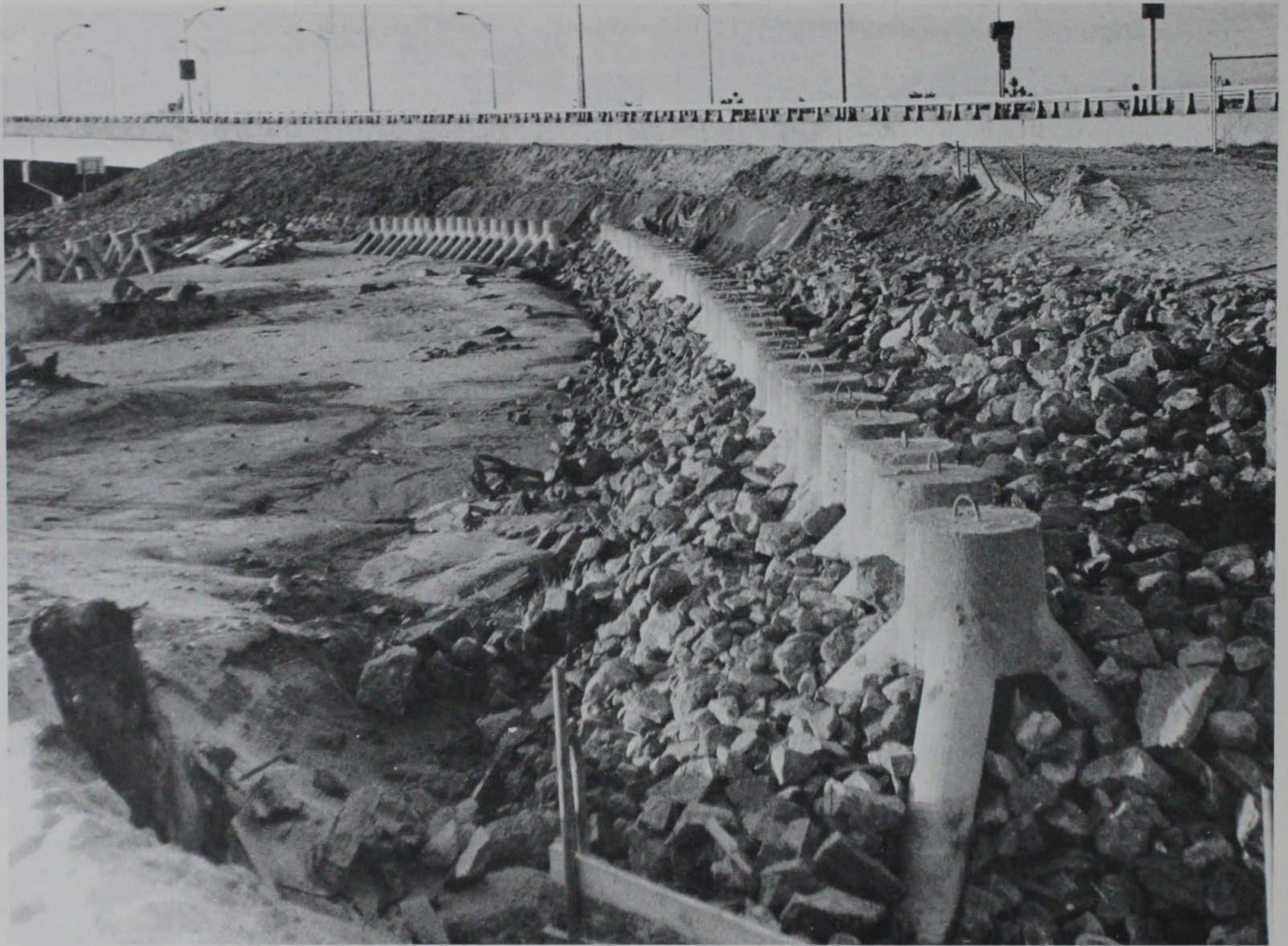
Photograph 1. Interlocking STA-PODS with entrapped stone fill for slope protection against high tides at the Cross Bay Parkway Bridge, Queens, New York
