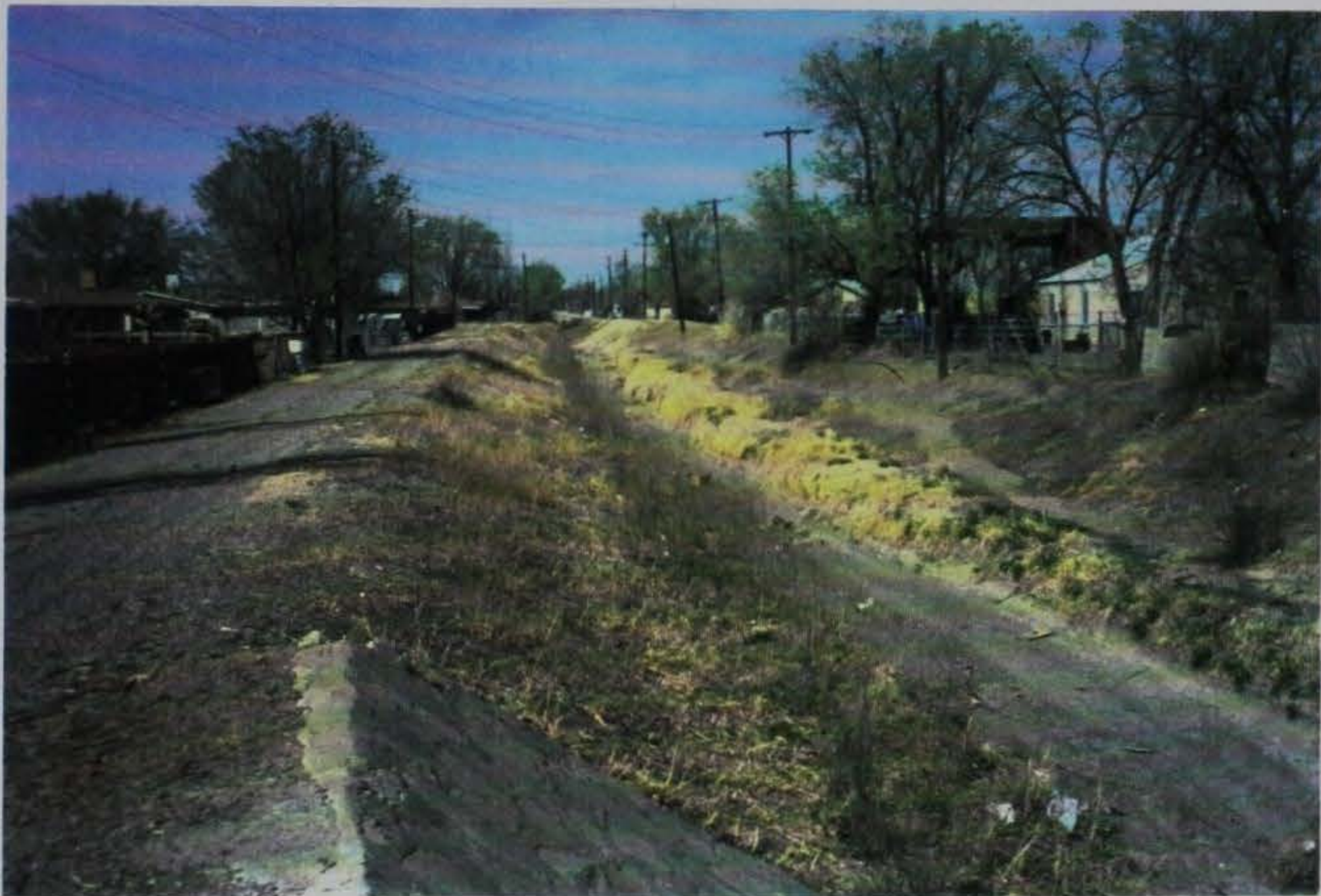
Figure 5. Rio Hondo channel in Roswell downstream of study reach (looking upstream)
