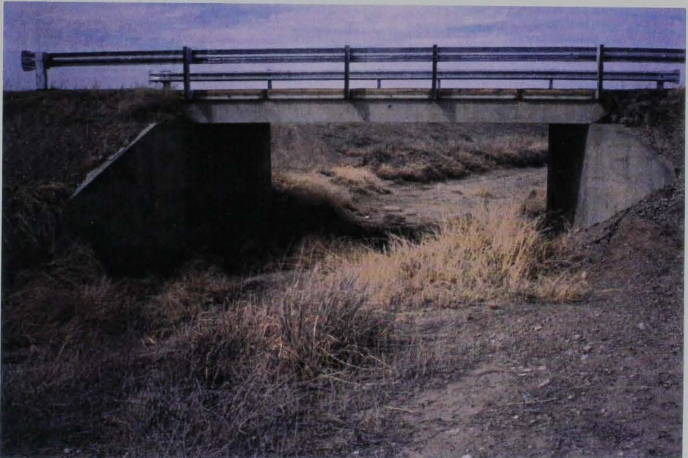
Figure 11. Rio Hondo channel at Brasher Road Bridge (looking downstream)
