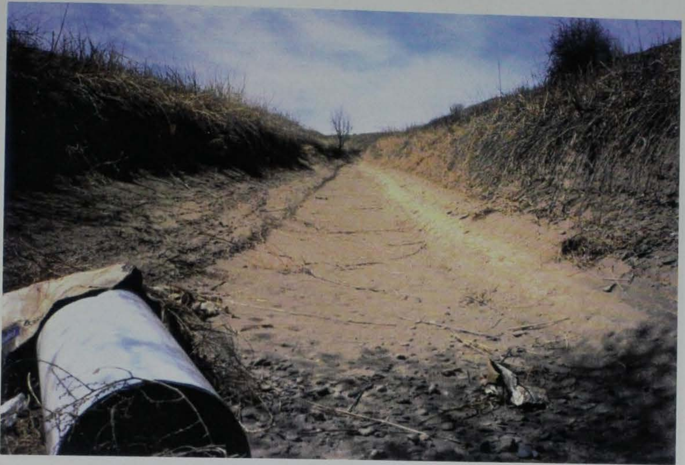
Figure 10. Rio Hondo channel in vicinity of detention basin reach (looking upstream)
