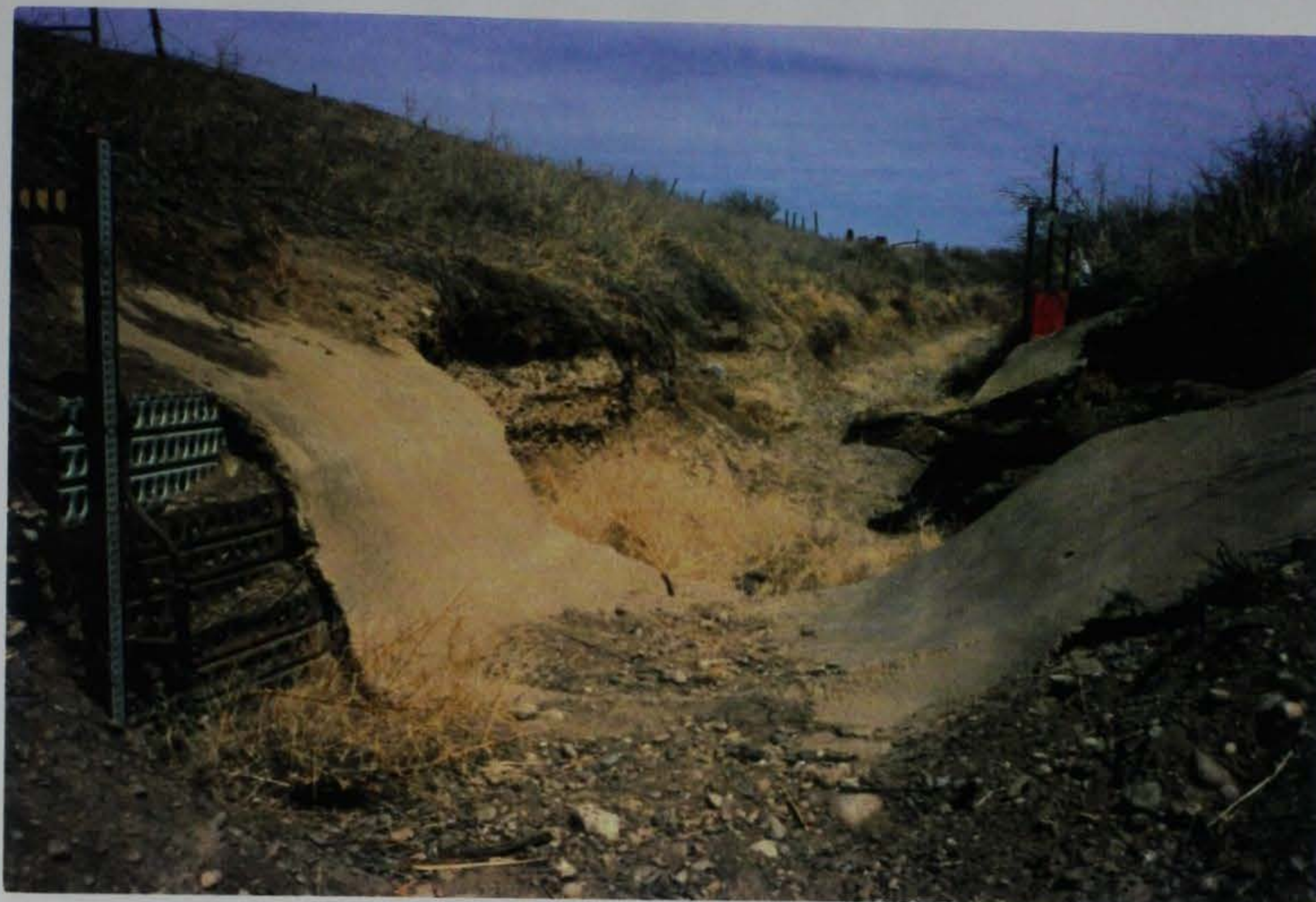
Figure 6. Rio Hondo channel at USGS gage 08393500 (looking downstream)
