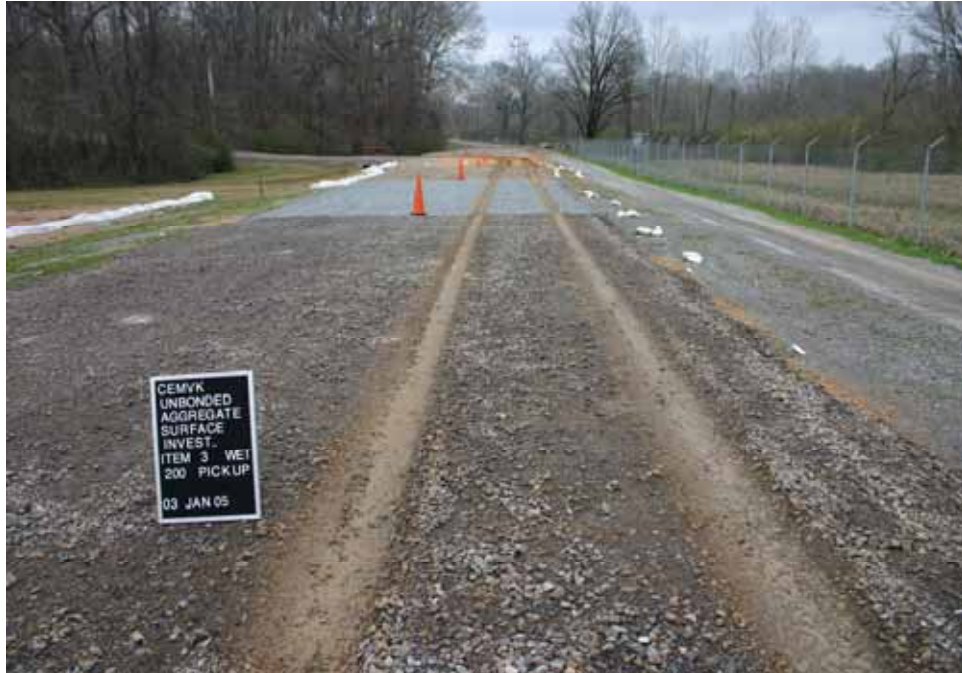
Photo C35. Item 3 (SST), wet lane, maintenance test section, 200 passes with pickup truck
