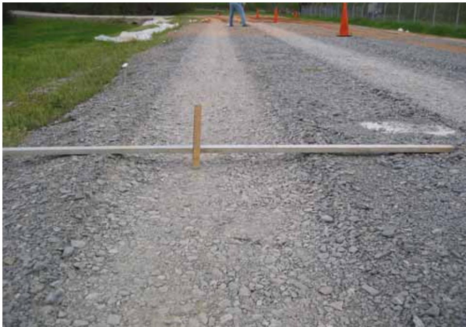
Photo C28. Item 4 (IGN), dry lane, maintenance test section, 200 passes with emulsion truck
