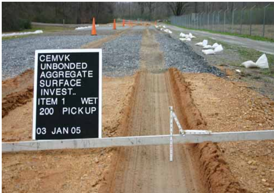
Photo C32. Item 1 (SCG), wet lane, maintenance test section, 200 passes with pickup truck
