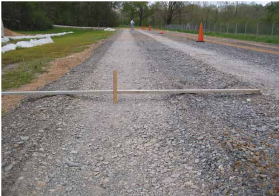
Photo C24. Item 2 (LST), dry lane, maintenance test section, 200 passes with emulsion truck
