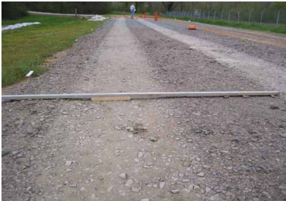
Photo C26. Item 3 (SST), dry lane, maintenance test section, 200 passes with emulsion truck
