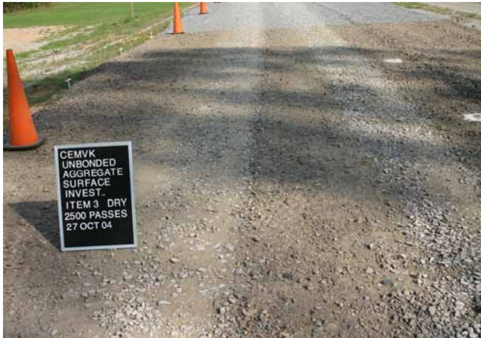
Photo C15. Item 3 (SST), dry lane, maintenance test section, 2500 passes with pickup truck
