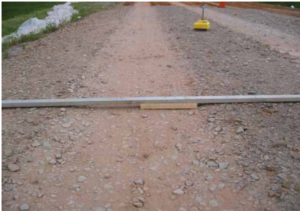
Photo C30. Item 5 (SSB), dry lane, maintenance test section, 200 passes with emulsion truck
