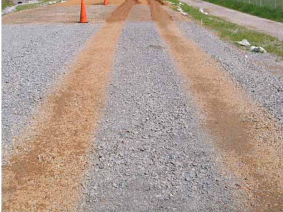
Photo C67. Item 4 (IGN), wet lane, maintenance test section, 50 passes with CBR truck
