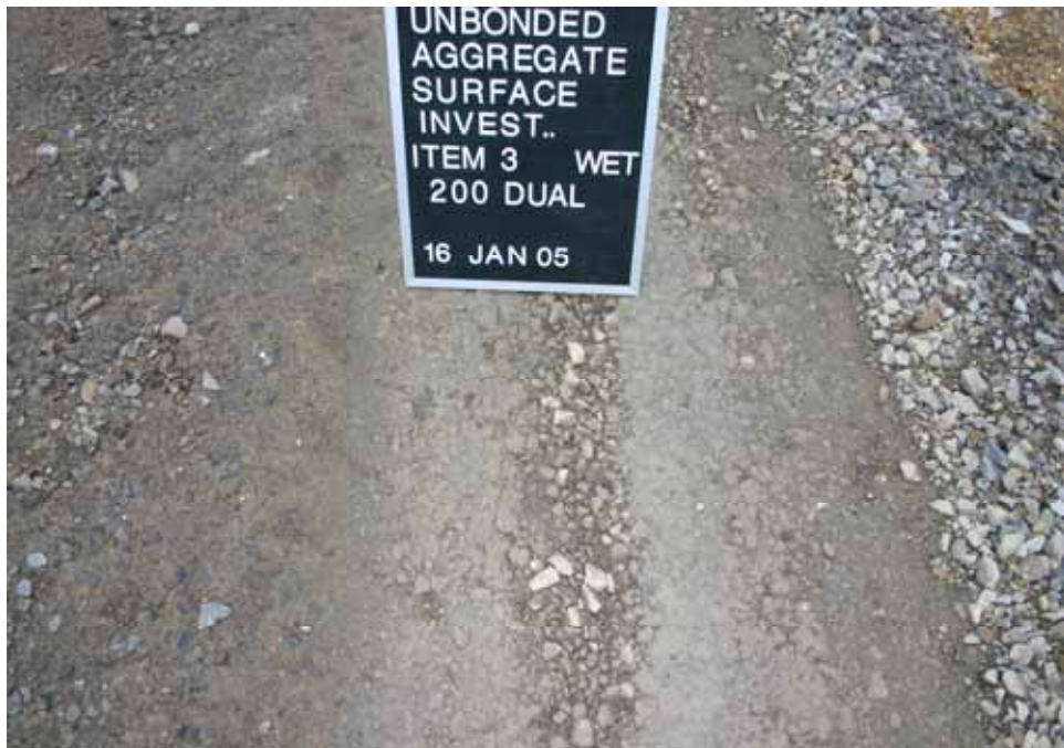
Photo C46. Item 3 (SST), wet lane, maintenance test section, 200 passes with dump truck
