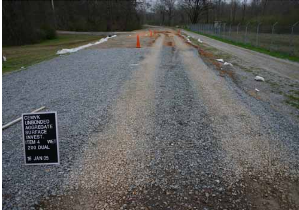
Photo C47. Item 4 (IGN), wet lane, maintenance test section, 200 passes with dump truck
