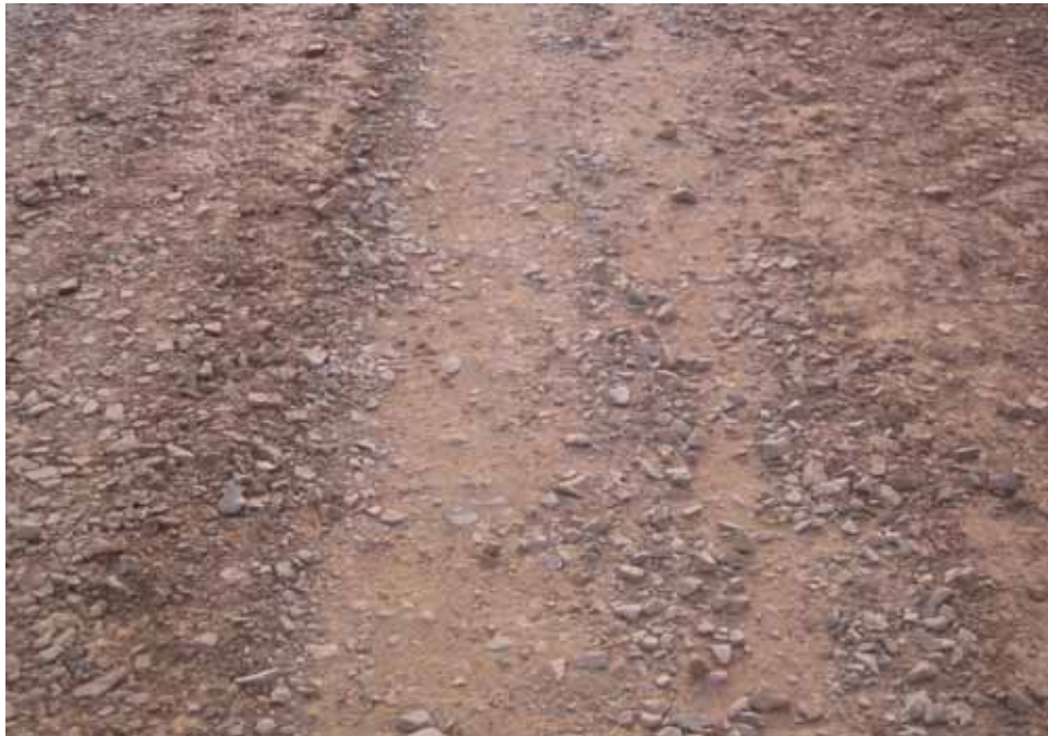
Photo C10. Item 5 (SSB), dry lane, maintenance test section, 500 passes with pickup truck
