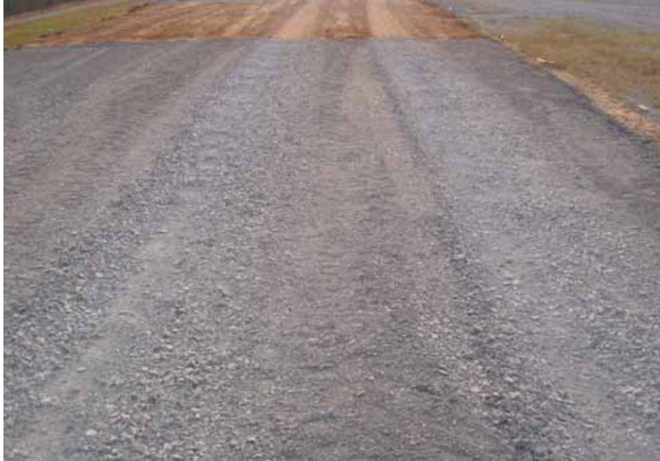
Photo C3. Item 2 (LST), dry lane, maintenance test section, 500 passes with pickup truck
