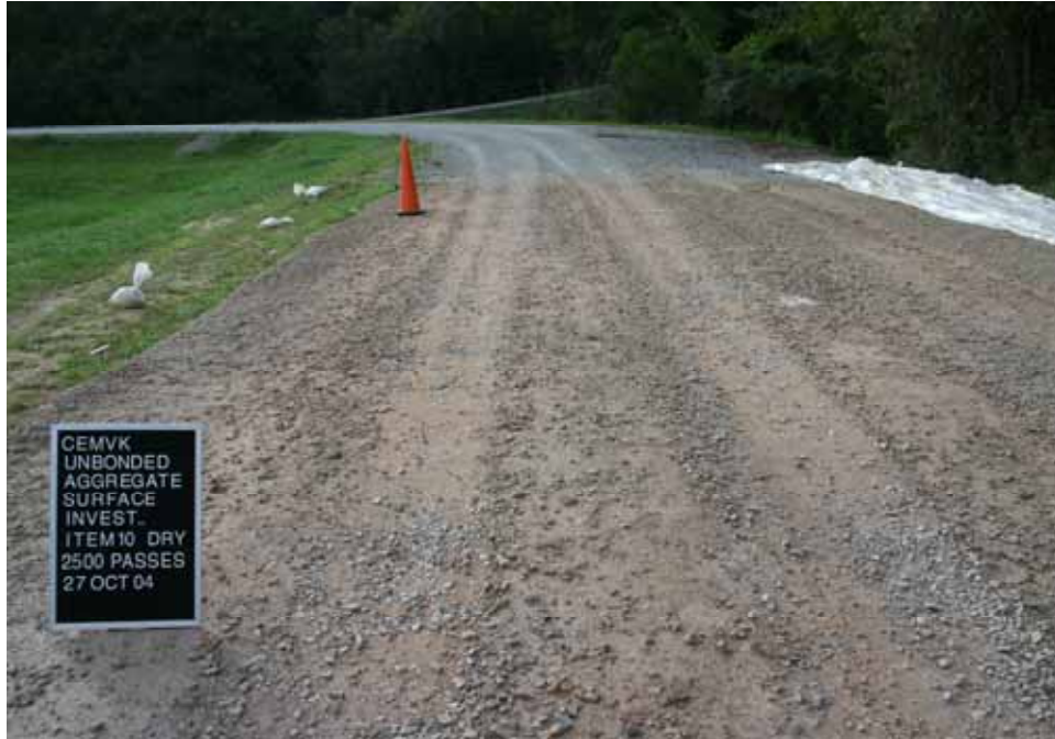
Photo C89. Item 10 (SSB), dry lane, new construction test section, 2500 passes with pickup truck
