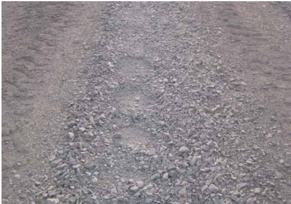
Photo C4. Item 2 (LST), dry lane, maintenance test section, 500 passes with pickup truck
