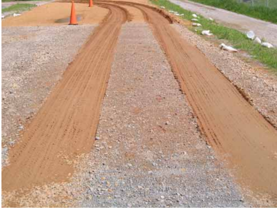
Photo C69. Item 5 (SSB), wet lane, maintenance test section, 50 passes with CBR truck
