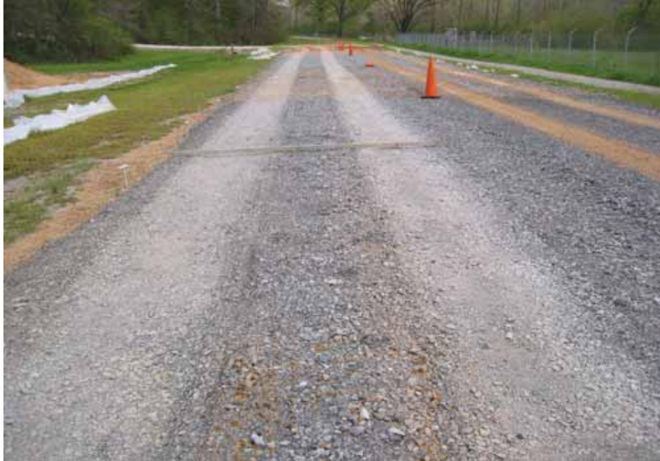
Photo C23. Item 2 (LST), dry lane, maintenance test section, 200 passes with emulsion truck
