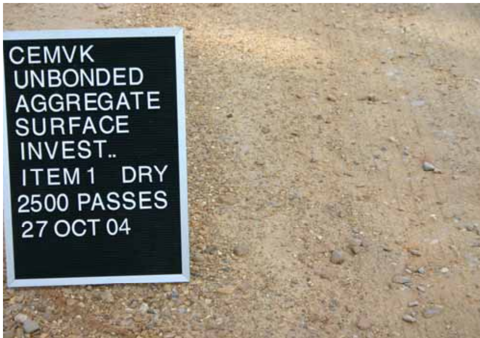
Photo C12. Item 1 (SCG), dry lane, maintenance test section, 2500 passes with pickup truck
