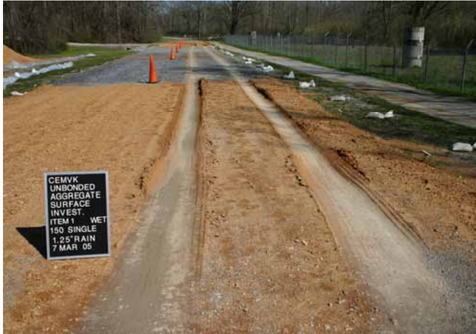
Photo C51. Item 1 (SCG), wet lane, maintenance test section, 150 passes with pickup truck
