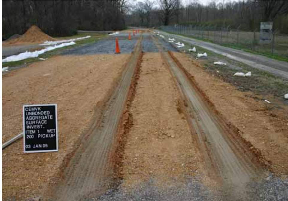
Photo C31. Item 1 (SCG), wet lane, maintenance test section, 200 passes with pickup truck
