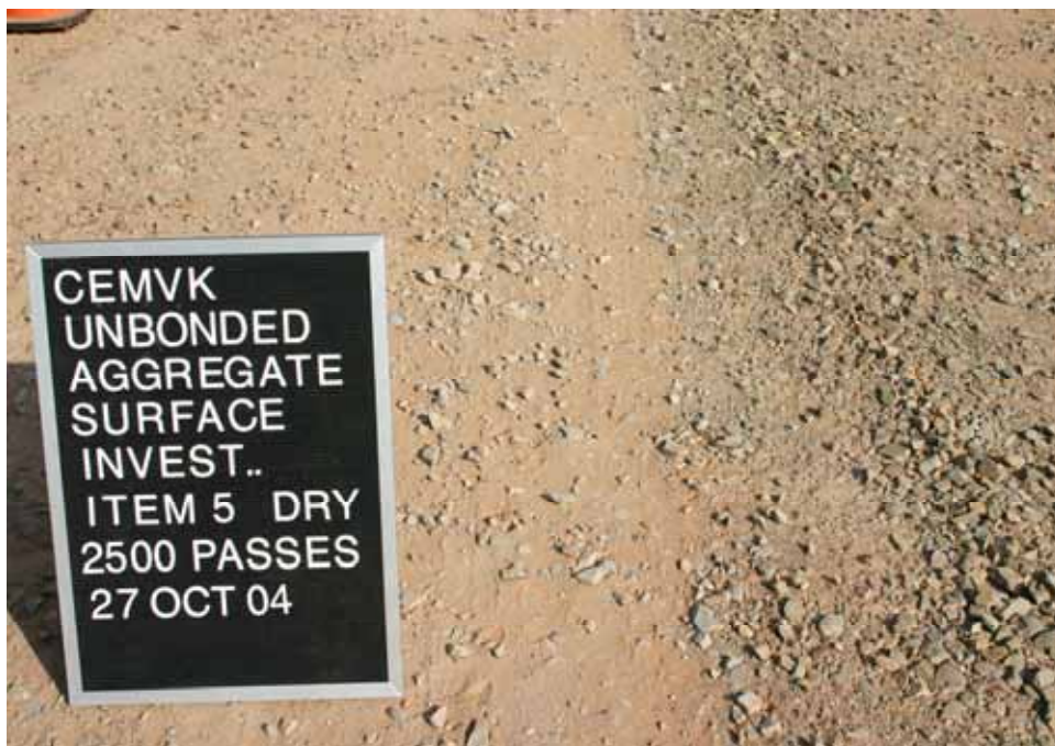
Photo C20. Item 5 (SSB), dry lane, maintenance test section, 2500 passes with pickup truck
