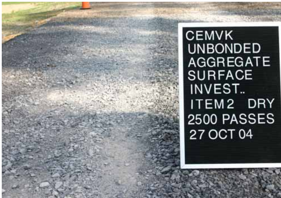
Photo C14. Item 2 (LST), dry lane, maintenance test section, 2500 passes with pickup truck
