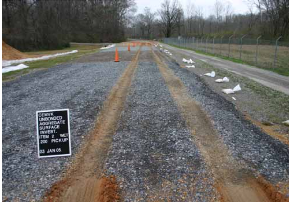
Photo C33. Item 2 (LST), wet lane, maintenance test section, 200 passes with pickup truck
