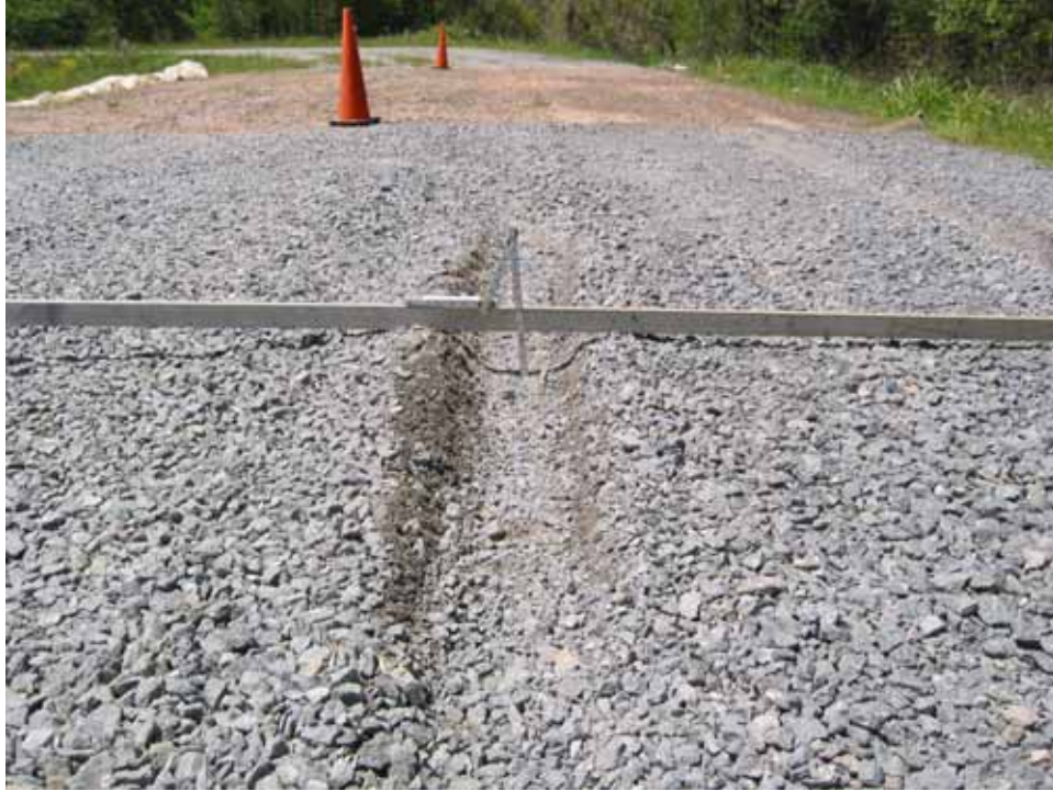
Photo C101. Item 9 (IGN), wet lane, new construction test section, 25 passes with pickup truck
