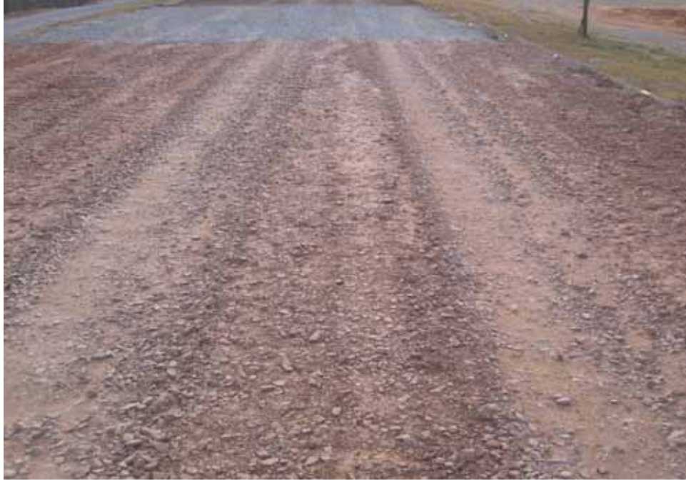
Photo C9. Item 5 (SSB), dry lane, maintenance test section, 500 passes with pickup truck
