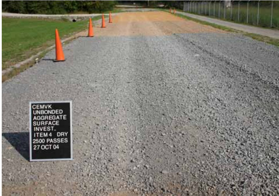
Photo C17. Item 4 (IGN), dry lane, maintenance test section, 2500 passes with pickup truck
