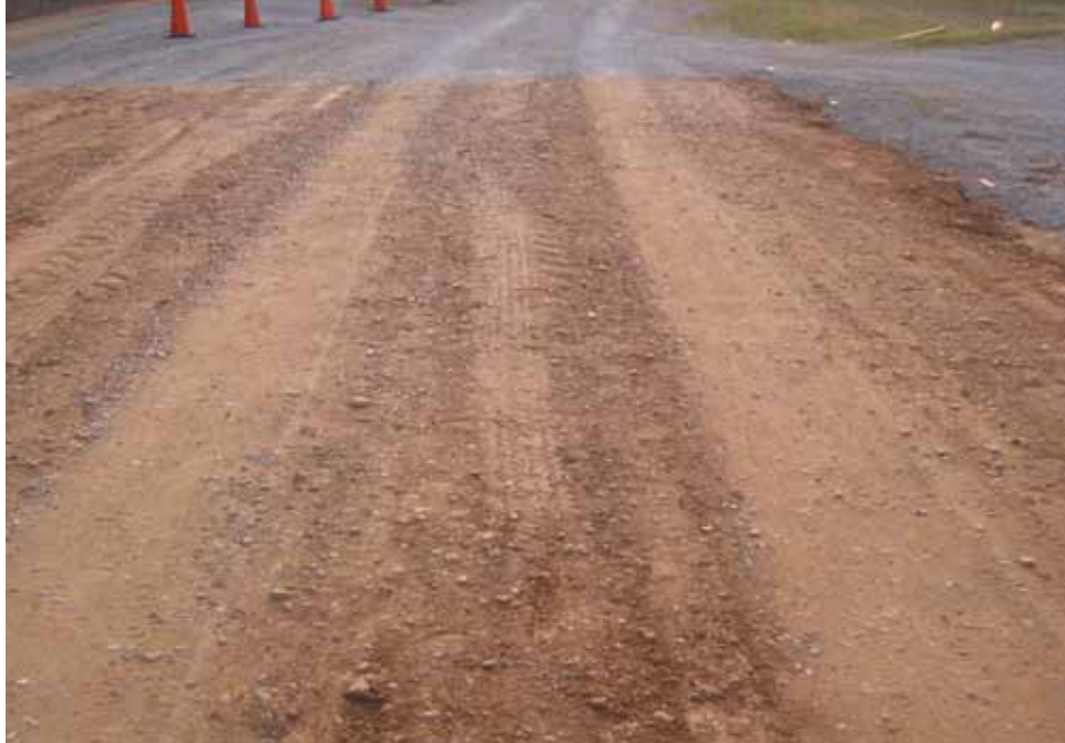
Photo C1. Item 1 (SCG), dry lane, maintenance test section, 500 passes with pickup truck
