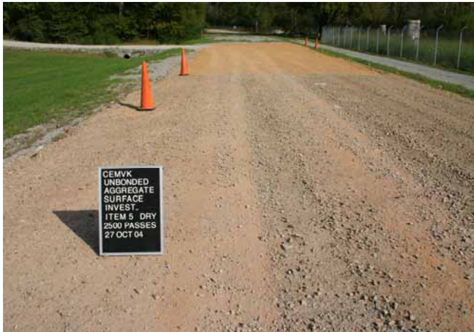
Photo C19. Item 5 (SSB), dry lane, maintenance test section, 2500 passes with pickup truck
