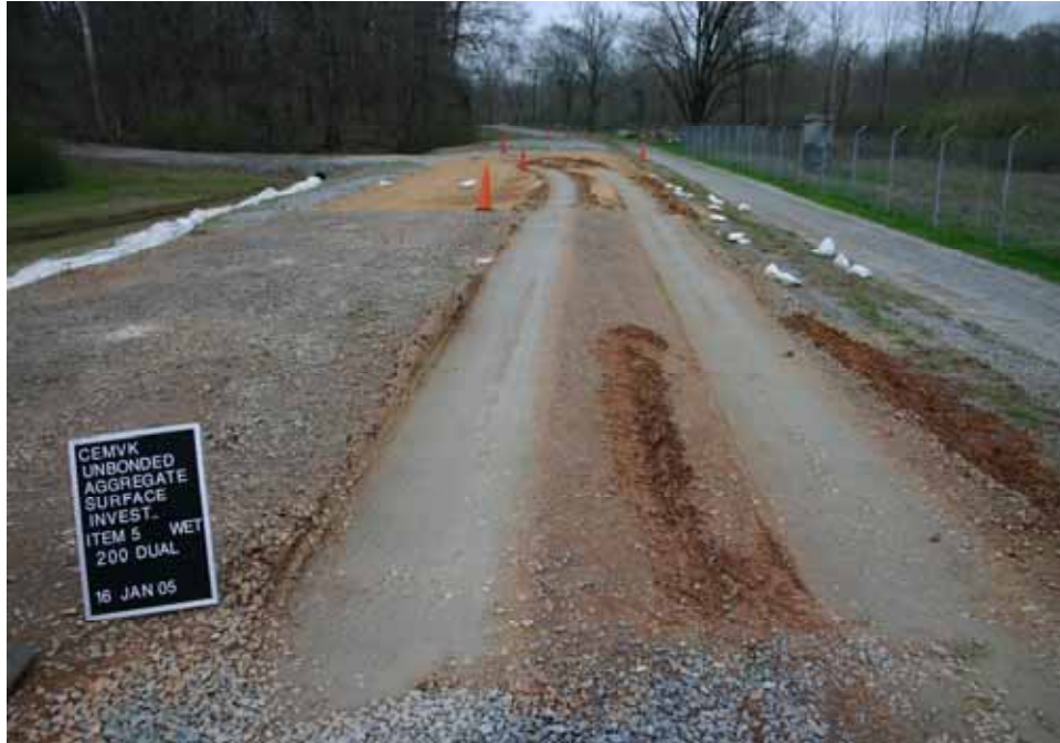
Photo C49. Item 5 (SSB), wet lane, maintenance test section, 200 passes with dump truck
