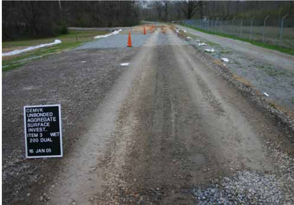
Photo C45. Item 3 (SST), wet lane, maintenance test section, 200 passes with dump truck
