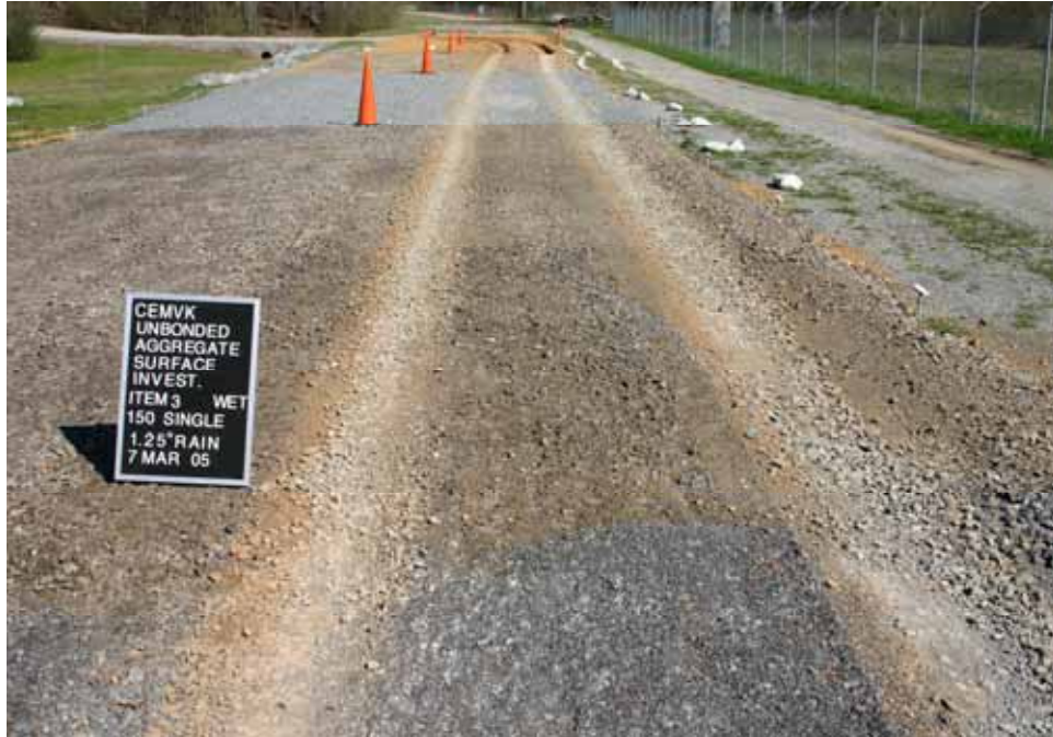
Photo C55. Item 3 (SST), wet lane, maintenance test section, 150 passes with pickup truck
