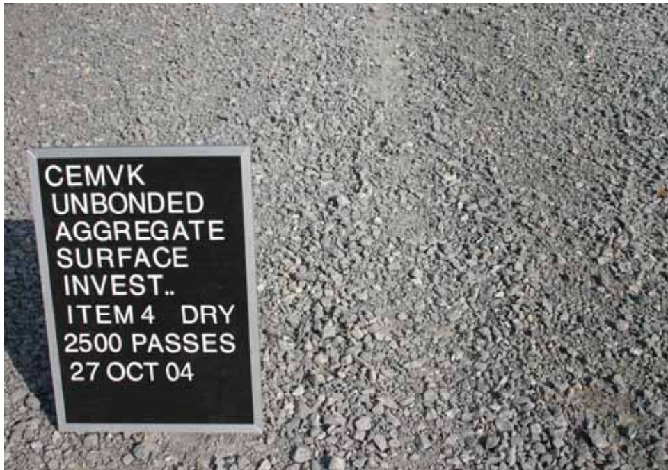
Photo C18. Item 4 (IGN), dry lane, maintenance test section, 2500 passes with pickup truck
