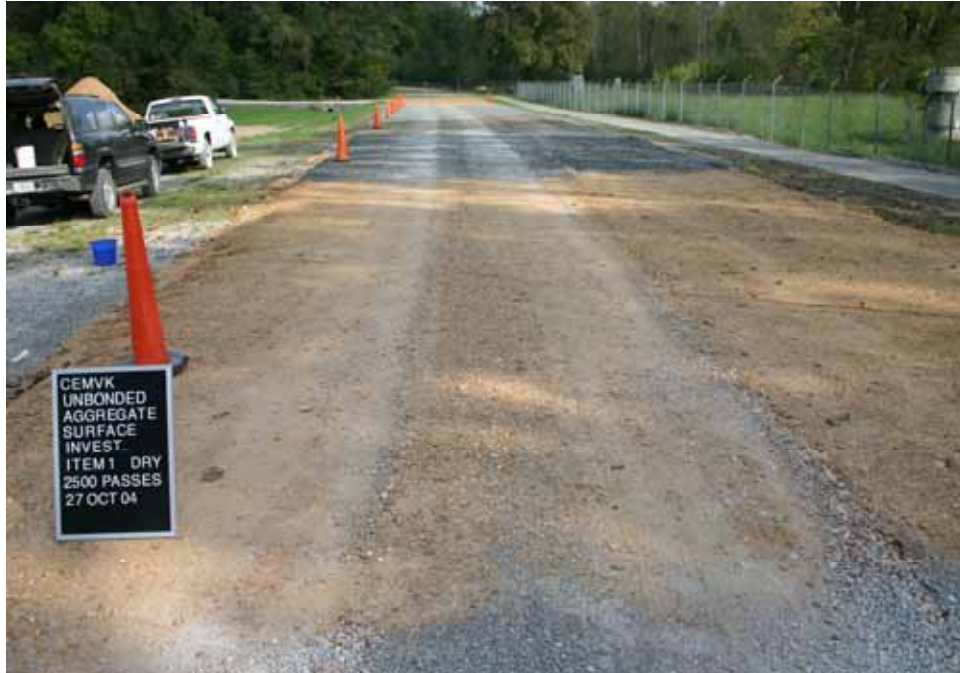
Photo C11. Item 1 (SCG), dry lane, maintenance test section, 2500 passes with pickup truck
