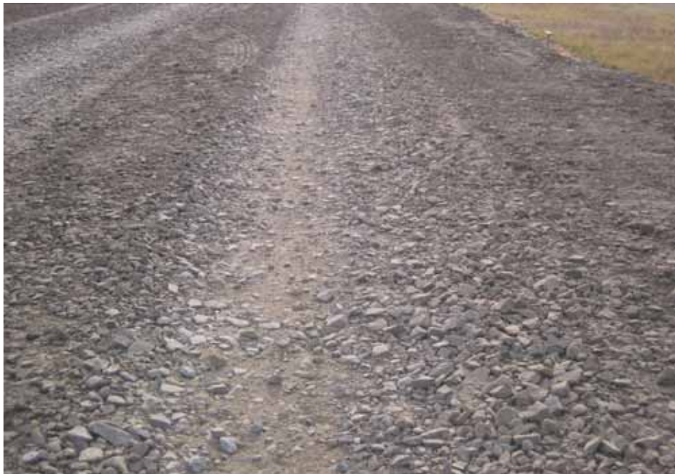
Photo C6. Item 3 (SST), dry lane, maintenance test section, 500 passes with pickup truck
