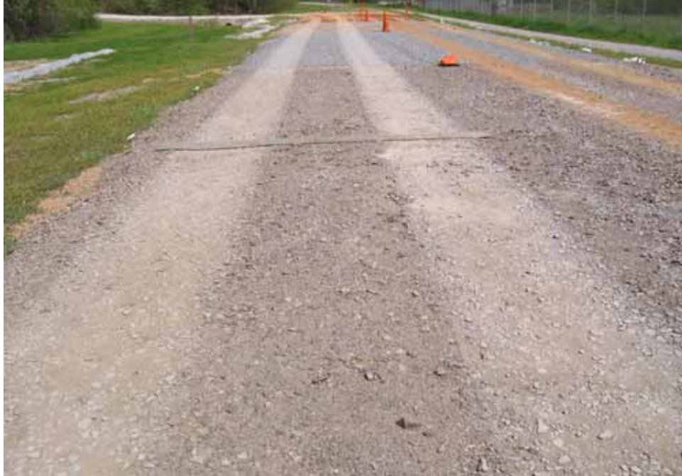
Photo C25. Item 3 (SST), dry lane, maintenance test section, 200 passes with emulsion truck
