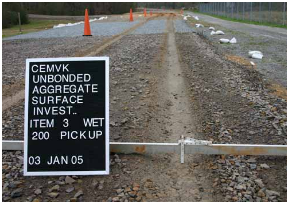
Photo C36. Item 3 (SST), wet lane, maintenance test section, 200 passes with pickup truck
