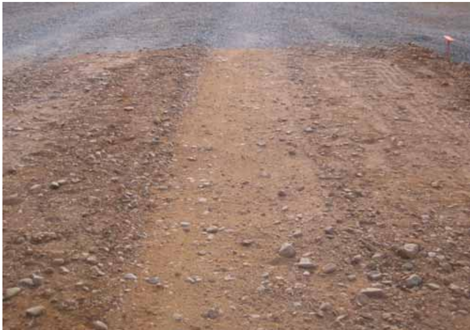
Photo C2. Item 1 (SCG), dry lane, maintenance test section, 500 passes with pickup truck
