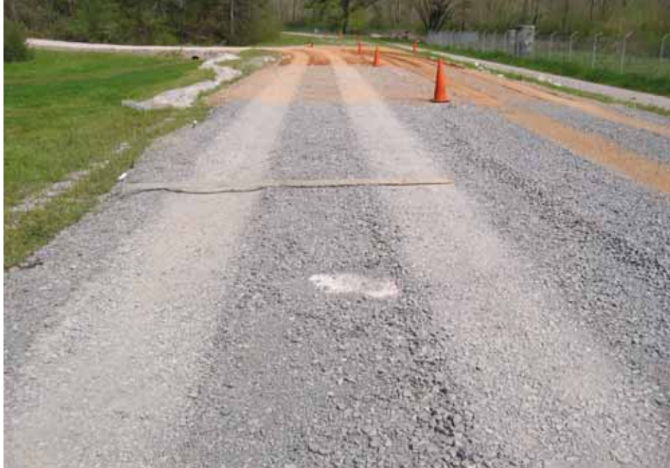
Photo C27. Item 4 (IGN), dry lane, maintenance test section, 200 passes with emulsion truck
