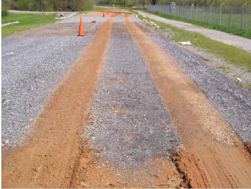
Photo C63. Item 2 (LST), wet lane, maintenance test section, 50 passes with CBR truck
