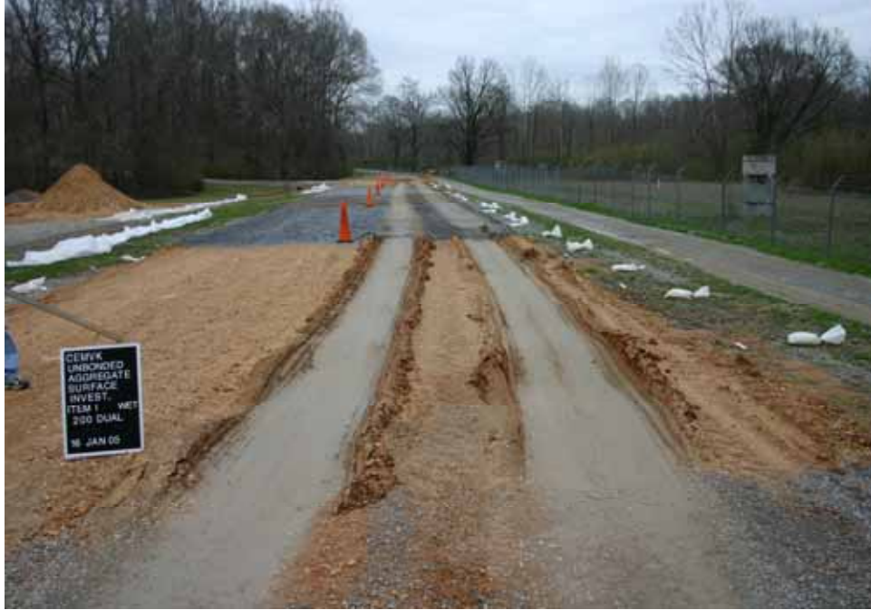
Photo C41. Item 1 (SCG), wet lane, maintenance test section, 200 passes with dump truck
