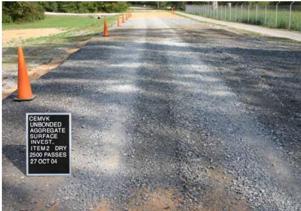
Photo C13. Item 2 (LST), dry lane, maintenance test section, 2500 passes with pickup truck
