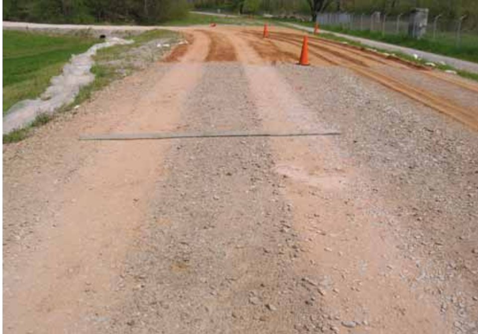
Photo C29. Item 5 (SSB), dry lane, maintenance test section, 200 passes with emulsion truck
