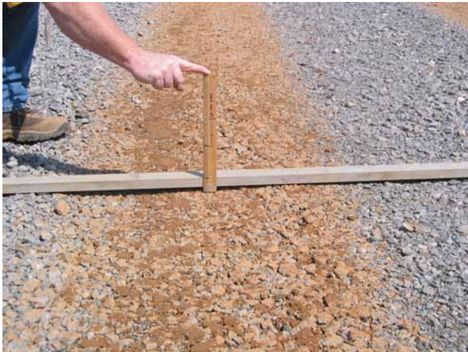
Photo C68. Item 4 (IGN), wet lane, maintenance test section, 50 passes with CBR truck
