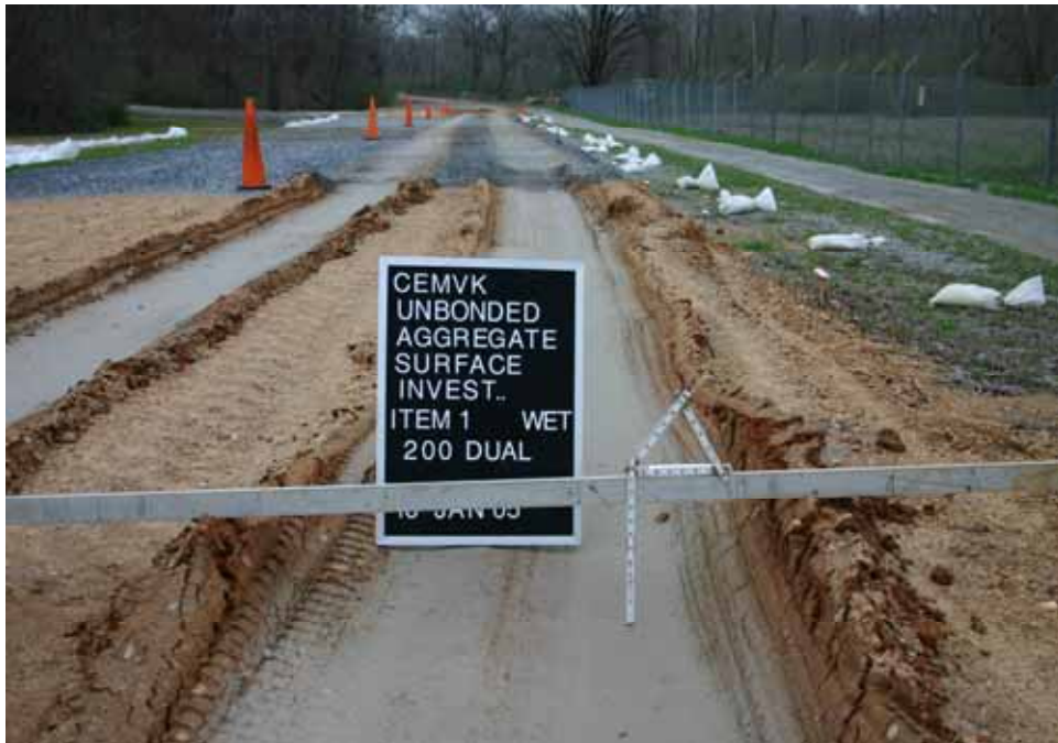
Photo C42. Item 1 (SCG), wet lane, maintenance test section, 200 passes with dump truck
