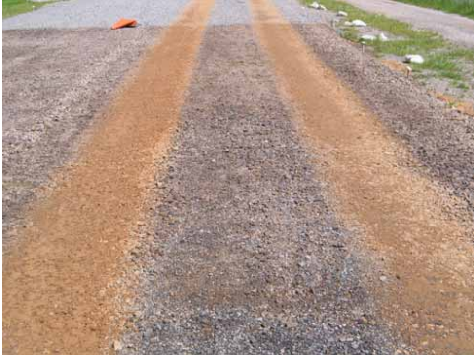
Photo C65. Item 3 (SST), wet lane, maintenance test section, 50 passes with CBR truck
