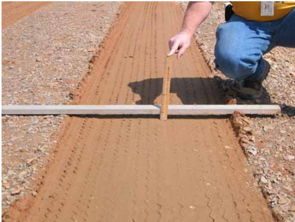
Photo C70. Item 5 (SSB), wet lane, maintenance test section, 50 passes with CBR truck
