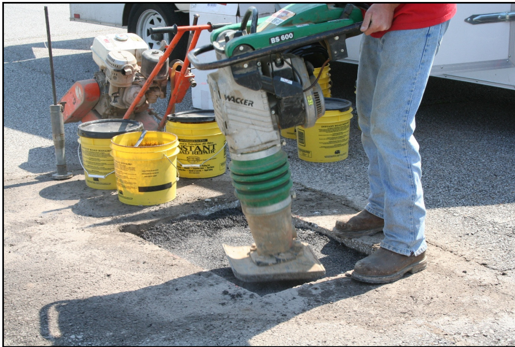
Figure 7. Patching the hole of the removed aged AC sample.
