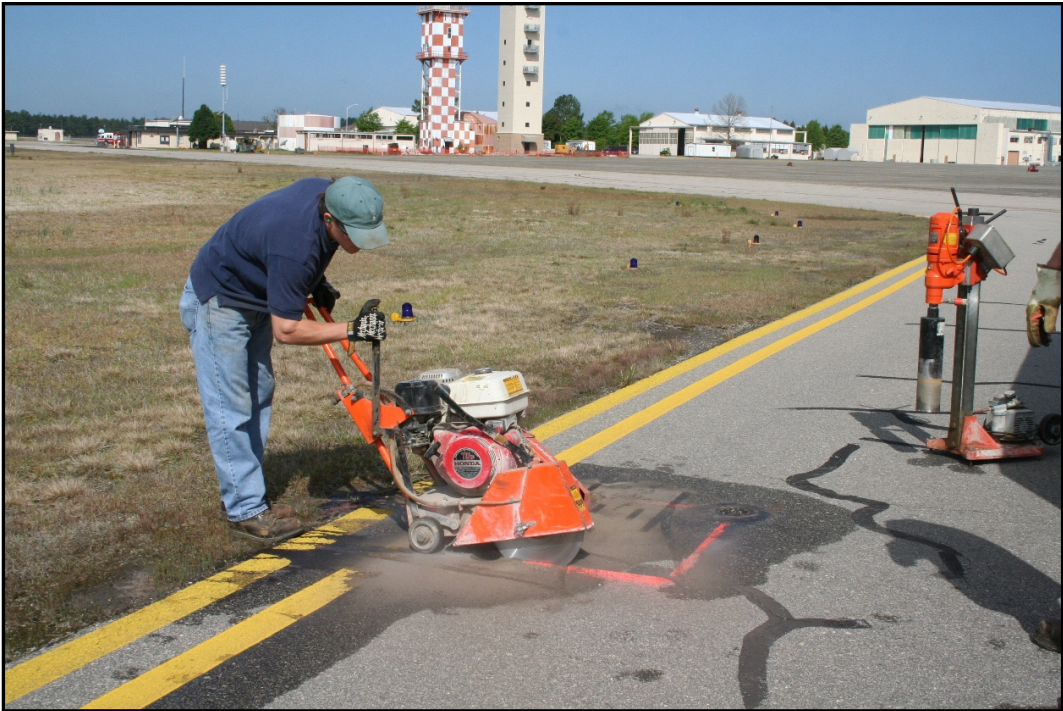
Figure 5. Sawing the aged AC sample.
