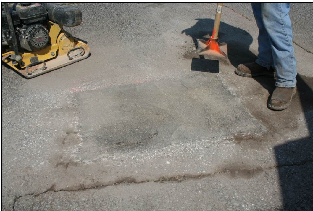
Figure 8. Patched AC sample.
