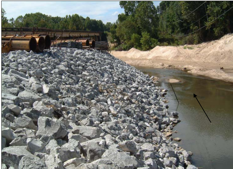
Figure 93. Newly installed riprap on the left bank of the Comite River at the Louisiana Hwy 67 crossing near Olive Branch, LA (downstream view—July 2004) (arrow notes flow direction).
