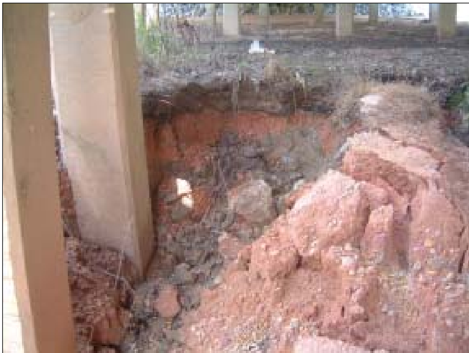
Figure 15. Scour of bridge piers at the Hwy 24 crossing of the East Fork near Peoria, MS (July 2003).
