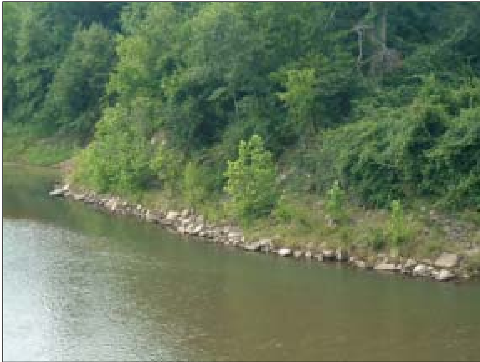
Figure 43. Riprap on the left bank of the Amite River at the Louisiana Hwy 37 crossing near Grangeville, LA (September 2003).
