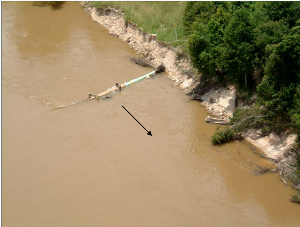
Figure 61. Exposed pipeline and steep, eroding right bank of the Amite River near Magnolia, LA (arrow notes flow direction—July 2004).
