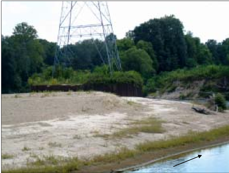
Figure 31. Power transmission pylon at the Louisiana Hwy 432 crossing of the Amite River near Felixville, LA (view downstream—September 2003) (arrow notes flow direction). Note the terrace effect on the point bar.
