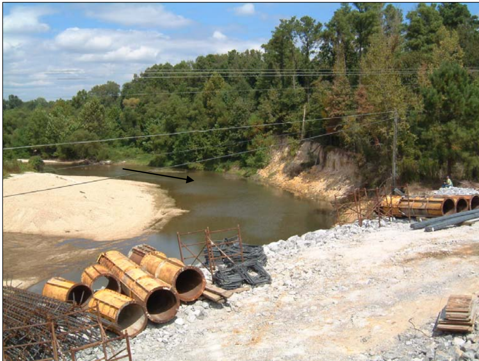
Figure 91. Upstream view of the Comite River at the Louisiana Hwy 67 crossing near Olive Branch, LA (note steep, eroding left bank—July 2004) (arrow notes flow direction).
