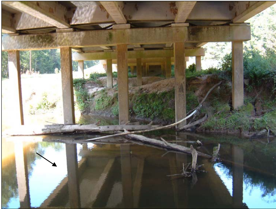
Figure 51. Steep, eroded left bank of Darling Creek at the Louisiana Hwy 10 crossing near Darlington, LA (arrow notes flow direction—September 2003).
