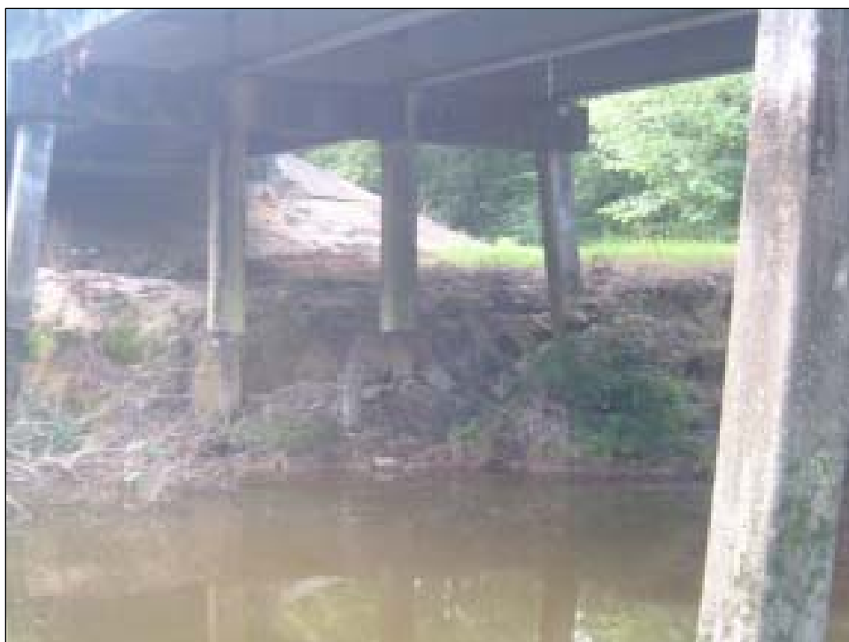
Figure 7. Scour of bridge piers at the Hwy 98 crossing of the East Fork near Smithdale, MS (July 2003).
