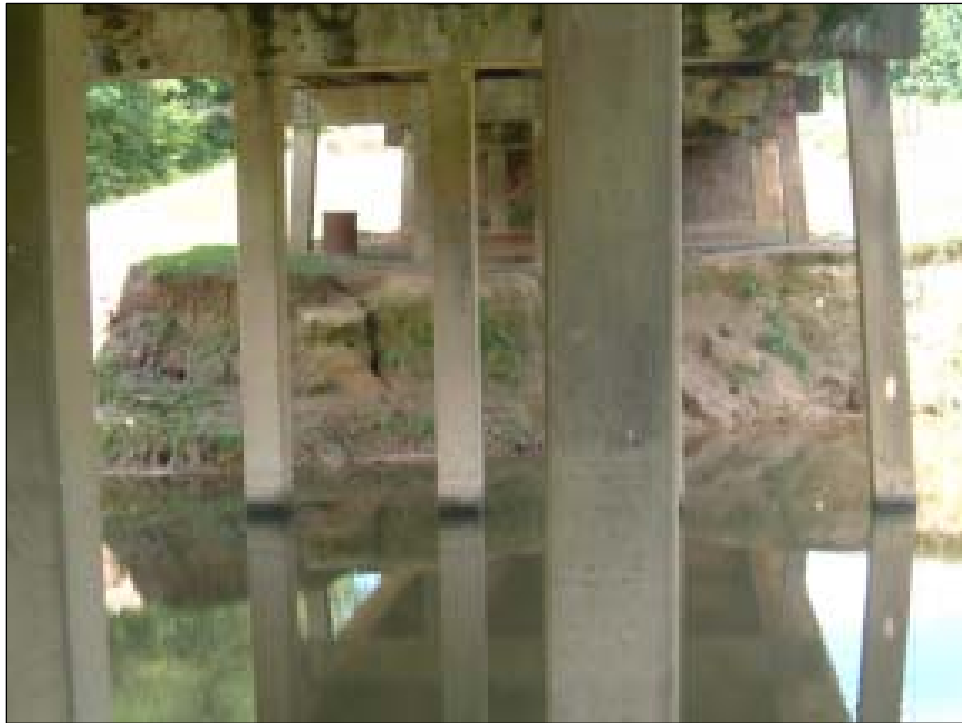
Figure 10. Steep, eroded bank of the East Fork at the Hwy 570 crossing near Mars Hill, MS (July 2003).
