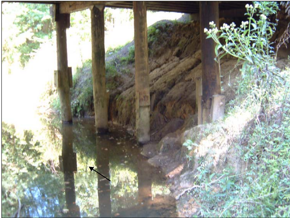
Figure 55. Bridge pier scour at the Louisiana Hwy 38 crossing of Darling Creek near Darlington, LA (arrow notes flow direction—September 2003).
