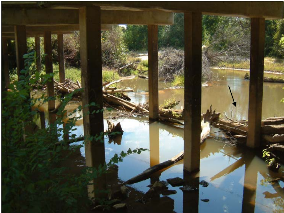
Figure 46. Debris jam on Beaver Creek at the Perkins Road crossing near the Mississippi/Louisiana state line (view upstream—September 2003) (arrow notes flow direction).
