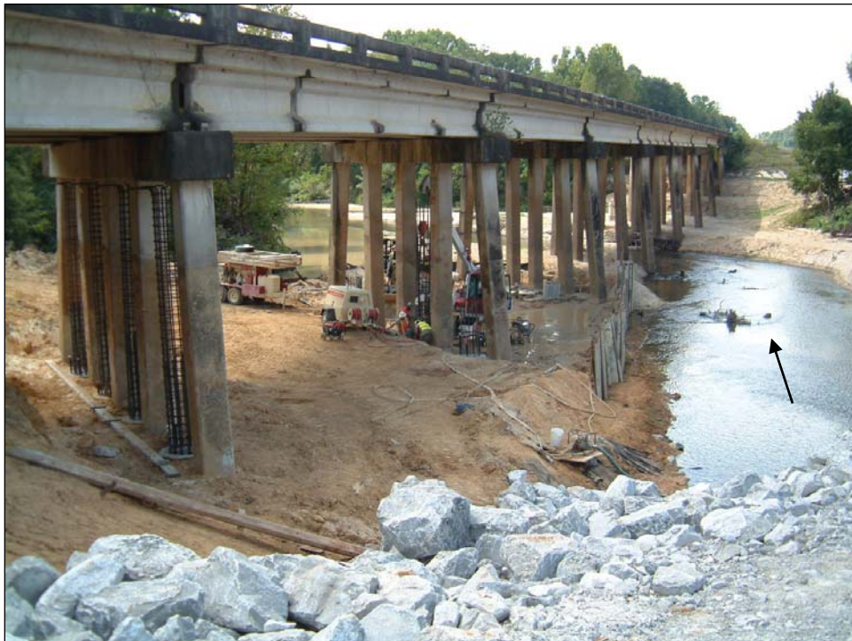
Figure 94. Bridge pier repair at the Louisiana Hwy 67 crossing of the Comite River near Olive Branch, LA (downstream view—July 2004) (arrow notes flow direction).
