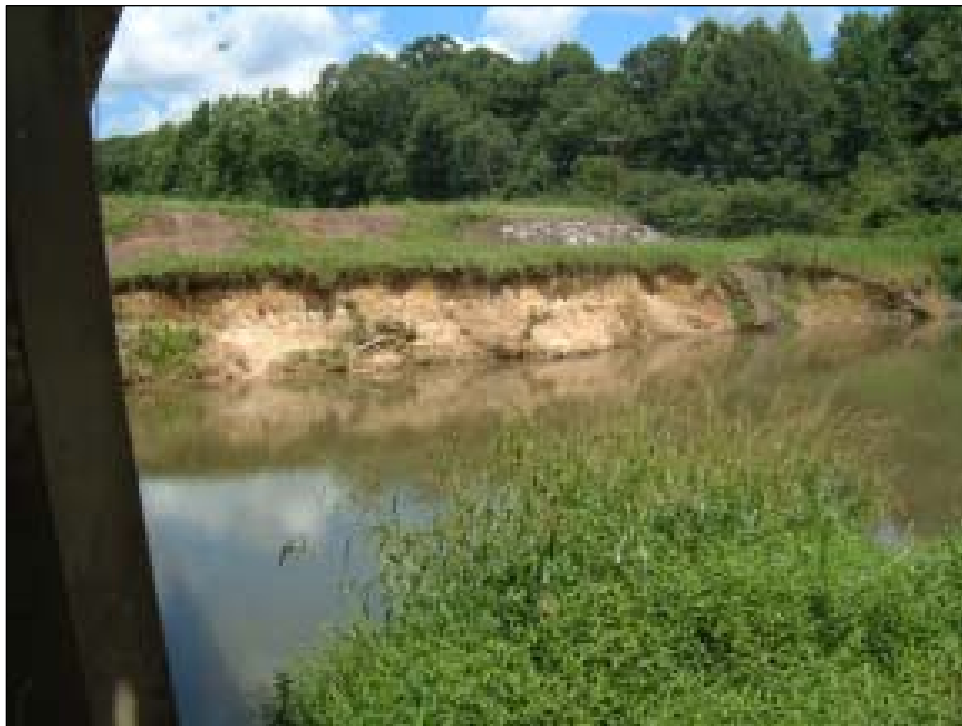
Figure 11. Steep, eroded right bank of the East Fork at the Hwy 570 crossing near Mars Hill, MS (July 2003).
