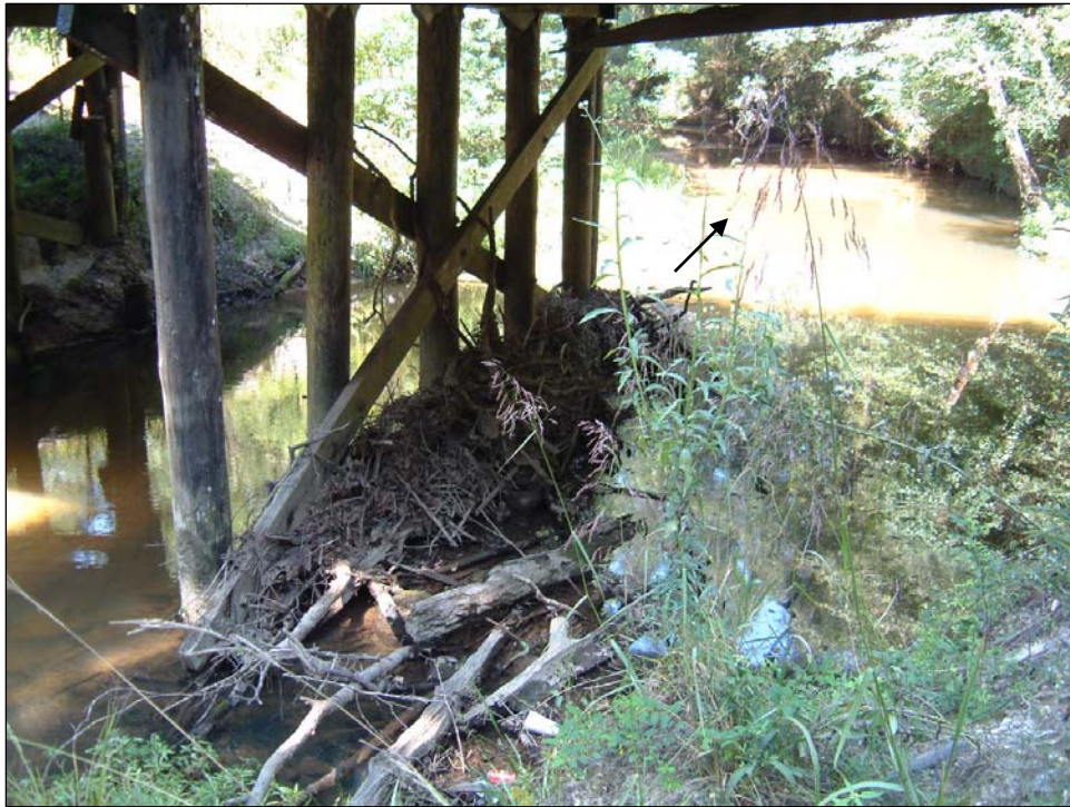
Figure 57. Debris jam at the Louisiana Hwy 38 crossing of Darling Creek near Darlington, LA (arrow notes flow direction—September 2003).
