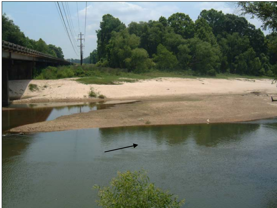
Figure 77. Eroding sand and gravel bar at the Louisiana Hwy 64 crossing of the Amite River near Magnolia, LA (arrow notes flow direction—June 2003).
