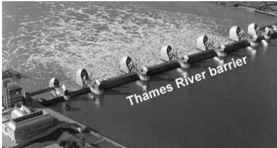
Figure 2. Thames River flood barrier gates (after Gilbert and Horner 1984)
