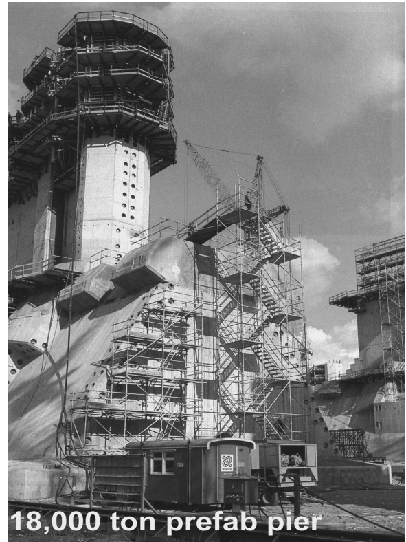
b. Storm surge barrier float-in pier detail
