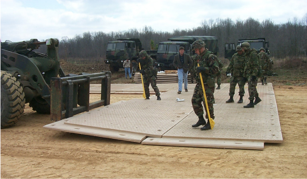
Photo 9. Bar tools used to align connector pinholes during placement
