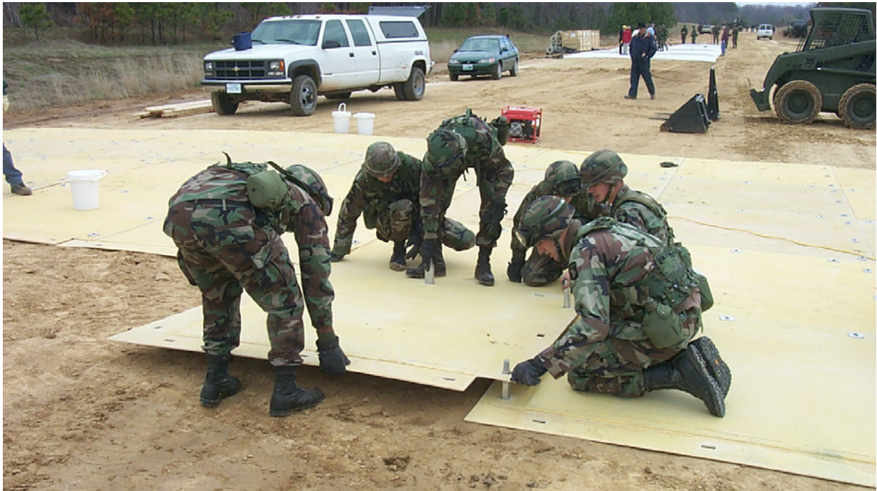
Photo 16. Hand placement and alignment of MP Mat panels
