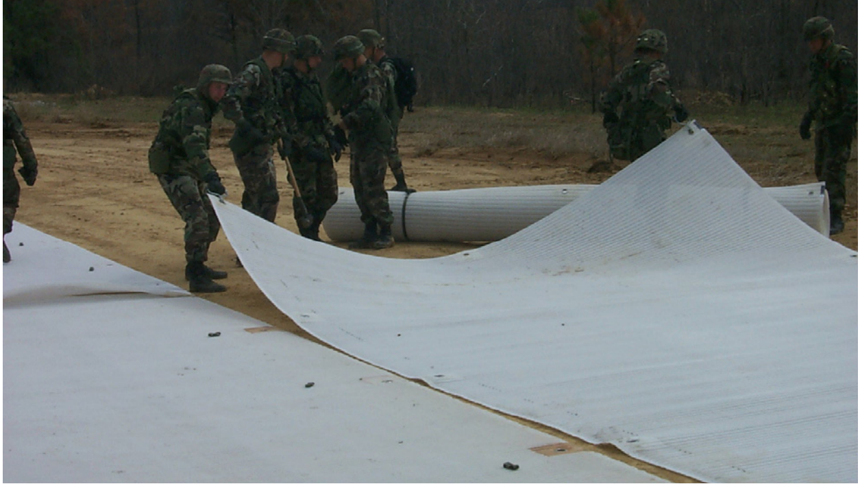
Photo 5. Stretching out Mobi-Mat panel before anchoring
