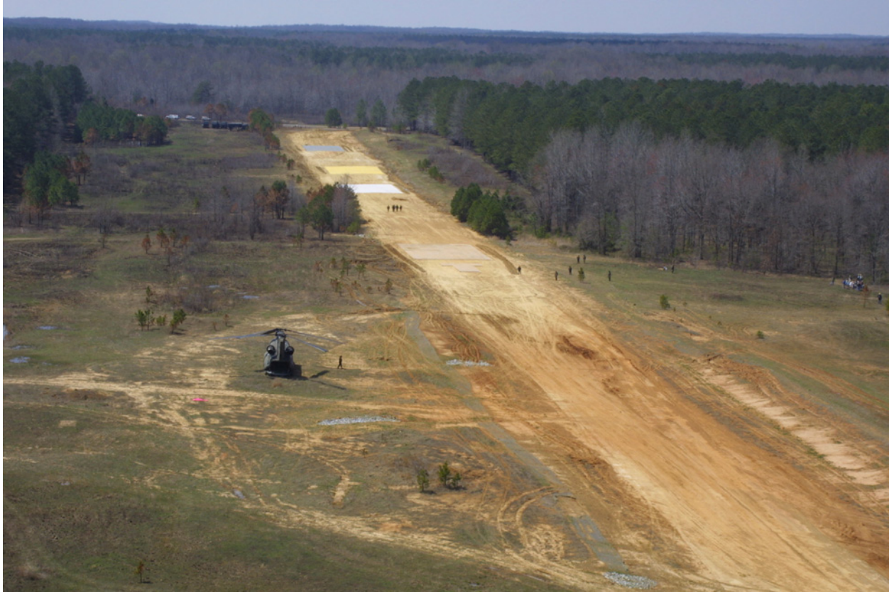
Photo 20. Aerial view of contingency helipad matting test sections at Aardvark LZ
