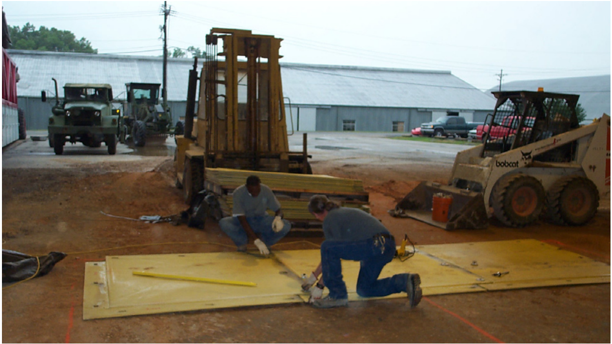
Photo 27. Installing 5-ply MP matting system
