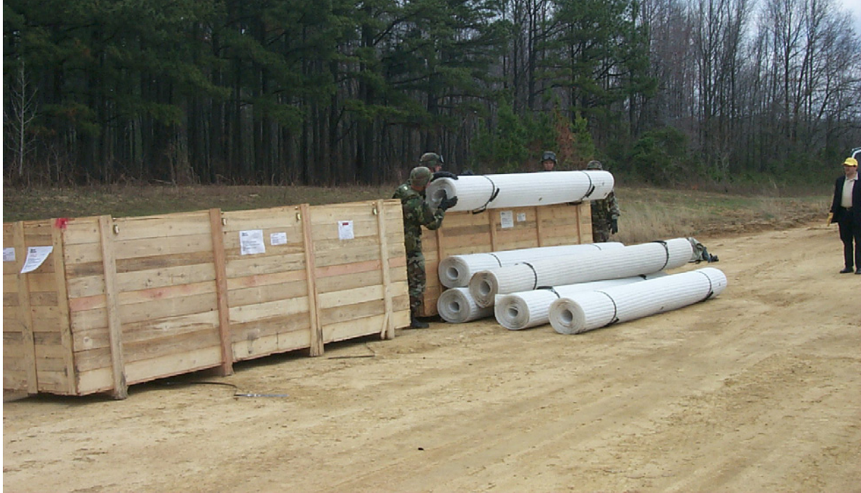
Photo 3. Unloading rolls of Mobi-Mat from shipping crates
