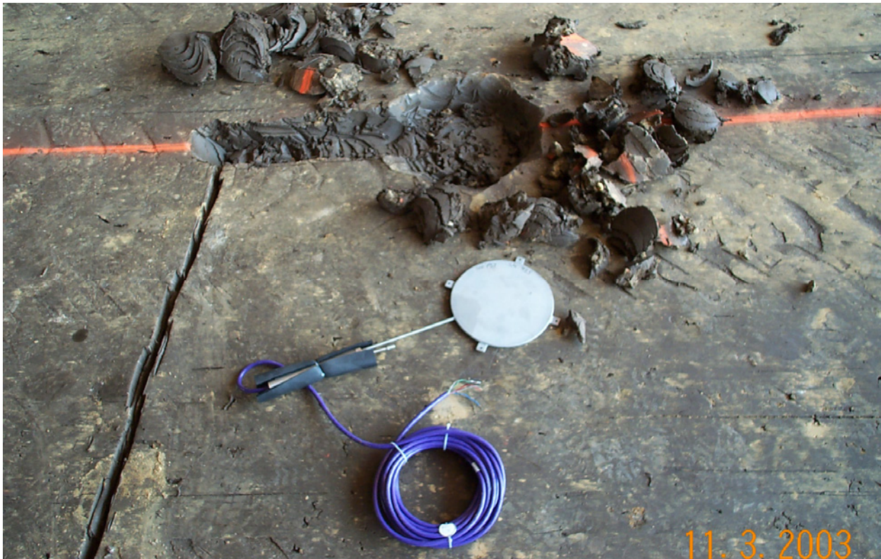
Photo 33. 100-psi GeoKon Pressure Cell awaits placement in CH clay
