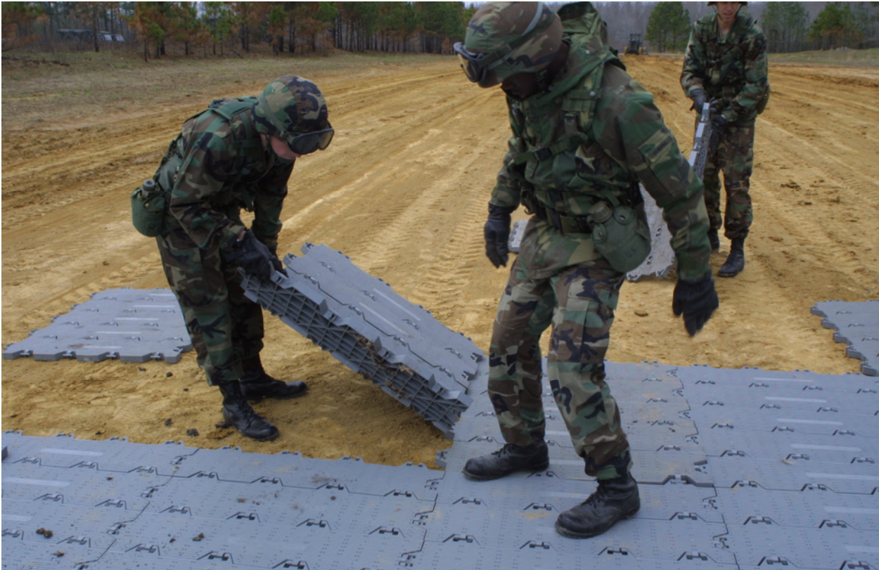
Photo 12. Snapping panels of SUPA-TRAC into place with boot heel
