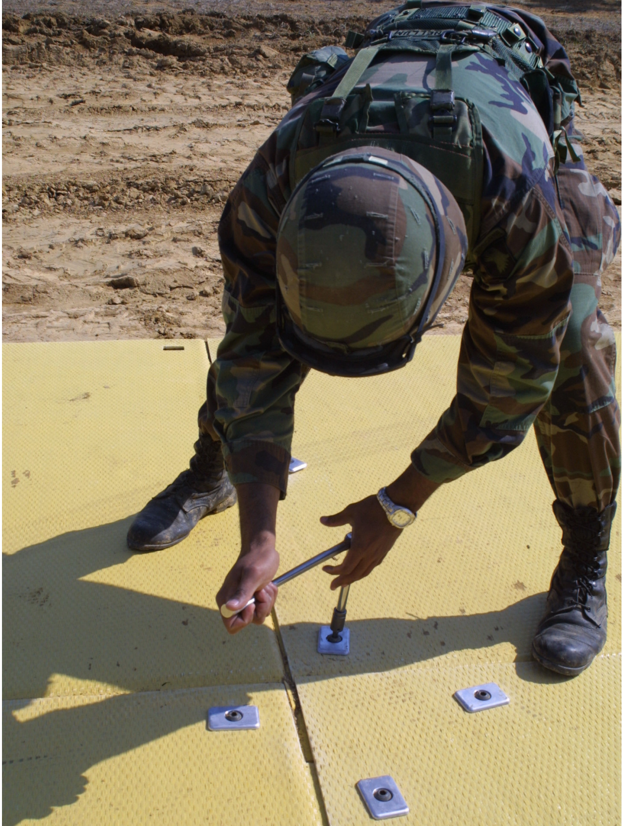
Photo 18. Locking MP Mat connector pins with socket wrench
