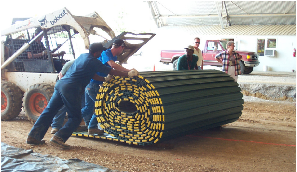
Photo 29. Installing Rolla-Road matting system
