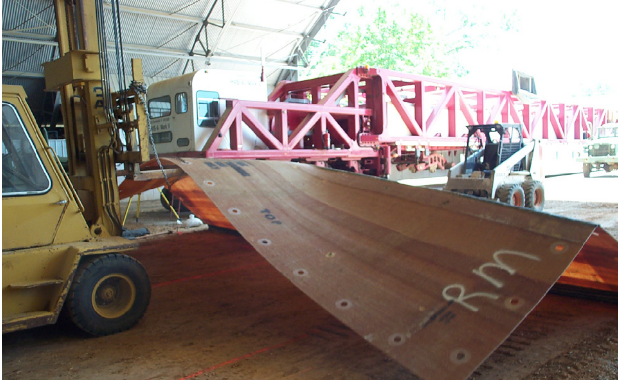
Photo 28. Installing Rapid Mat (FFM) matting system
