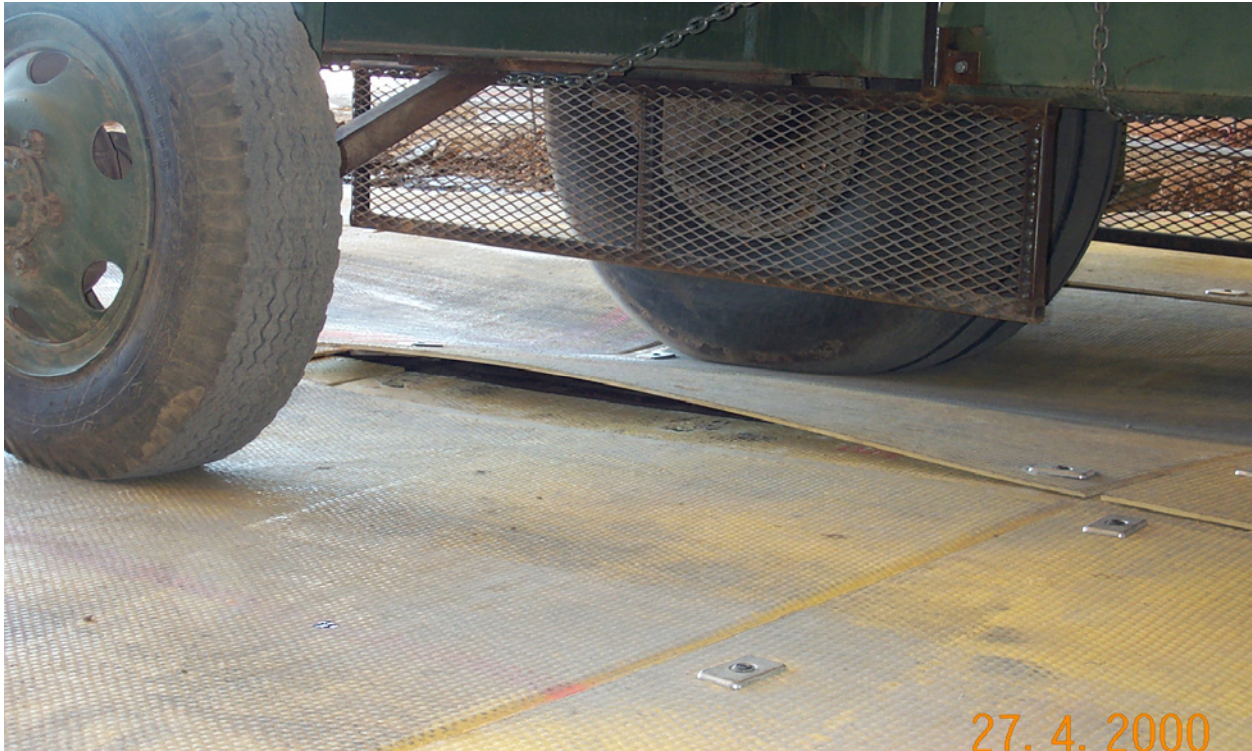
Photo 37. Secondary deflection of MP Mat on low-strength soil (3 to 5 CBR)
