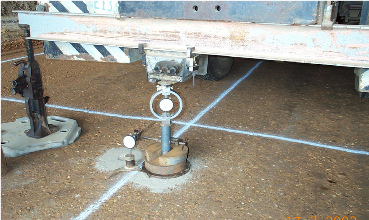
Photo 31. Field CBR test setup
