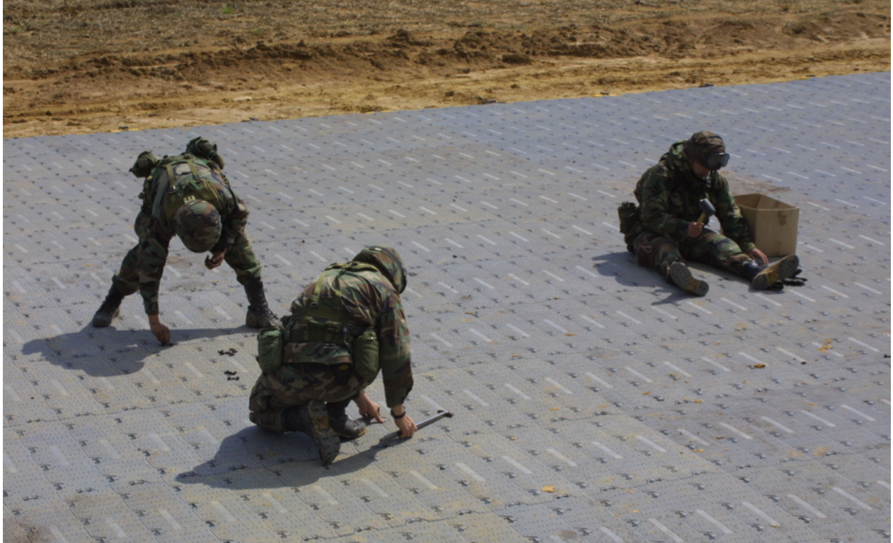
Photo 13. Tapping in SUPA-TRAC connector pins
