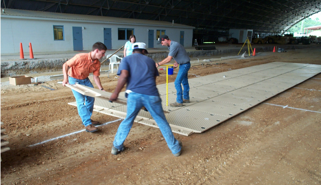
Photo 30. Installing SP-12 matting system
