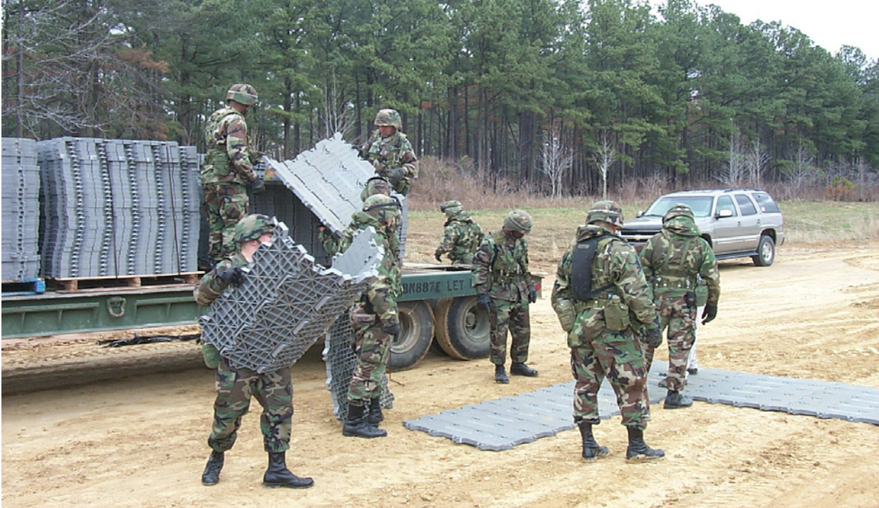
Photo 11. Panels of SUPA-TRAC being carried and placed by soldiers
