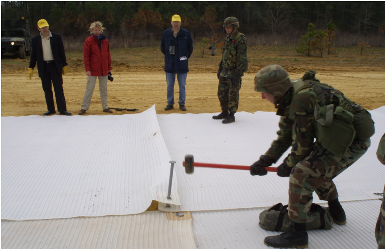
Photo 6. Hammering corner stakes into Mobi-Mat panels
