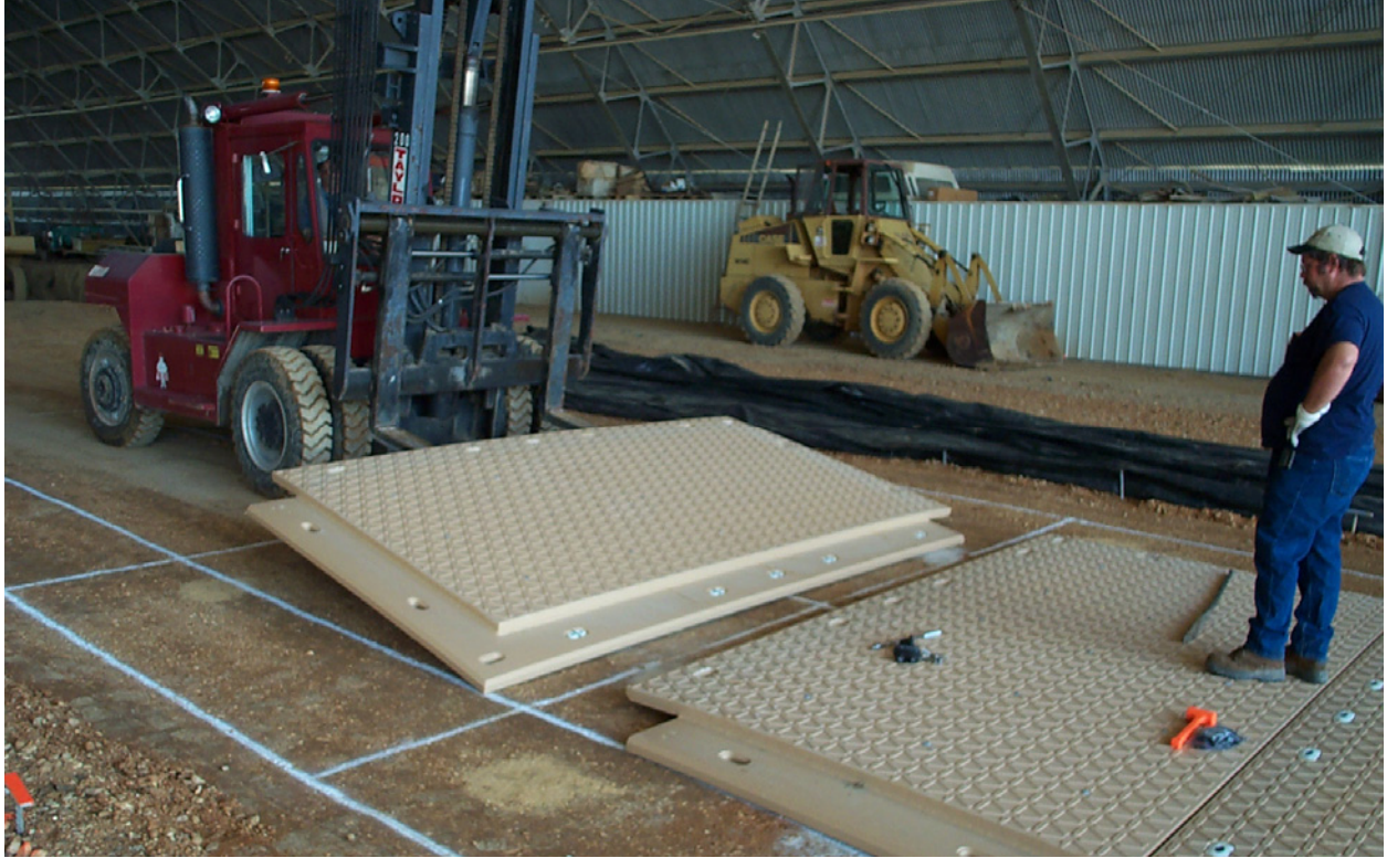
Photo 26. Installing DURA-BASE matting system
