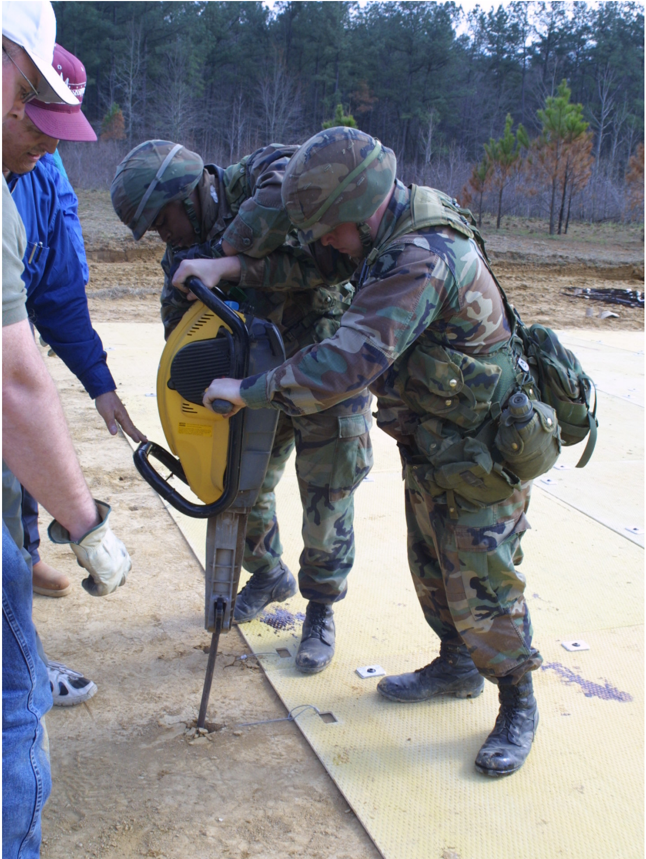
Photo 19. Gasoline-powered jackhammer used to drive duckbill anchors into ground
