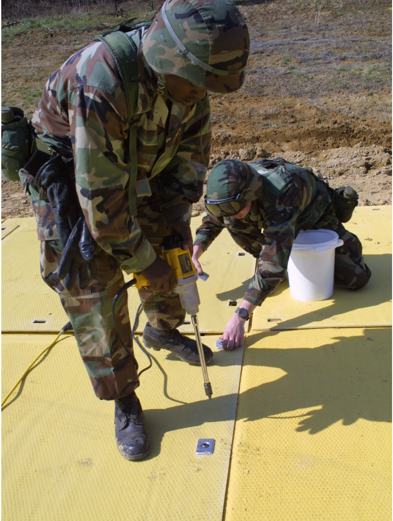
Photo 17. Placing MP Mat connector pins and locking pins with electric impact wrench
