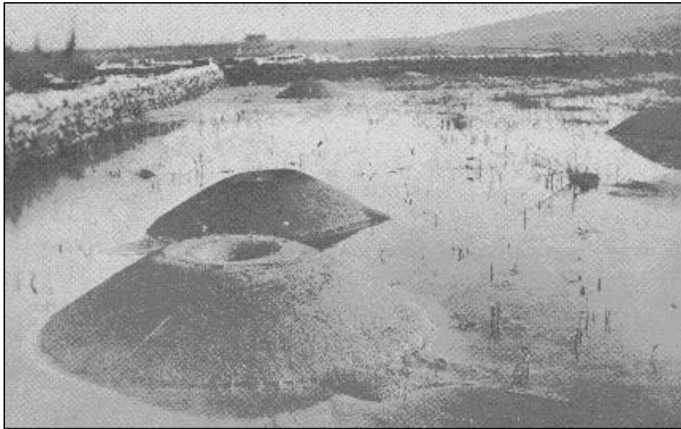
Figure 1. Sand boils at Trotters, MS, 1937, lower Mississippi River (USACE 1956b)
