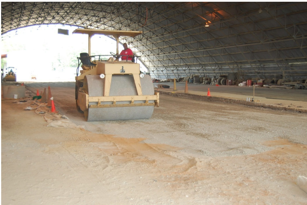
Figure 24. Final compaction of base course using steel-drum roller.
