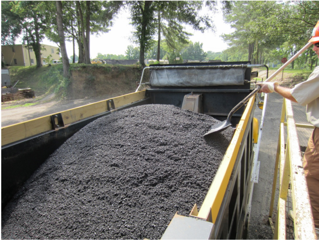
Figure 29. Sampling asphalt mixture from delivery trucks.
