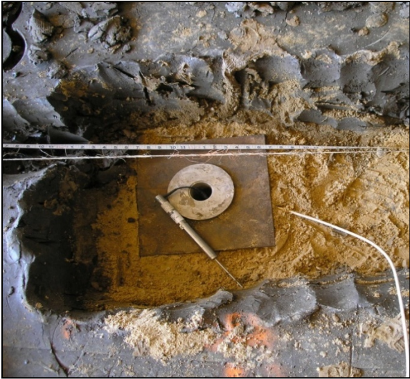
Figure 59. Typical SDD gauge installation.
