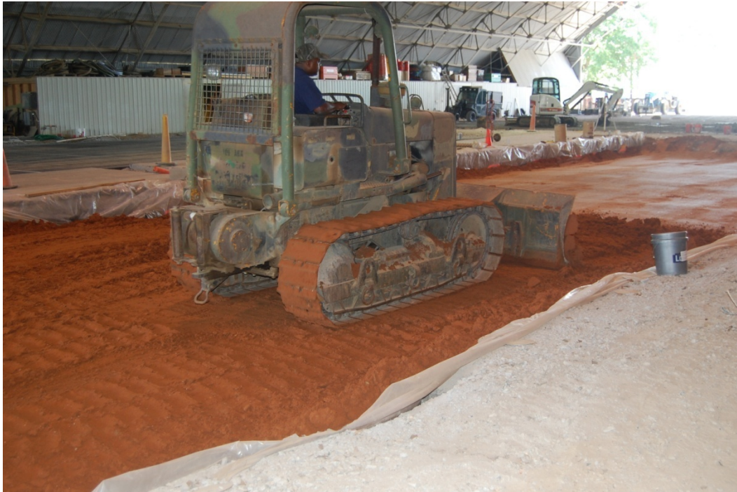
Figure 20. Spreading subbase soil with bulldozer.
