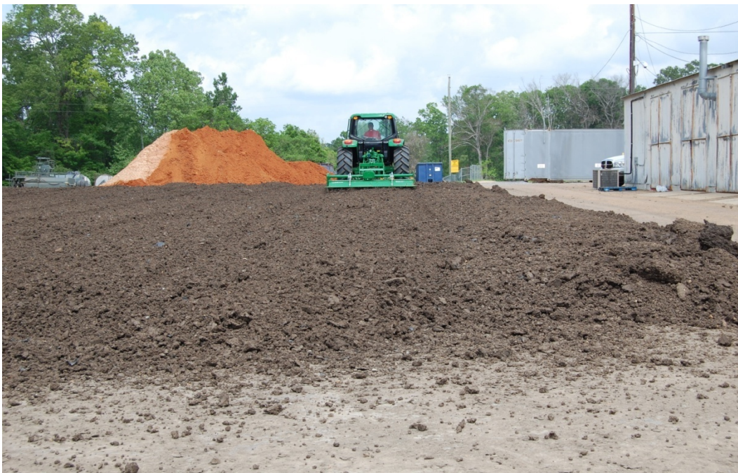
Figure 15. Processing subgrade soil to adjust moisture content.
