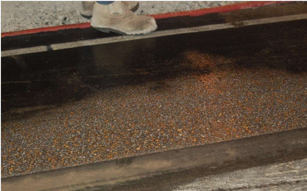
Figure 37. Pavement surface after grinding.
