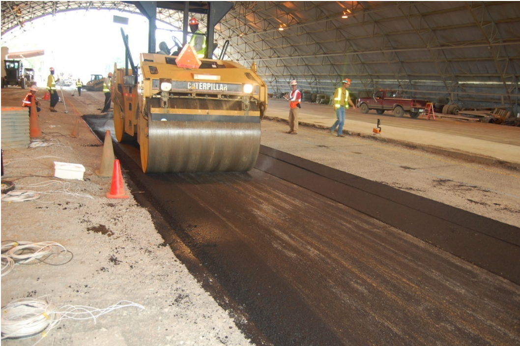
Figure 33. Breakdown rolling of asphalt concrete using vibratory compactor.
