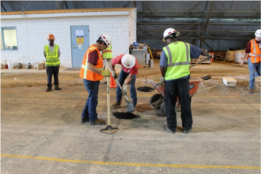
Figure 56. Installing asphalt strain gauge.
