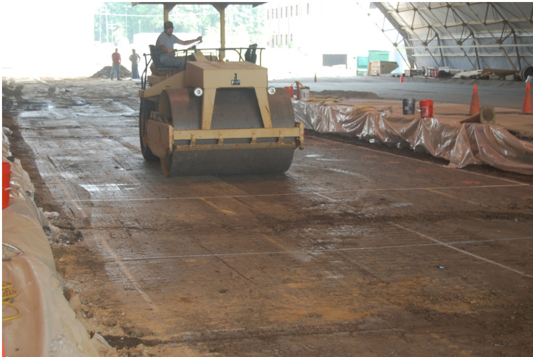
Figure 19. Smoothing surface of subgrade with steel-wheeled compactor.
