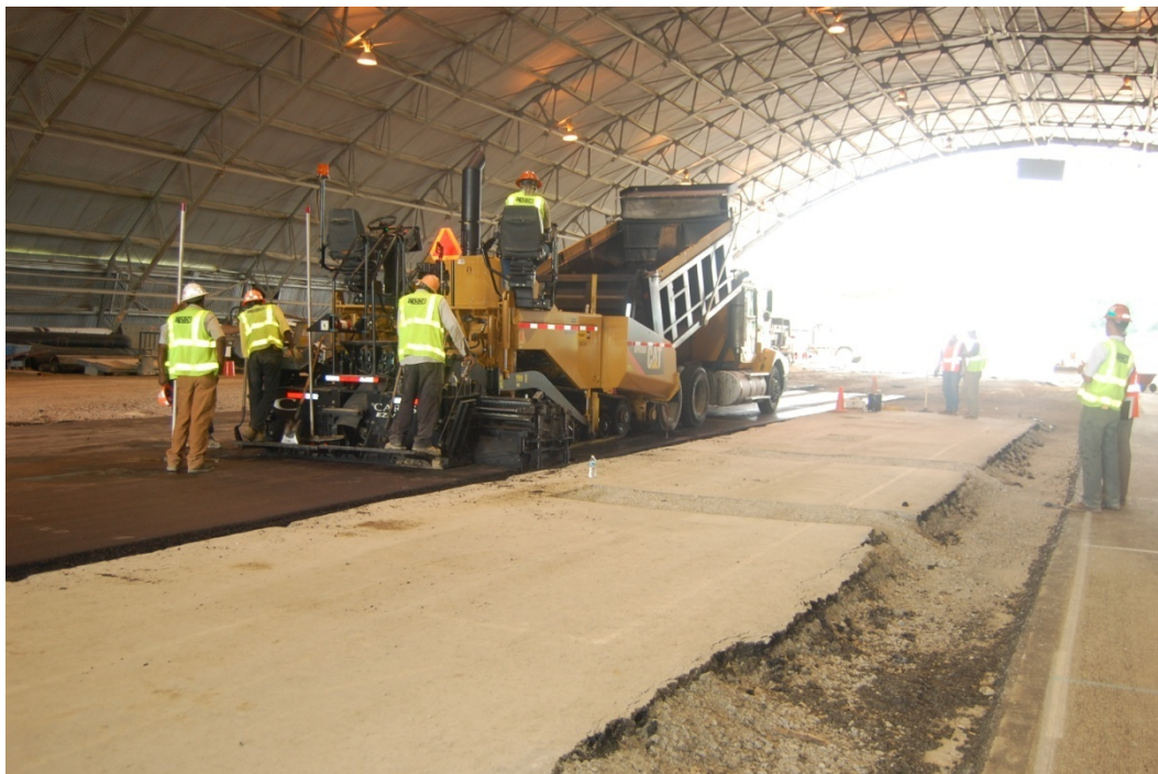
Figure 32. Paving asphalt mixture in covered test facility.
