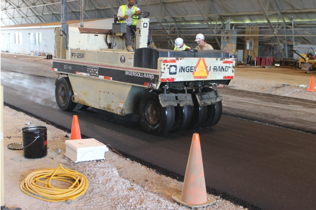
Figure 34. Intermediate rolling of asphalt concrete using pneumatic-tired roller.
