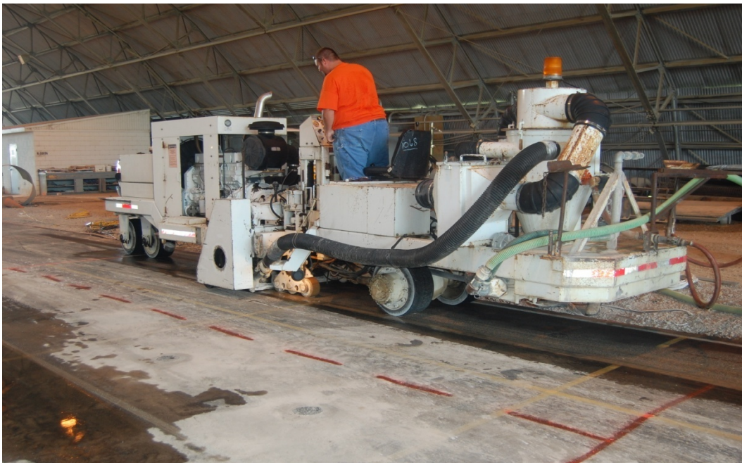
Figure 36. Surface grinding to create uniform asphalt thickness.
