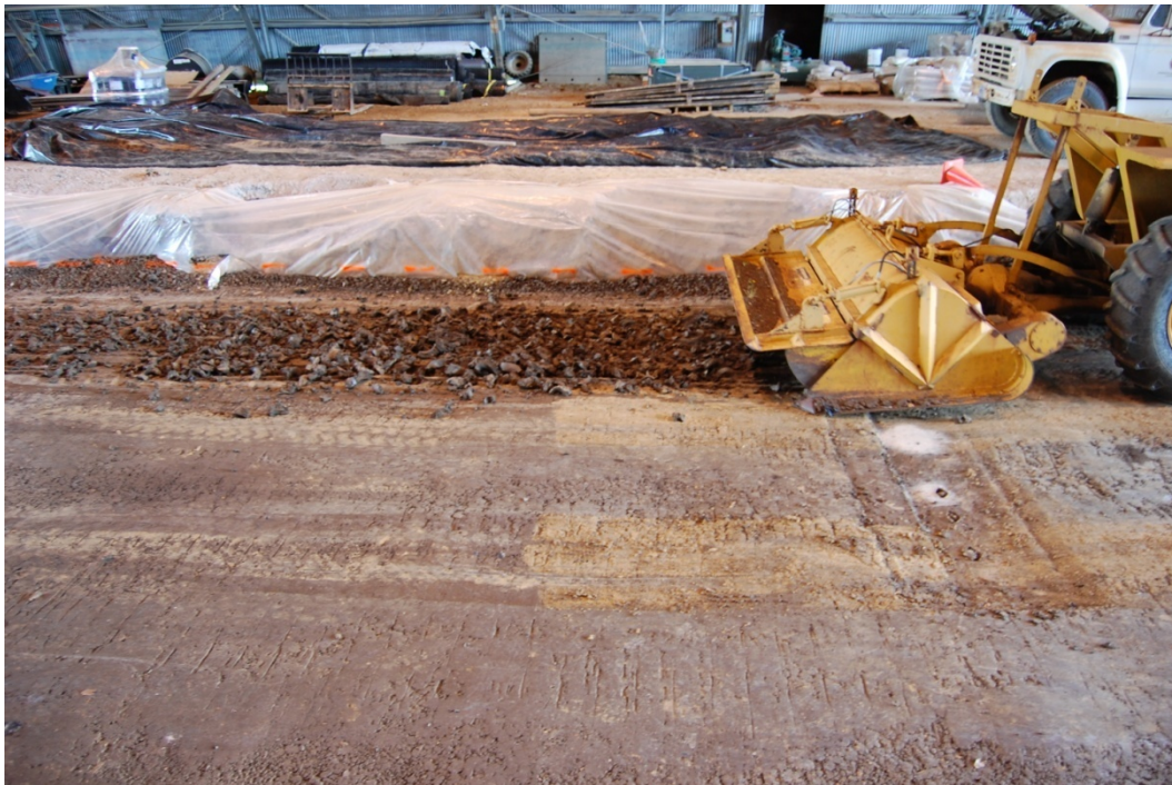
Figure 17. Scarifying surface of subgrade lift to achieve bond between layers.
