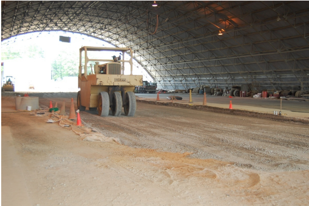
Figure 23. Compacting base course with pneumatic roller.
