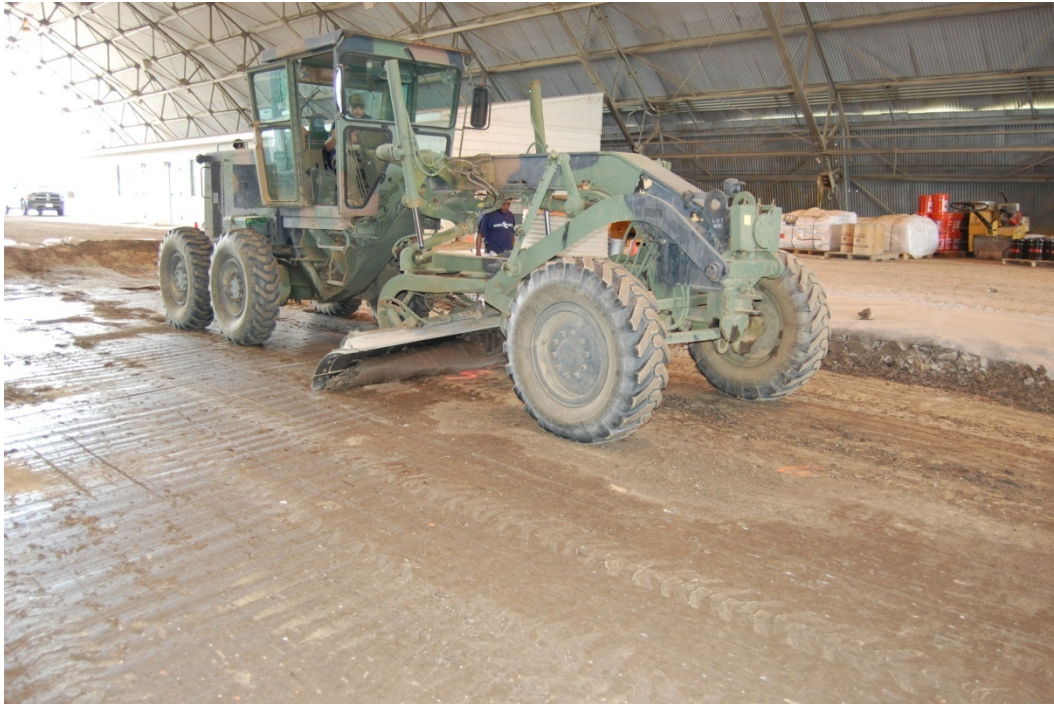
Figure 18. Establishing final grade of subgrade surface.
