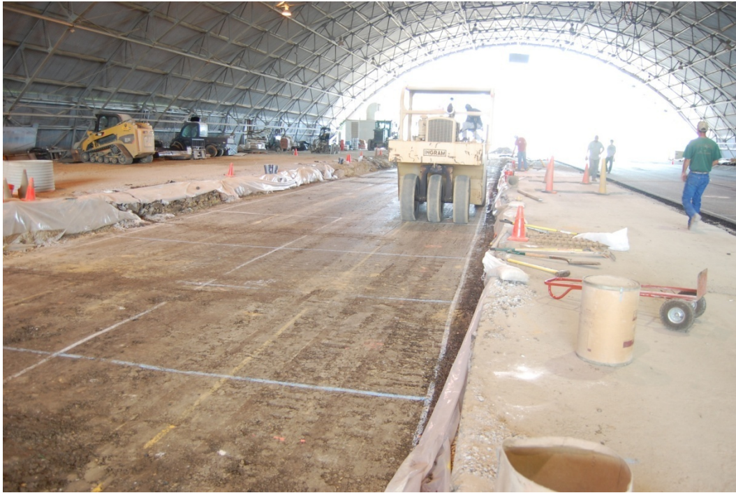
Figure 16. Compacting subgrade with pneumatic-tired roller.
