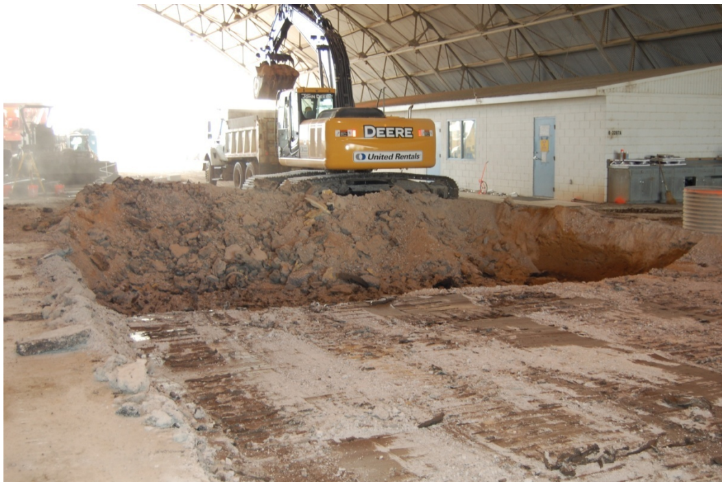
Figure 14. Excavating soil for test section construction.
