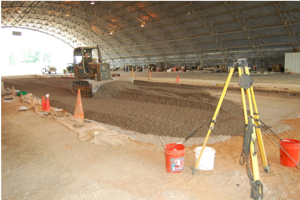
Figure 21. Spreading base material using a bulldozer.
