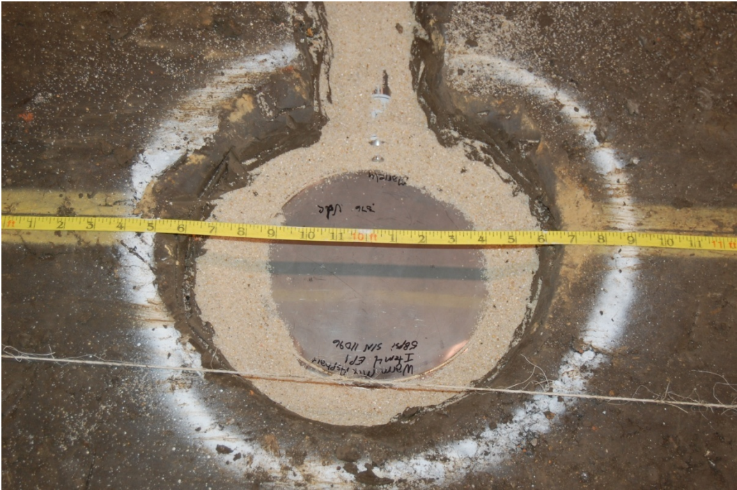
Figure 58. Typical earth pressure cell installation.
