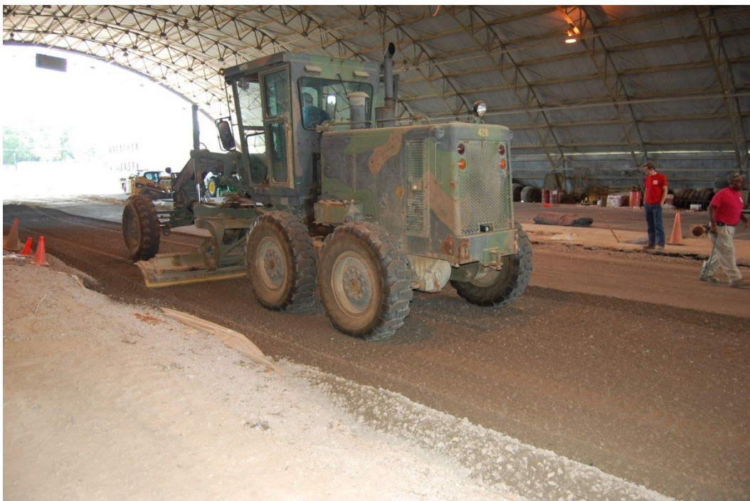
Figure 22. Grading base course surface.
