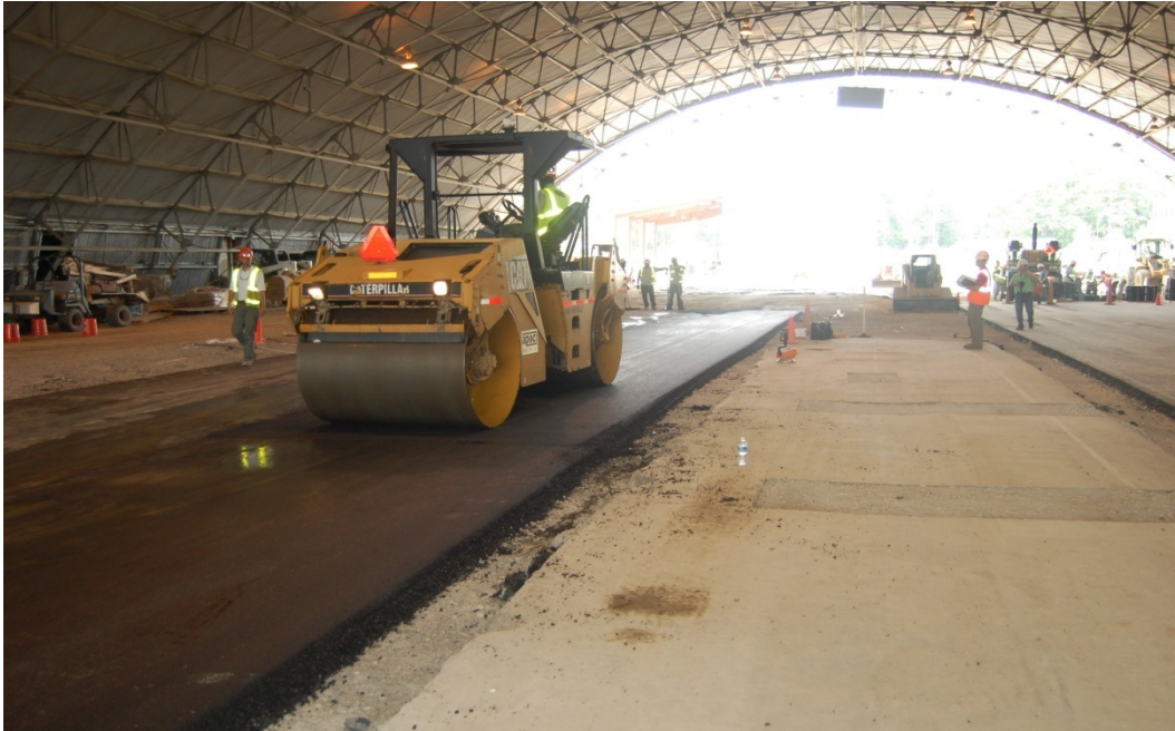
Figure 35. Finish rolling asphalt concrete using static steel-wheel compactor.
