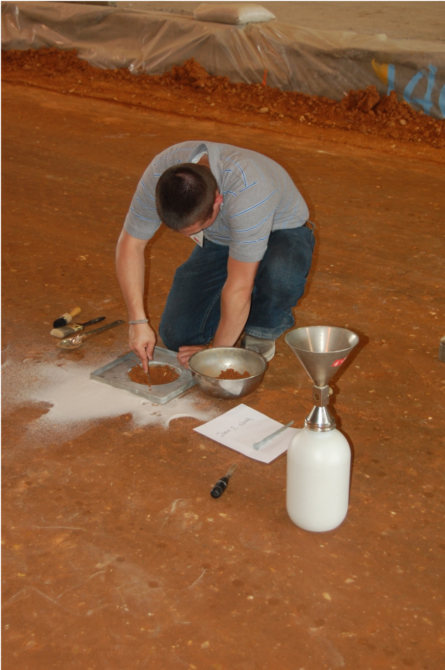
Figure 26. Performing density tests on compacted subbase using sand cone method.
