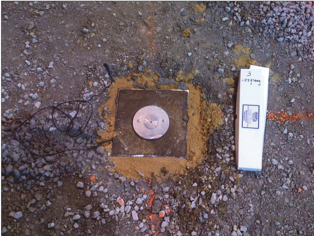
Figure 36. SDD after installation.
