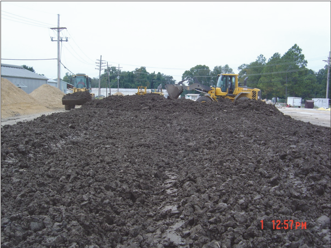
Figure 20. Subgrade material processing.
