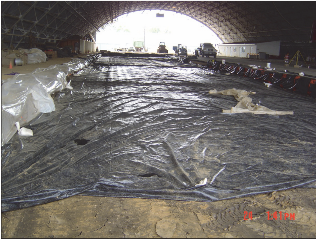
Figure 22. Subgrade layer covered after compaction.
