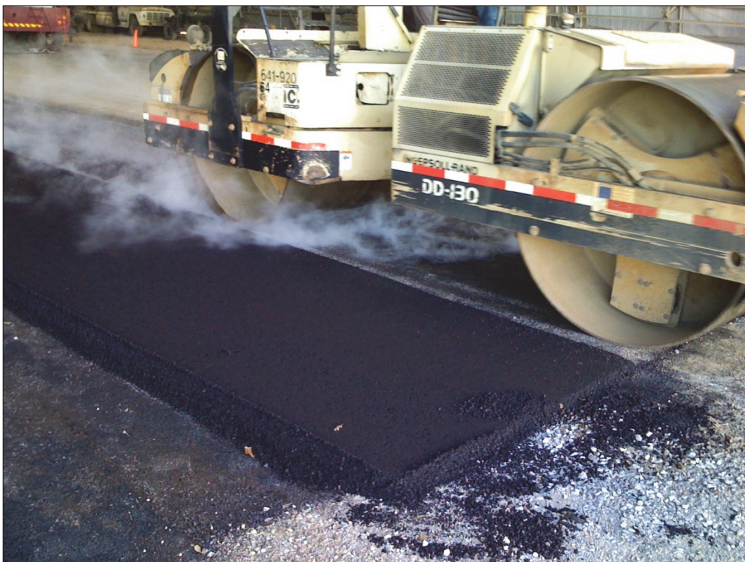
Figure 30. Paving operations, break-down rolling.
