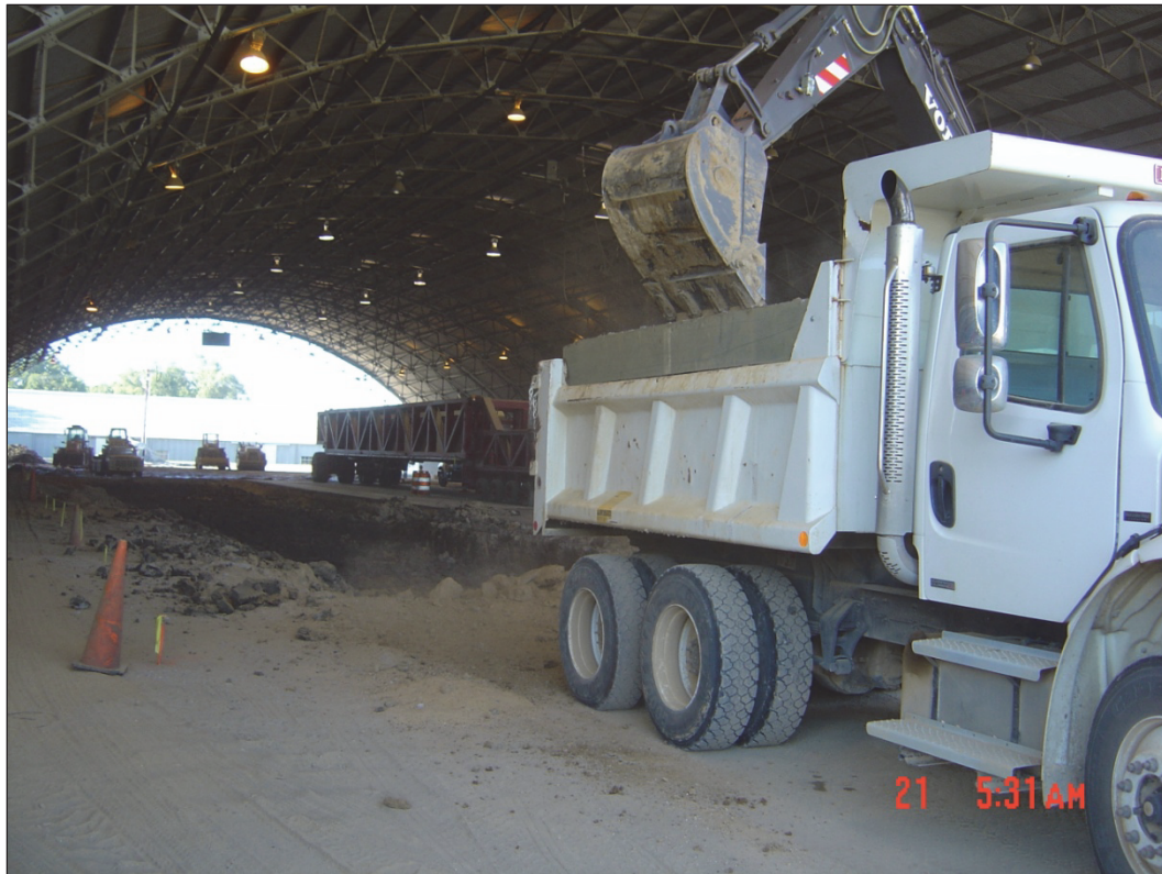
Figure 18. Test section excavation.
