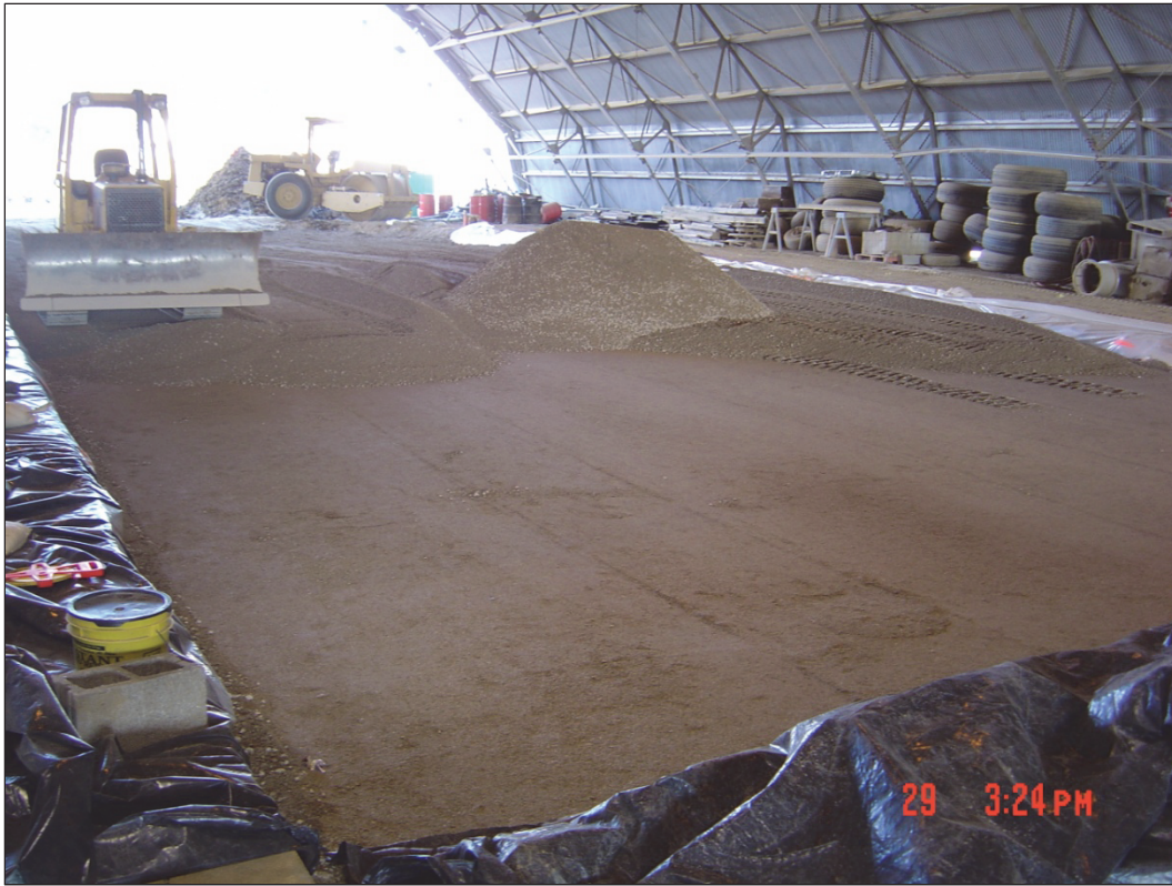
Figure 25. Subbase placement activities.
