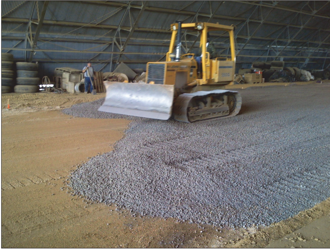
Figure 27. Base layer placement.
