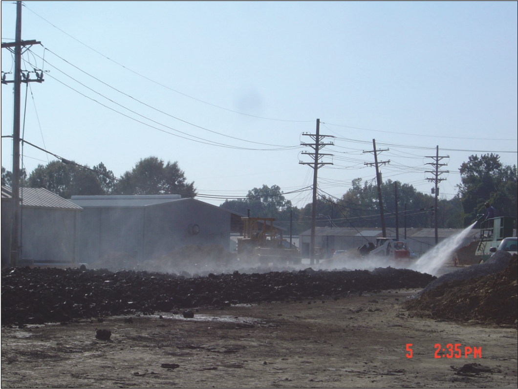
Figure 19. Adding water to the subgrade material.
