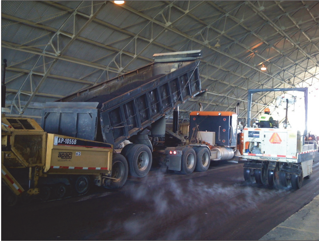
Figure 31. Paving operations, rubber-tire roller compaction.
