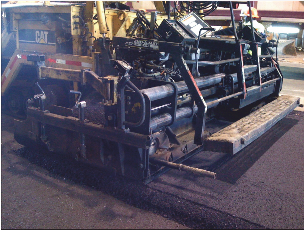
Figure 29. Paving operations, mat placement.
