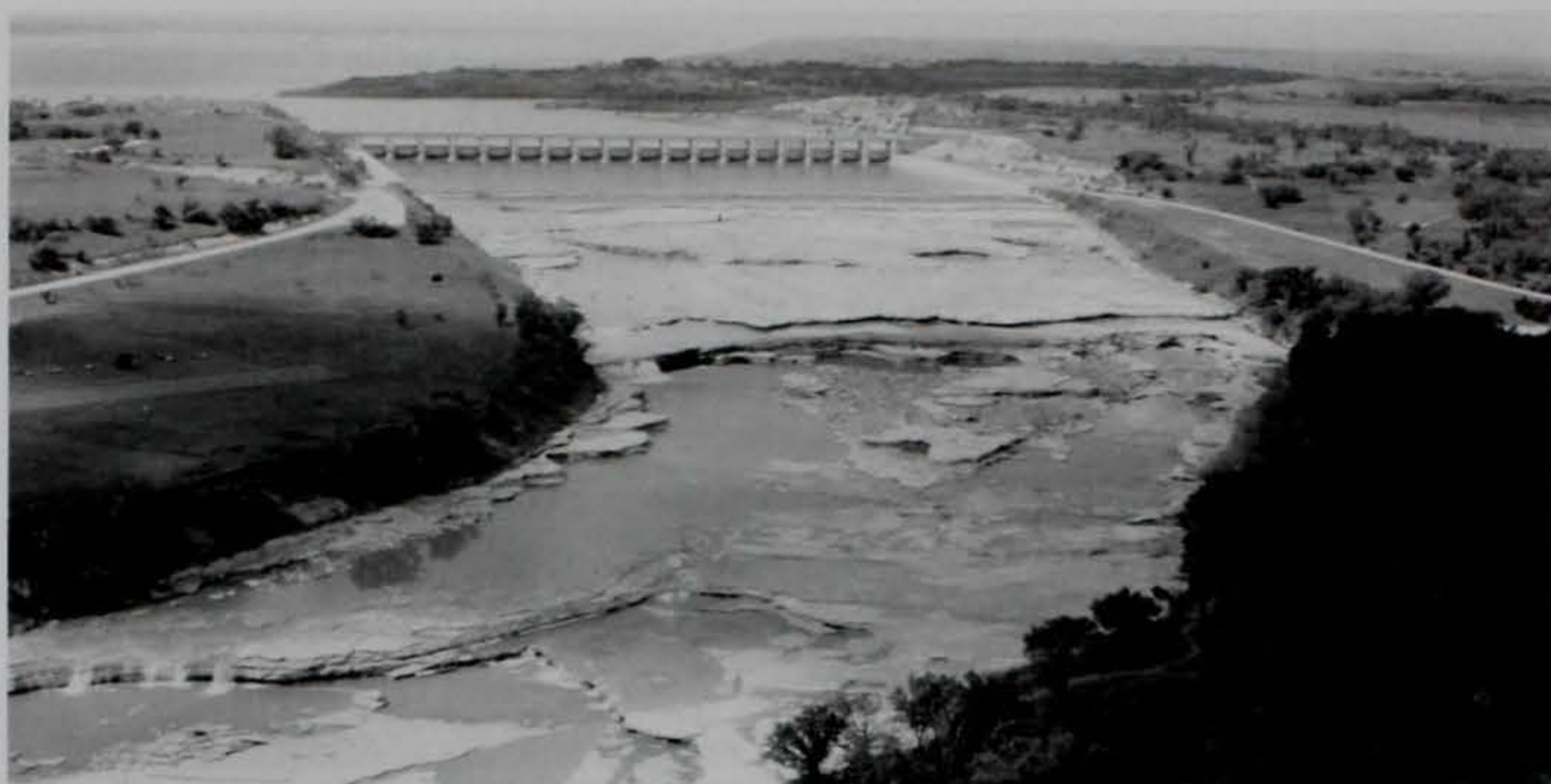
Figure 16. Tuttle Creek Spillway after being used during the Flood of 1993.
