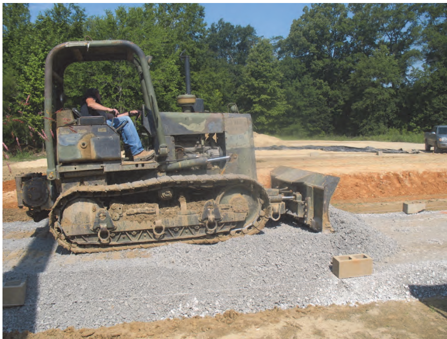
Figure 18. Leveling of loose GP-GM material prior to compaction with bulldozer.
