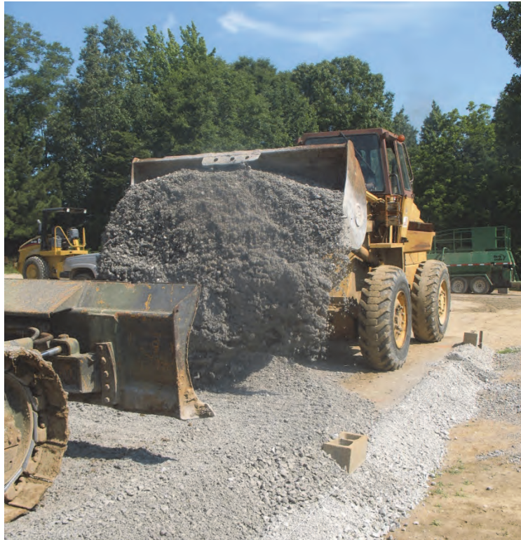
Figure 17. Placement of loose GP-GM soil prior to compaction with front-end loader.
