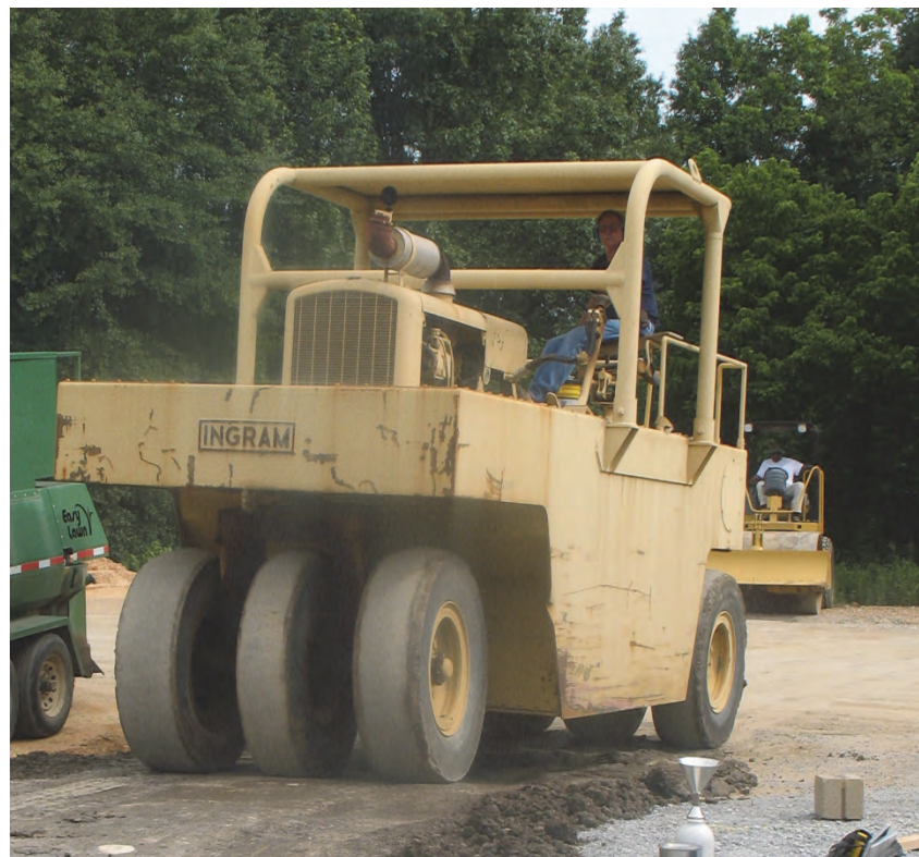
Figure 20. 7-Tire Ingram Rubber Tire Roller used in CH compaction.
