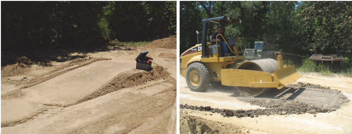
Figure 25. Low moisture-low density calibration pad for EDG on ML-1 (left) and CH (right)
