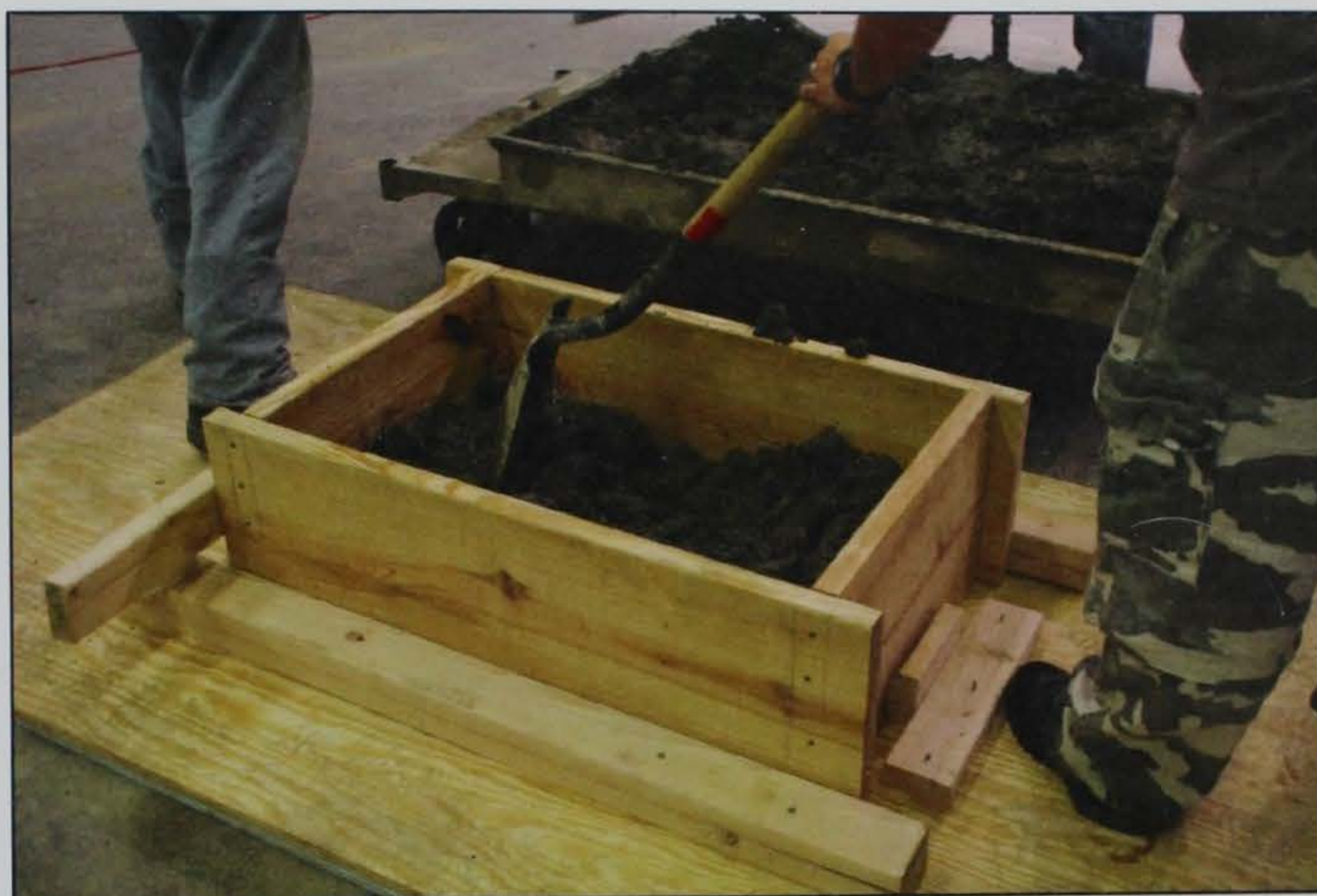
Figure 8. Pouring a concrete mixture into a wooden frame.
