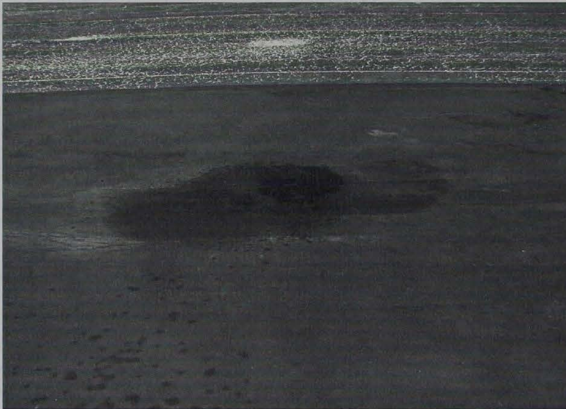
Figure 7. E-Krete section at MacDill AFB exhibiting staining from synthetic jet turbine lubricant
