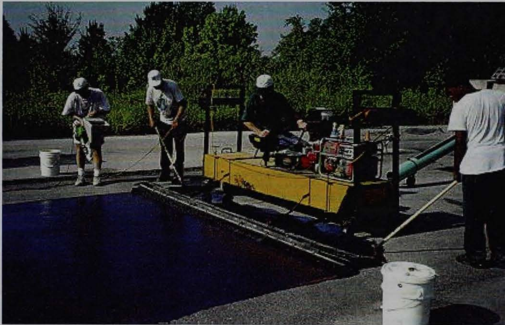
Figure 2. Application of E-Krete at ERDC, August 1998
