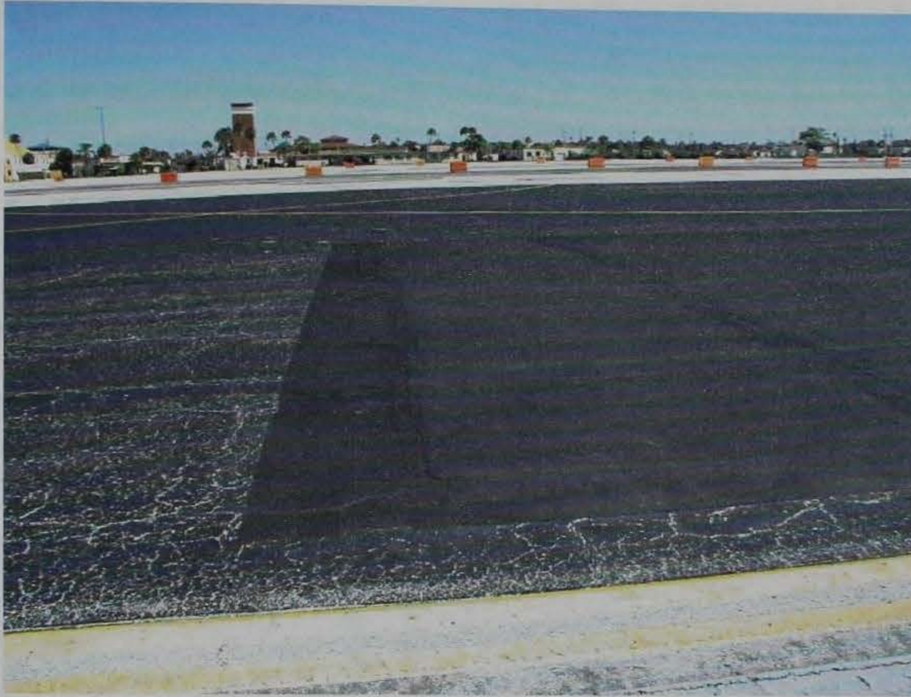
Figure 5. E-Krete surface in October 2000 at MacDill AFB. The adjacent pavement is coal tar that is approximately 14 years old and is severely deteriorated
