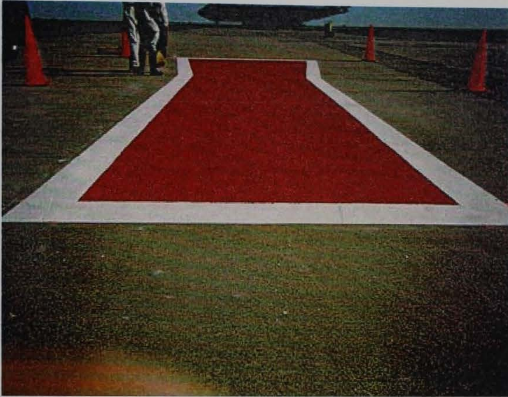
Figure 18. "Red Carpet" area at Forbes Field in November 1998. This E-Krete section was placed to provide a walkway for dignitaries exiting aircraft
