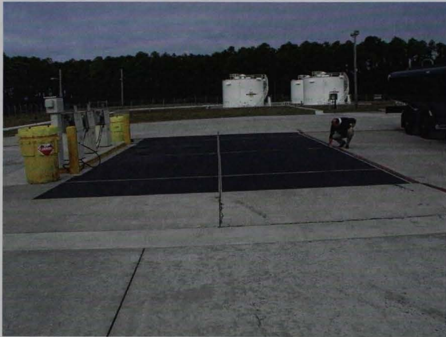
Figure 9. E-Krete section in fuel depot at Tyndall AFB, October 2000
