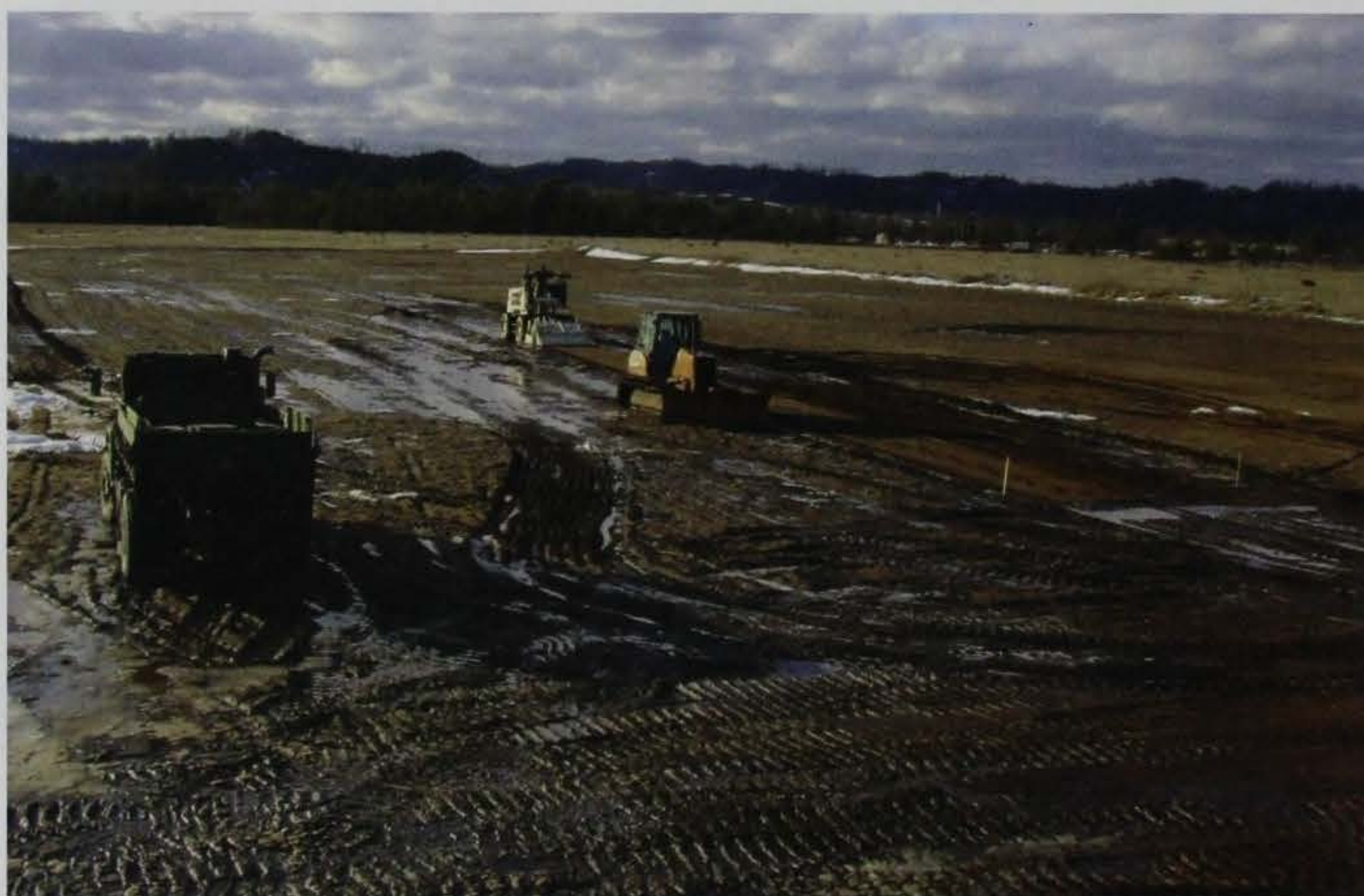
Figure 12. Subgrade preparation at Engineer Dig Site 09, Fort McCoy, WI.
