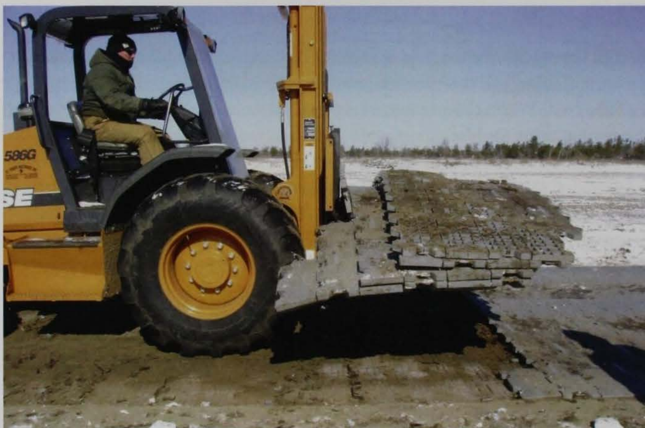
Figure 68. Removal of matting with a forklift on SC-2 test section.
