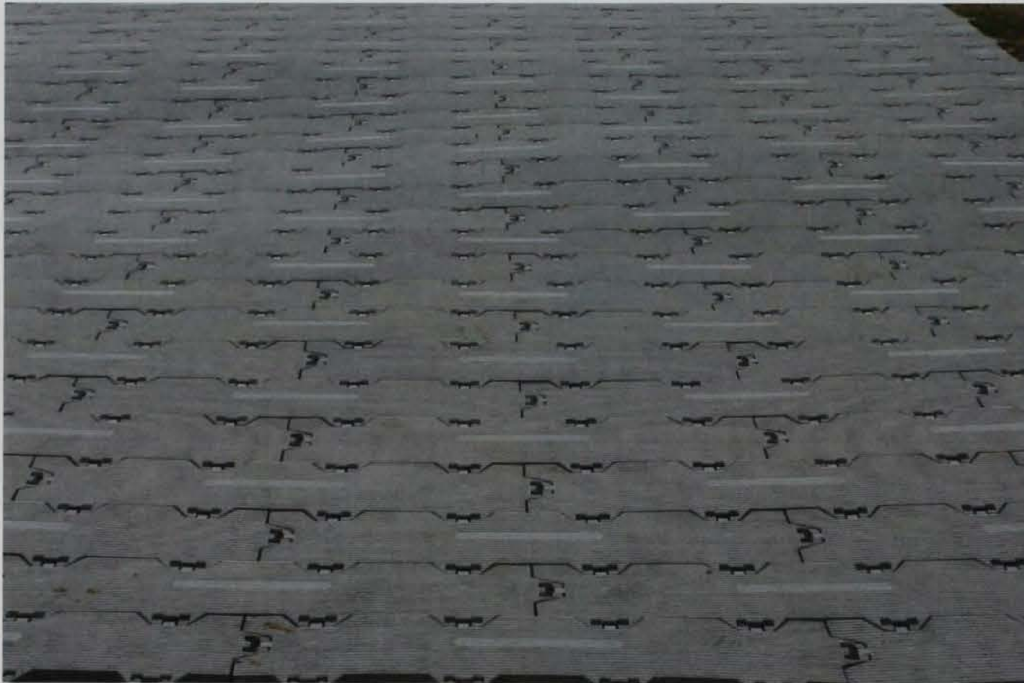
Figure 3. Supa-Trac configured with staggered longitudinal joints.
