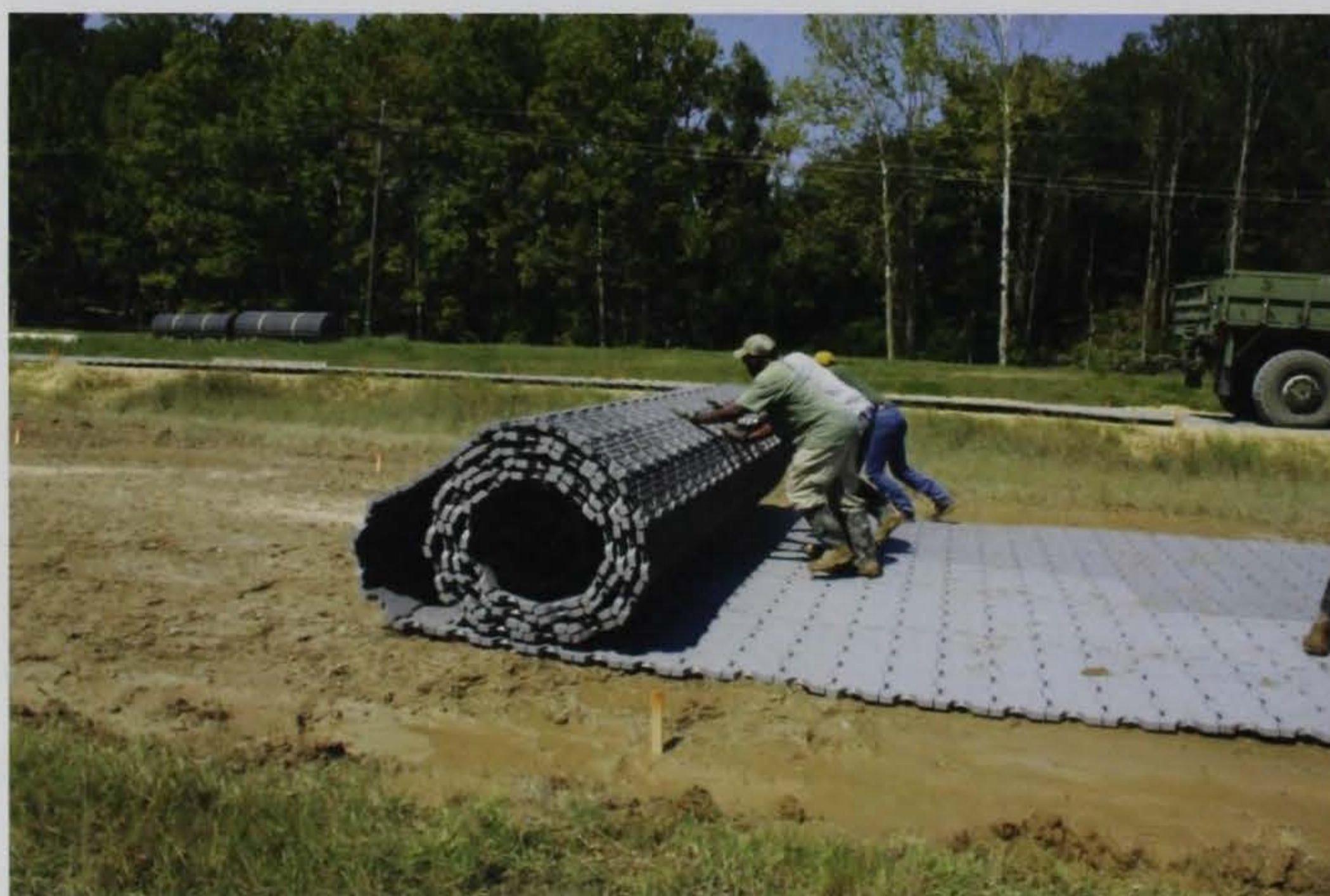
Figure 15. Installation of Supa-Trac matting on SM-1 test section.
