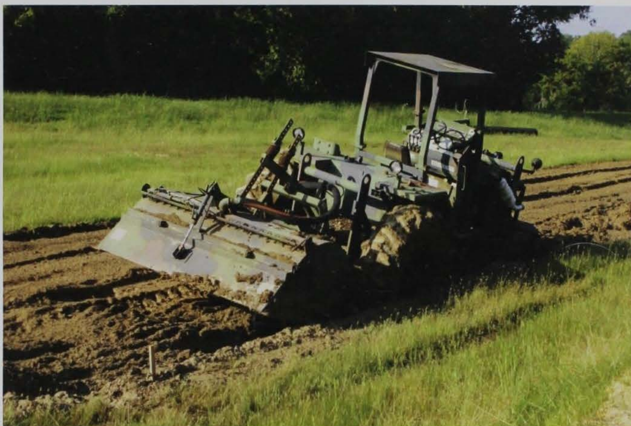
Figure 6. SM-1 test section subgrade construction.
