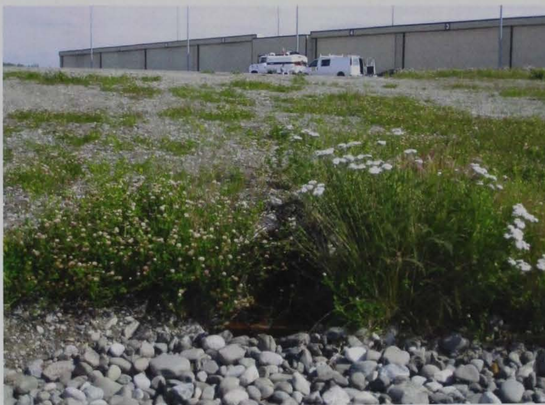
Figure 22. Outlet pipe leading from weather shelter apron.
