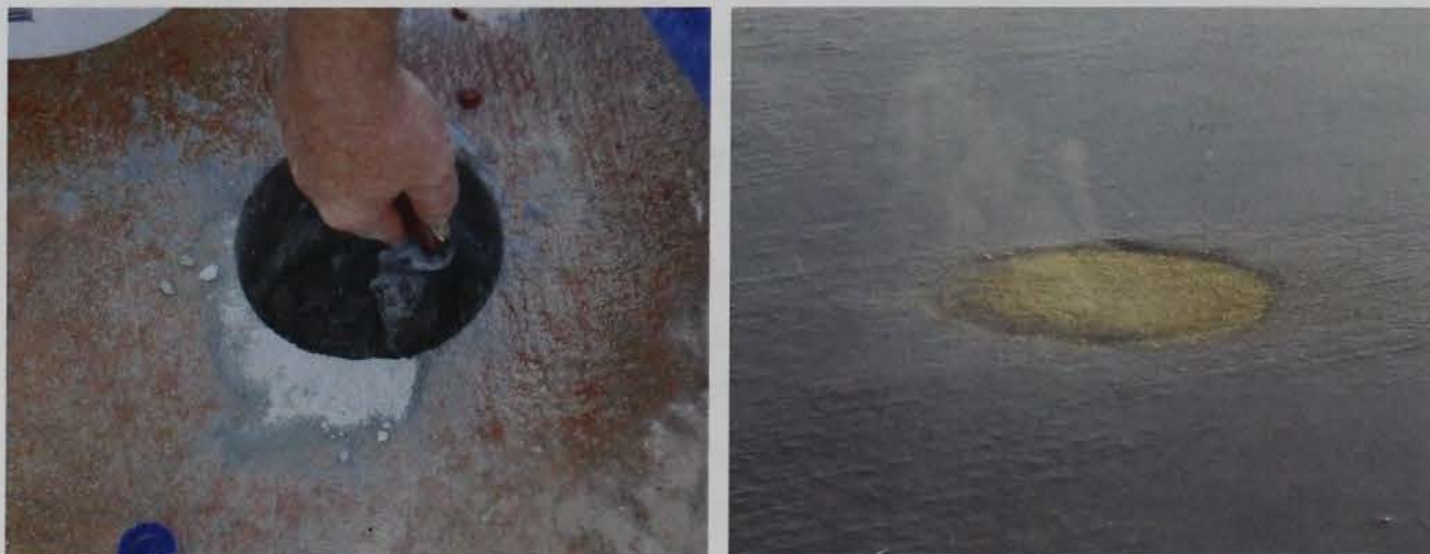
Figure 9. Core hole patching.
