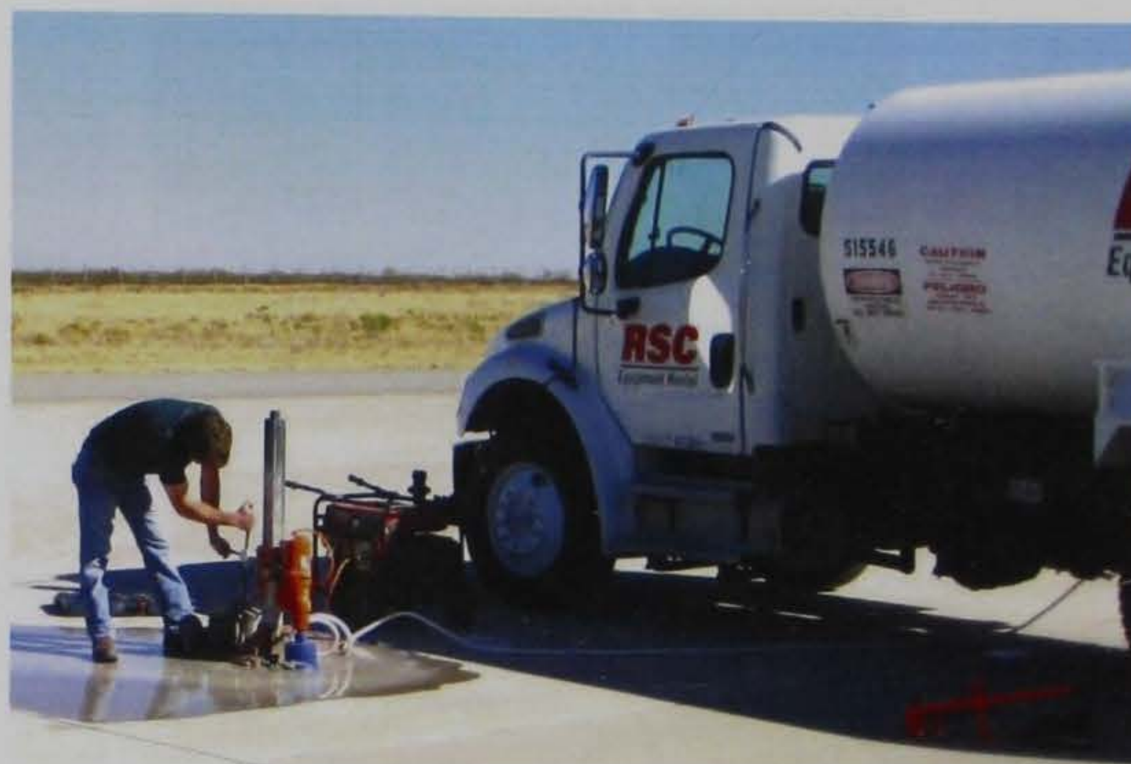
Figure 4. Coring and flow test equipment.
