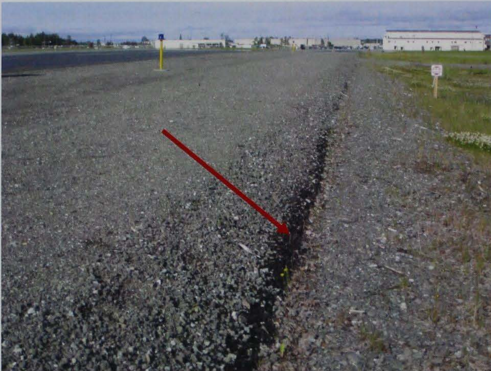
Figure 13. Photo of daylighted drainage layer on fuel cell taxiway.
