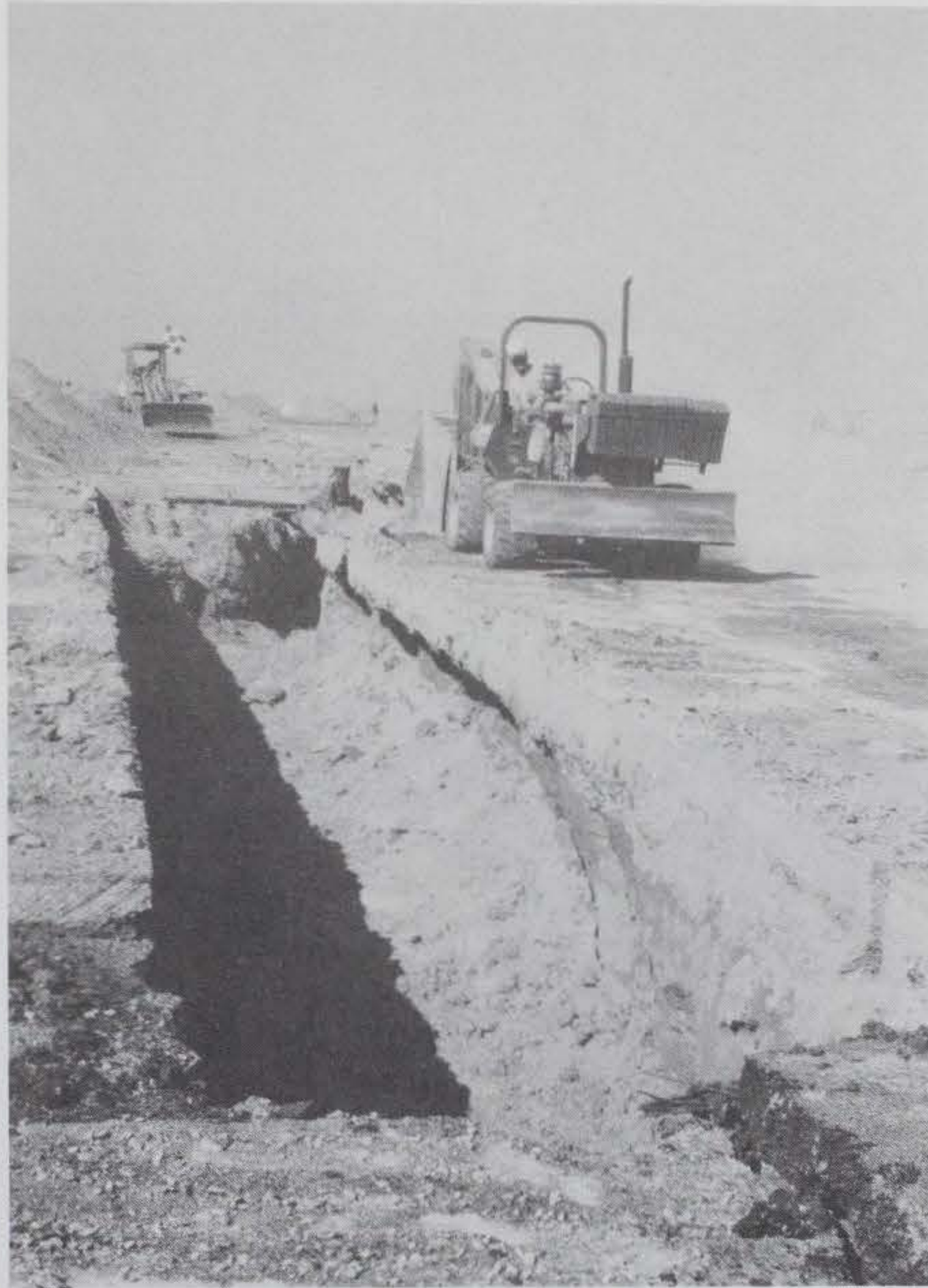
Figure 19. Excavated crack
