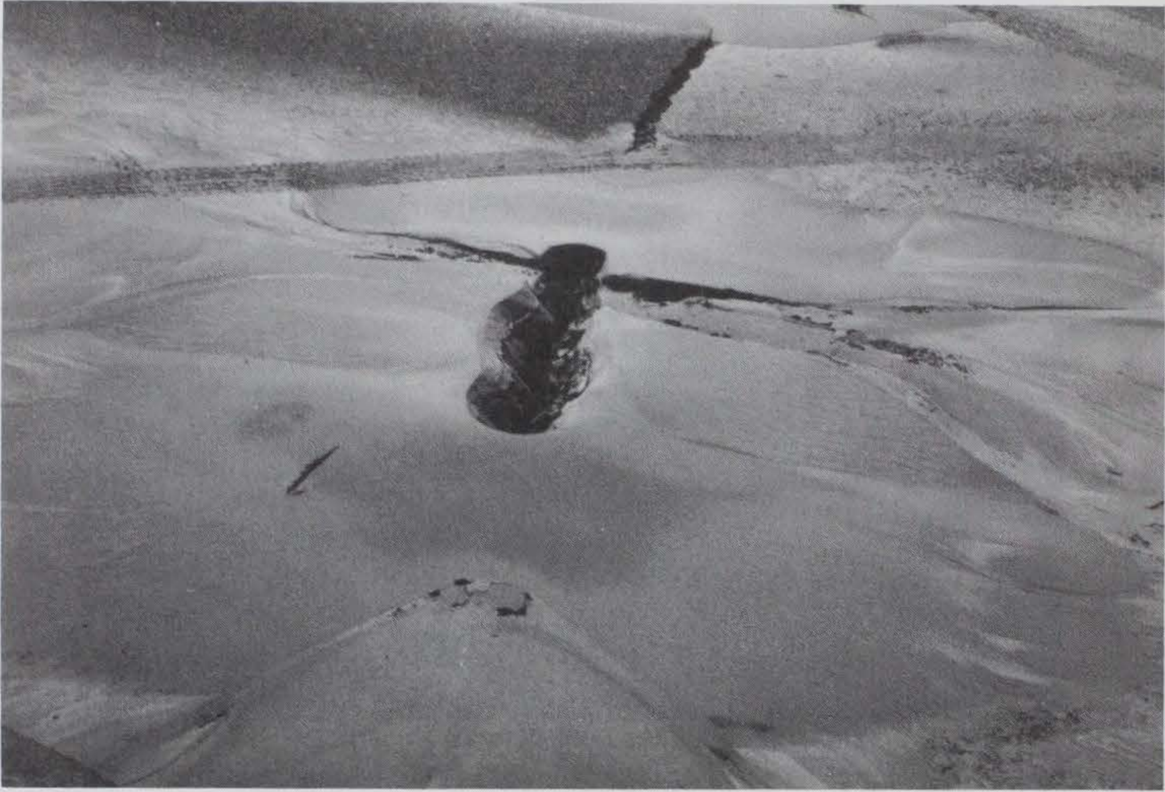
Figure 12. Close-up of sand boil on Runway 11-29
