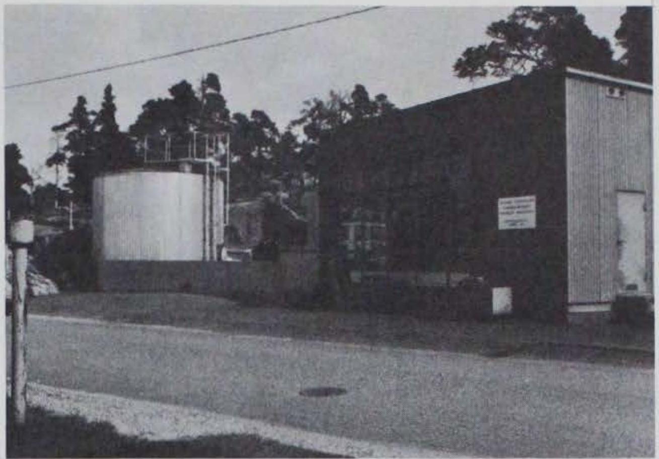
Photo 19. Exterior to Red Hill sewage treatment plant Rauma, Finland
