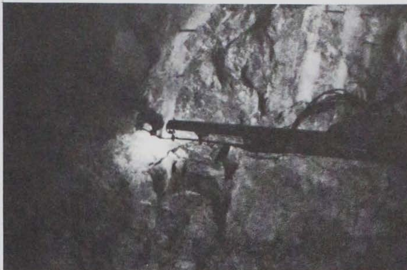
Photo 31. Jumbo drill operating in underground diesel oil facility, Vasteras, Sweden
