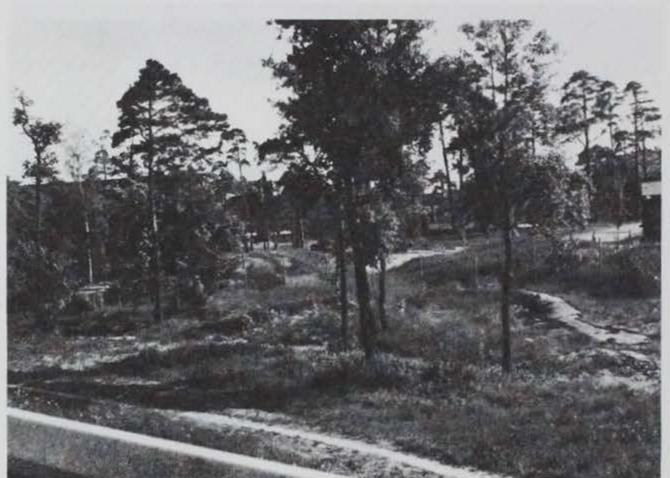
Photo 5. Site of under- ground residual oil stor- age facility, Helsinki, Finland
