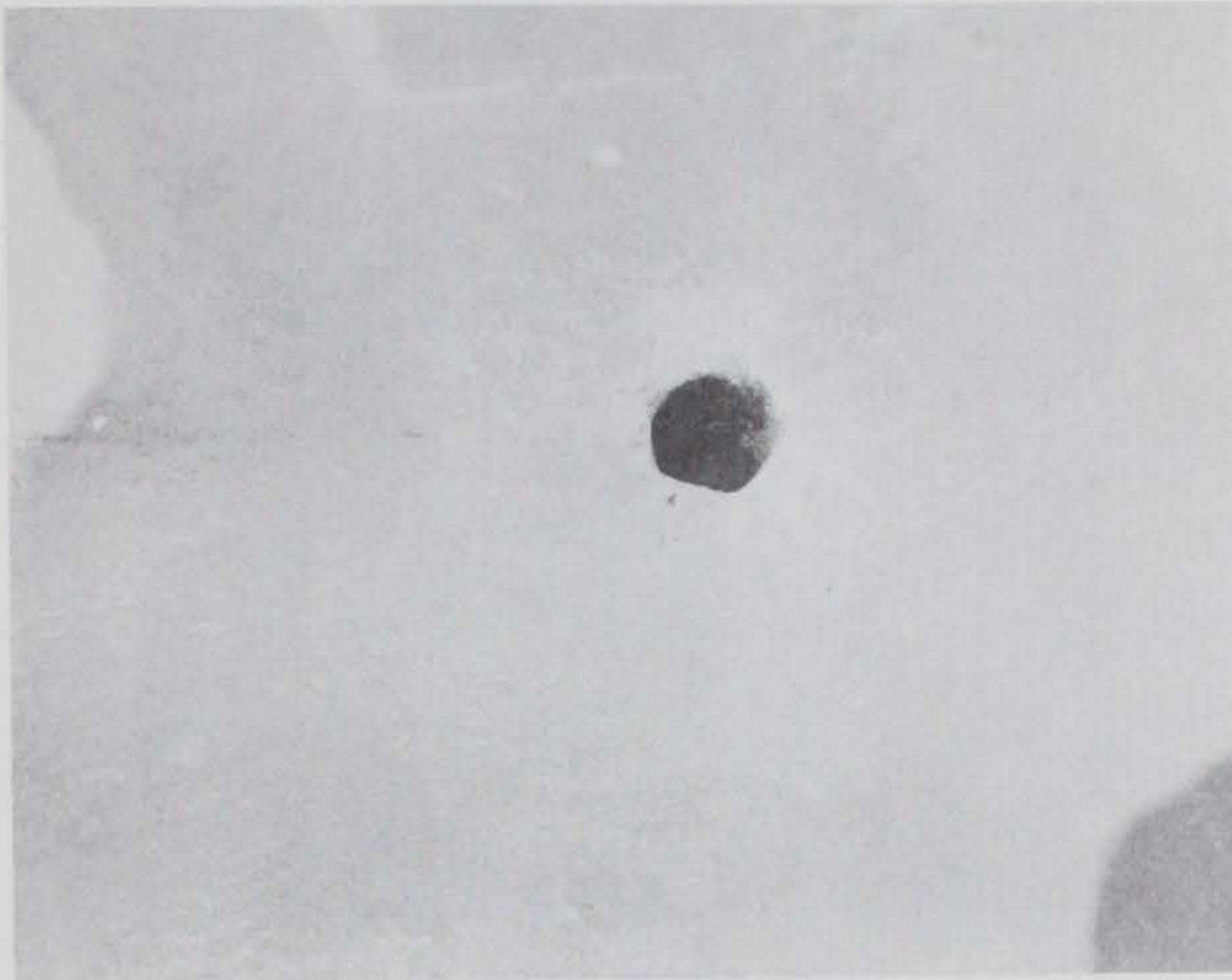
Photo 4. Spalling around hole after test 1, shot 1
