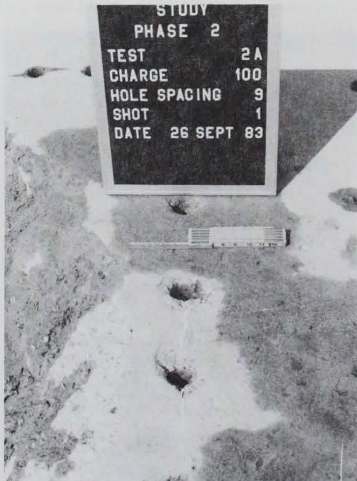
Photo 21. Cracking and spalling resulting from test 2A
