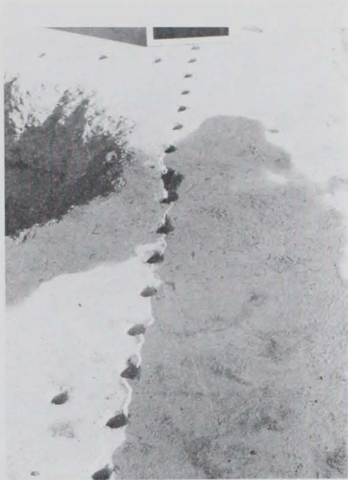
Photo 18. Extent of cracking after test 1, shot 7
