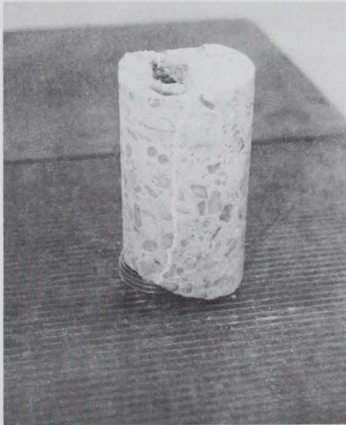
Photo 12. Core taken from test 1A (east side between holes 2 and 3)
