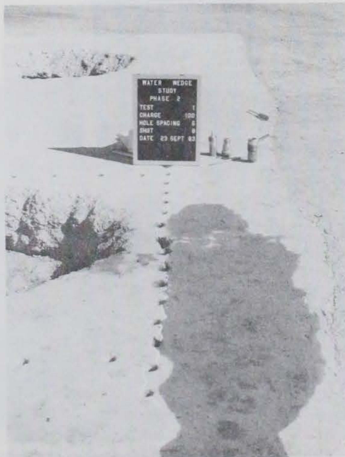
Photo 19. Cracking and spalling after test 1, shot 8
