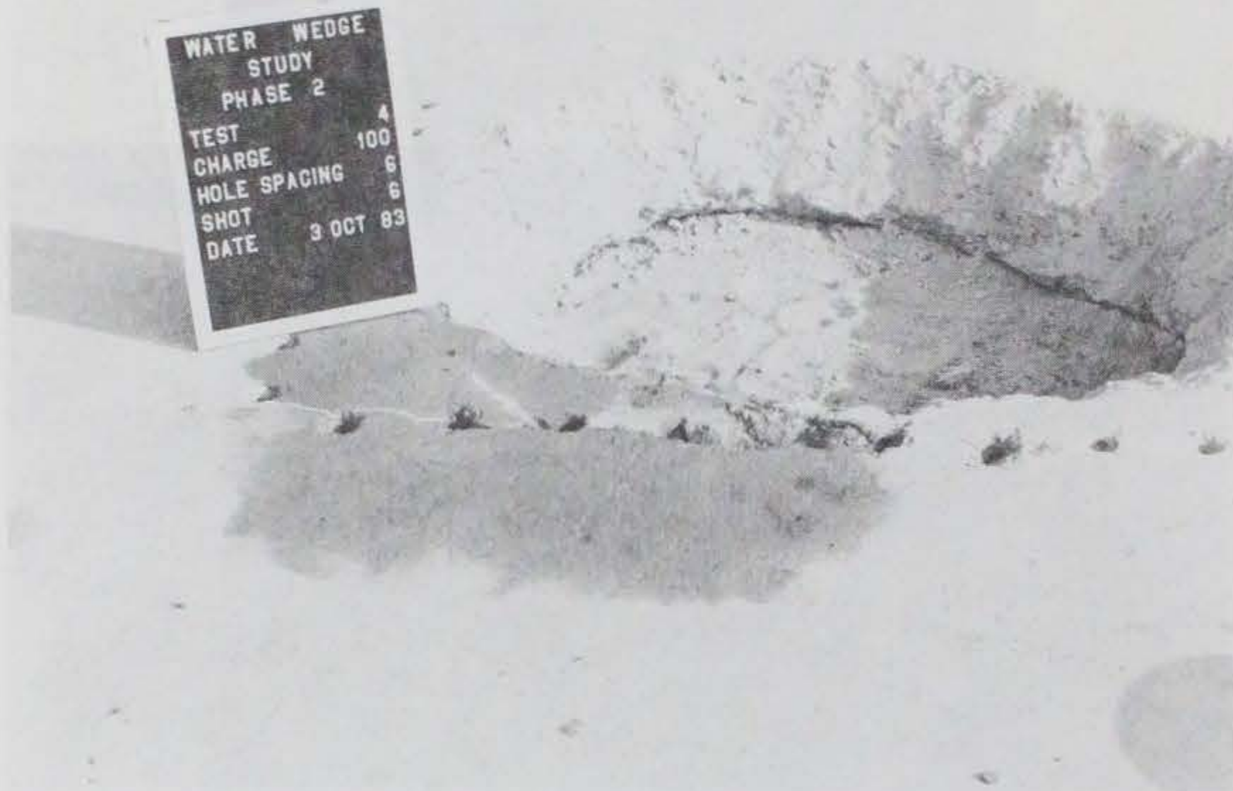
Photo 28. Extent of cracking and spalling after shot 6, test 4
