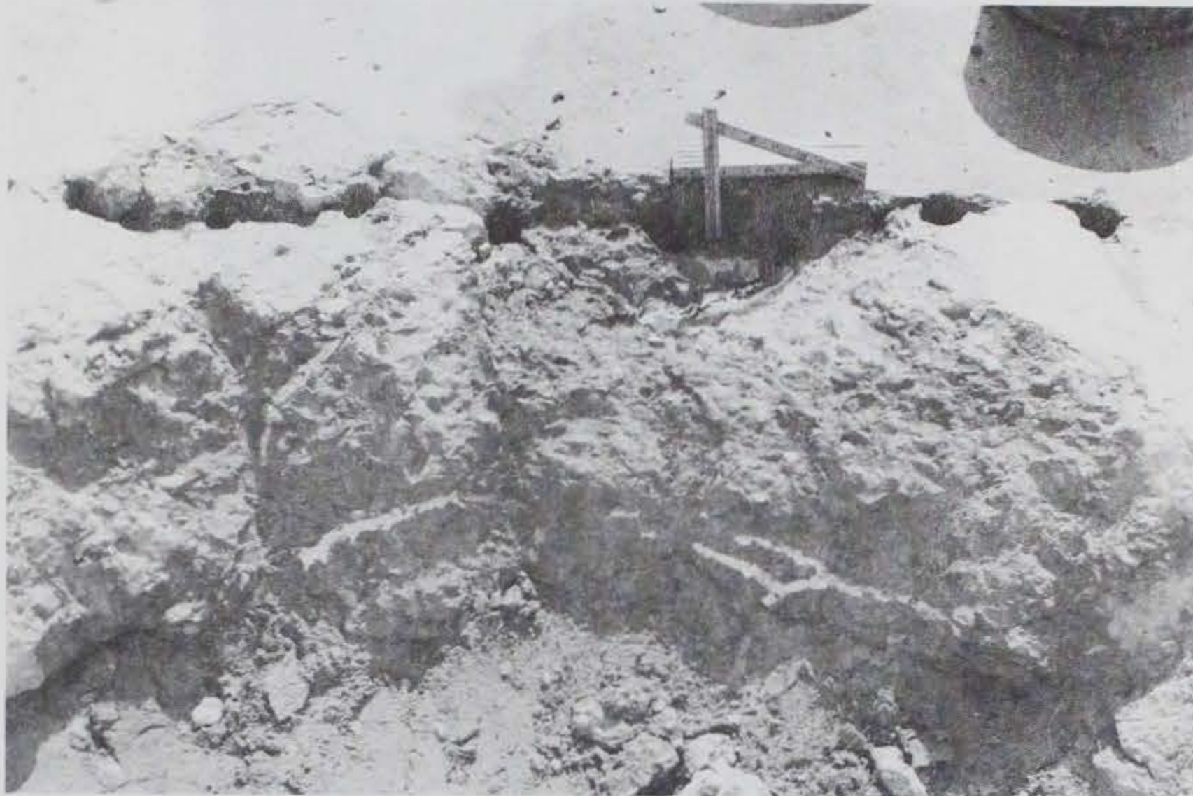
Photo 30. Cracks occurring in wall of crater after shot 23, test 4
