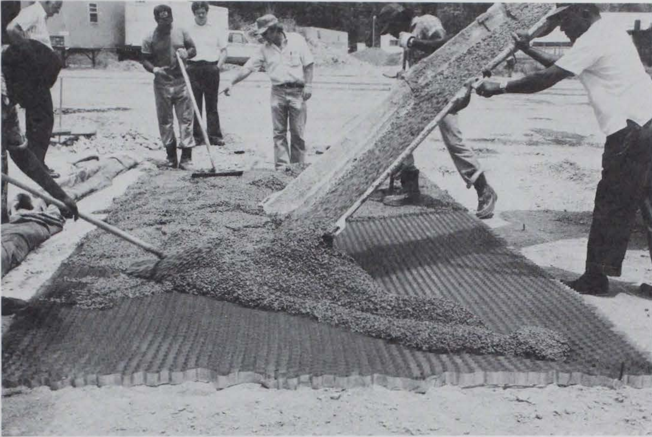
Photo 9. Placing concrete in grids by chute
