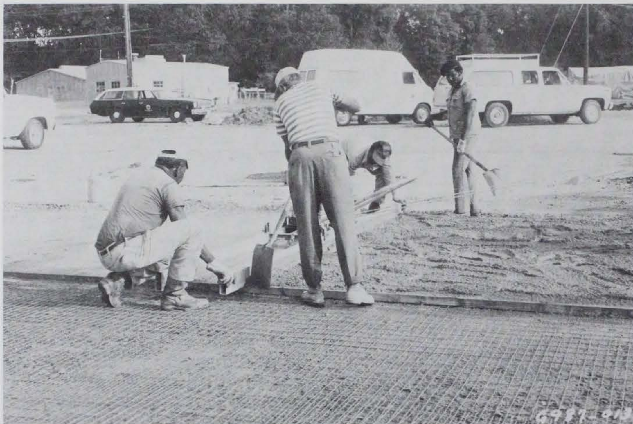
Photo 3. Placing concrete in item 1
