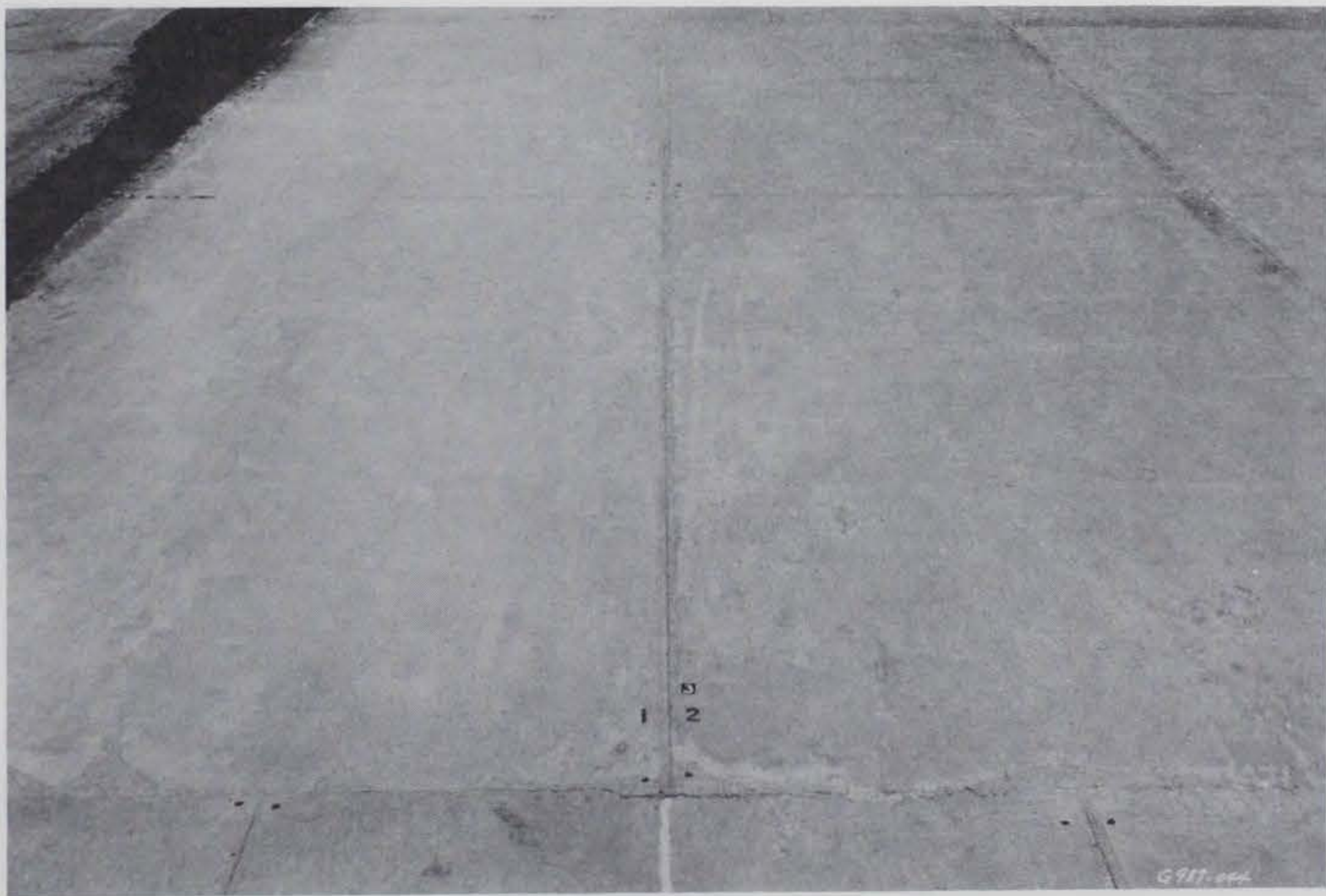
Photo 14. Item 3 showing irregularities in surface due to finishing
