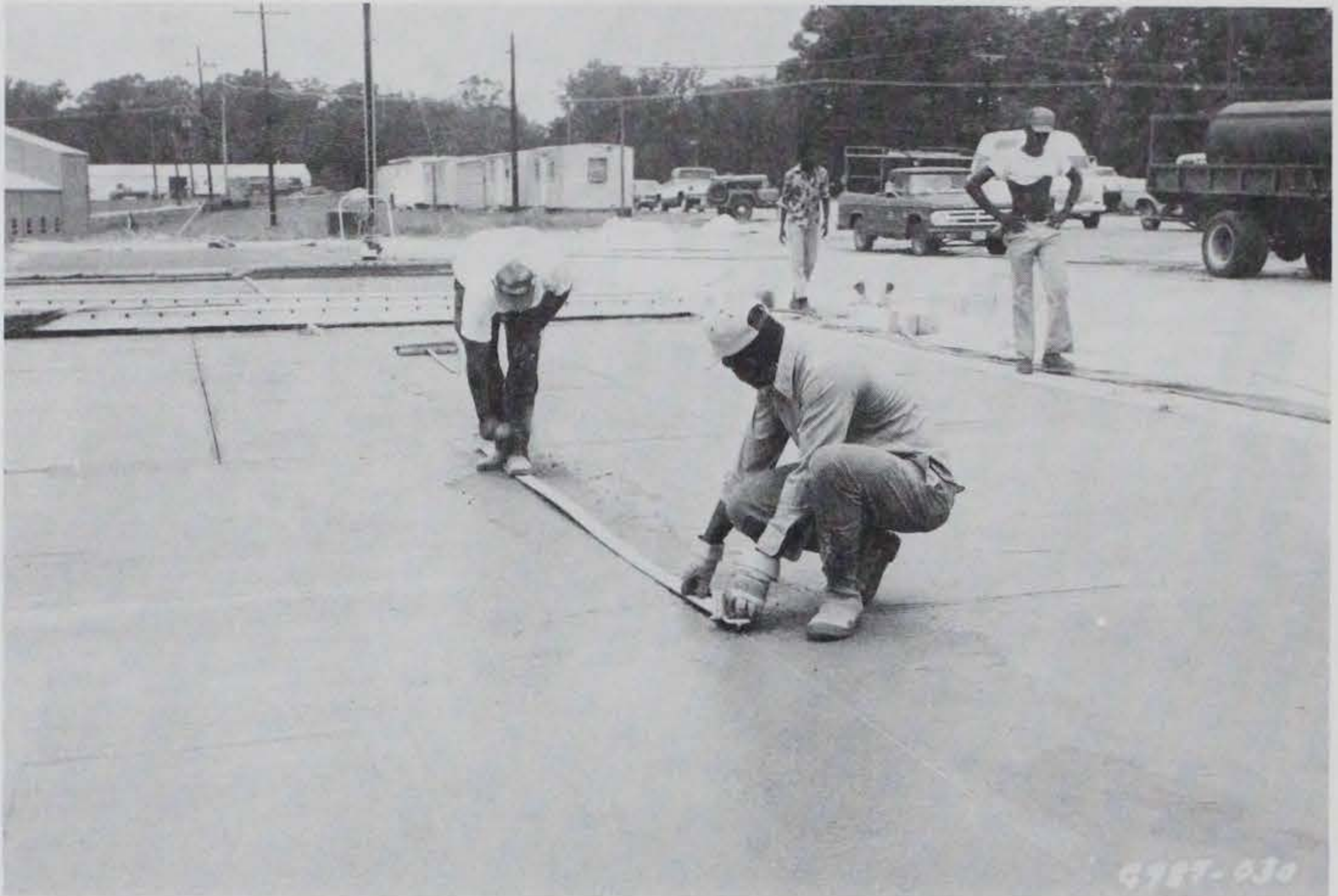
Photo 7. Forming weakened plane joints in items 1-10
