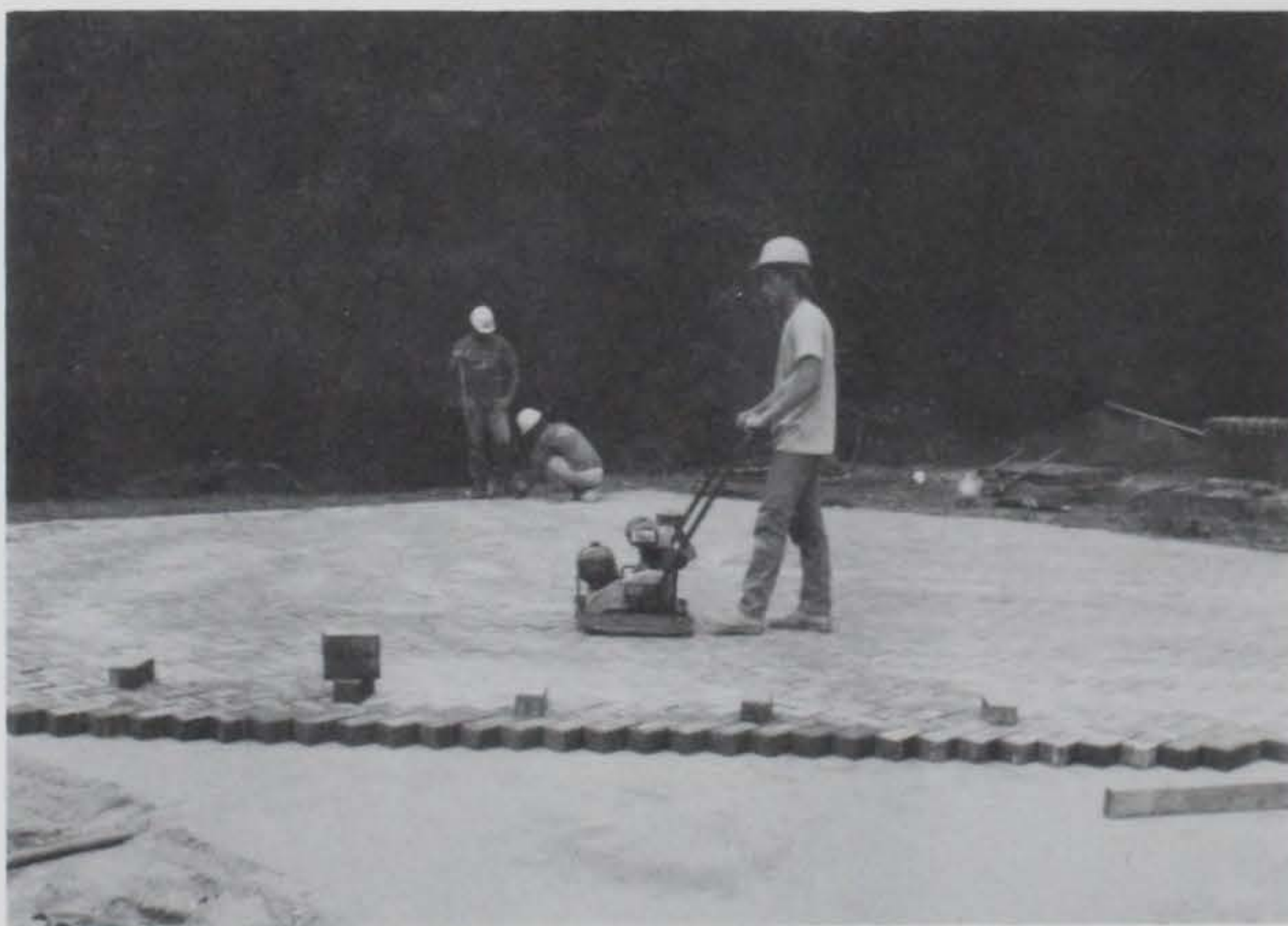
Figure 8. Initial compacting of paving blocks
