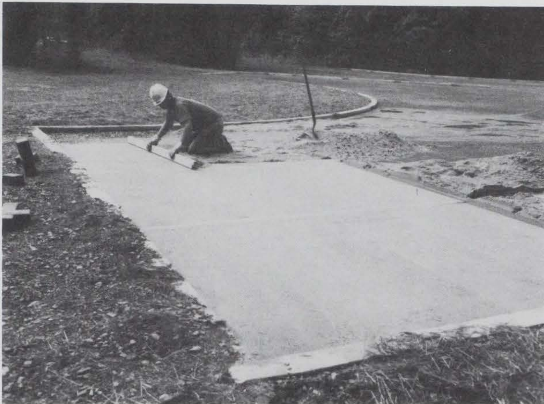
Figure 5. Screeding bedding sand
