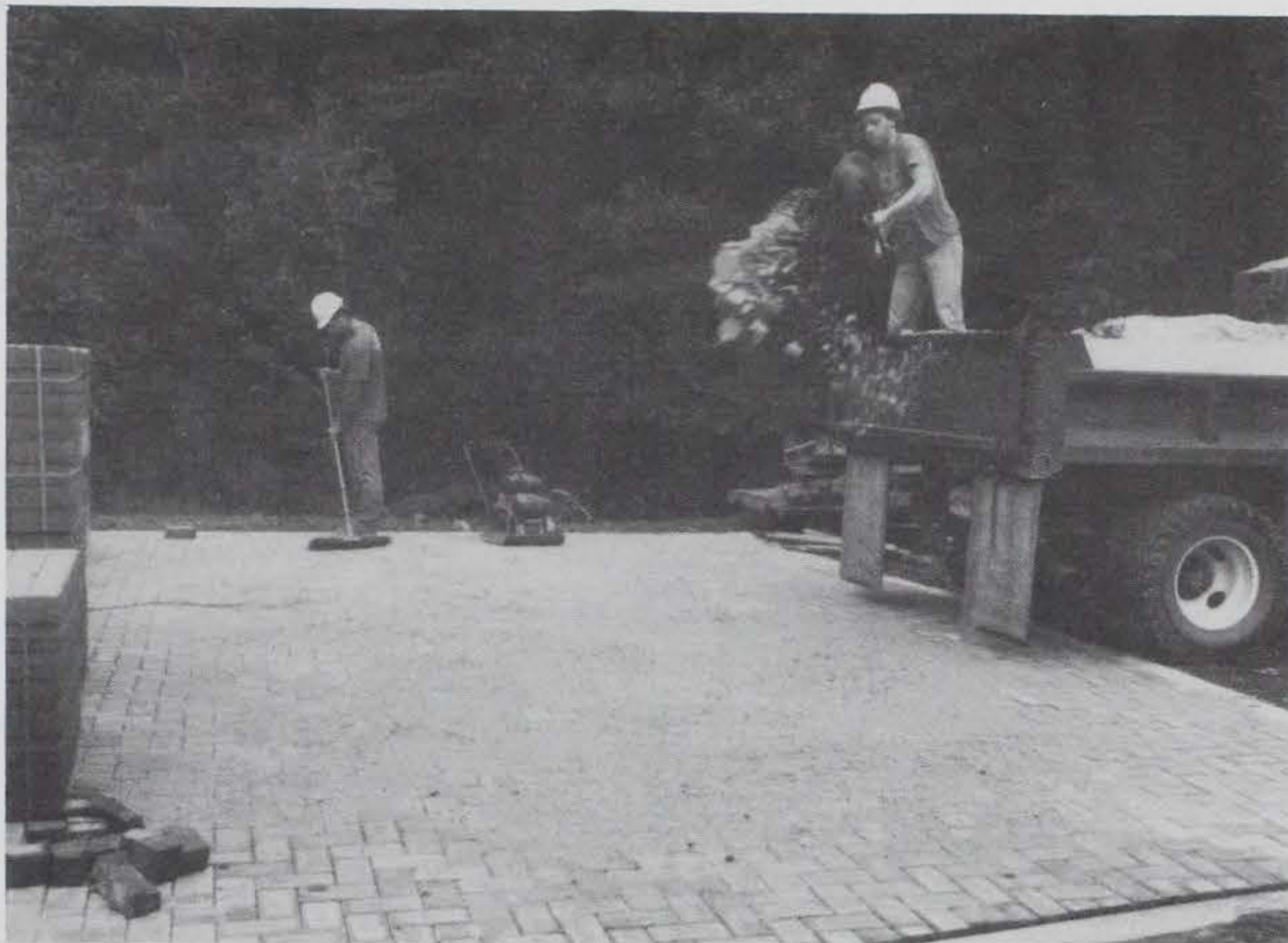
Figure 9. Spreading jointing sand over compacted paving blocks
