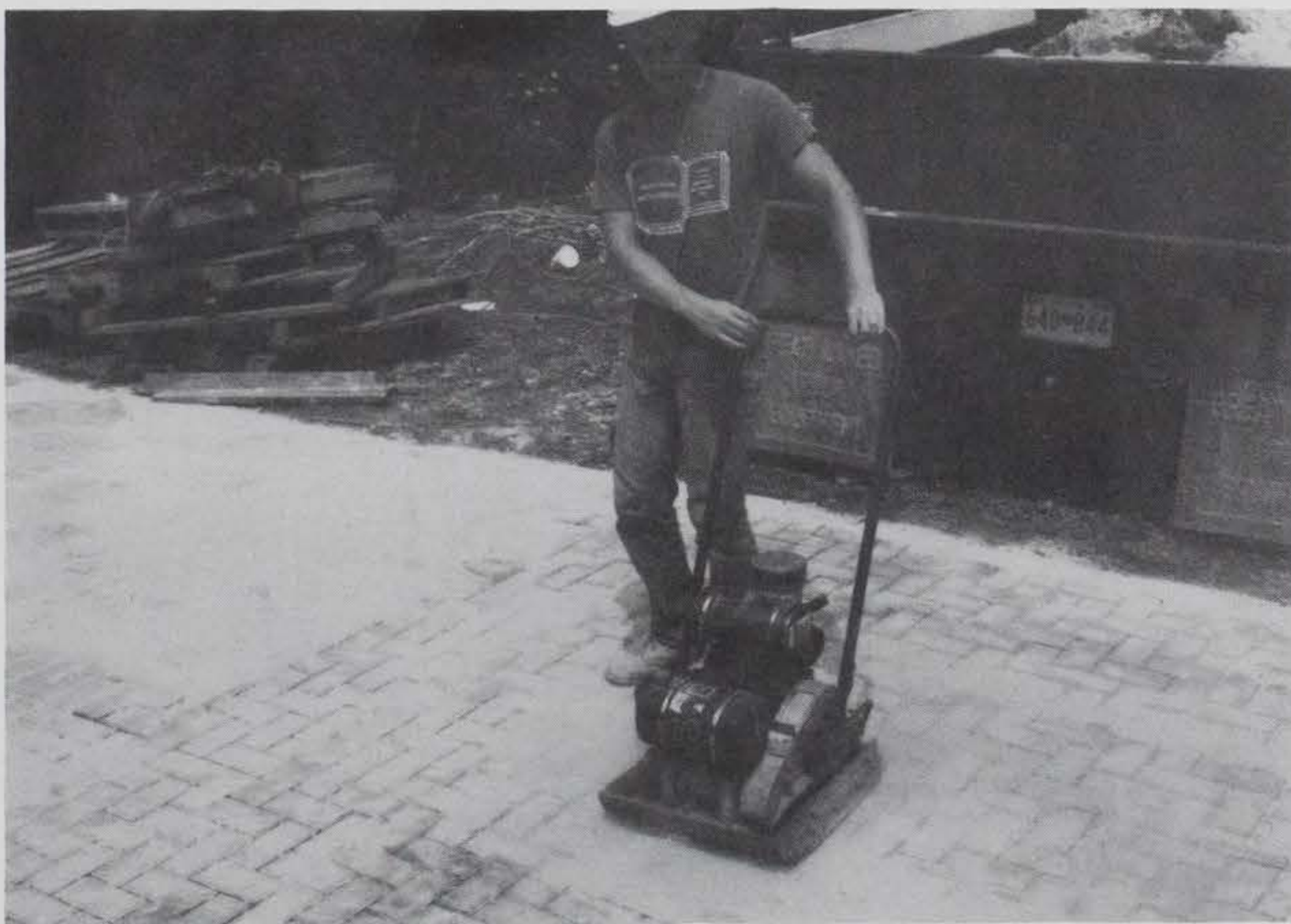
Figure 10. Vibrating jointing sand into paving block joints
