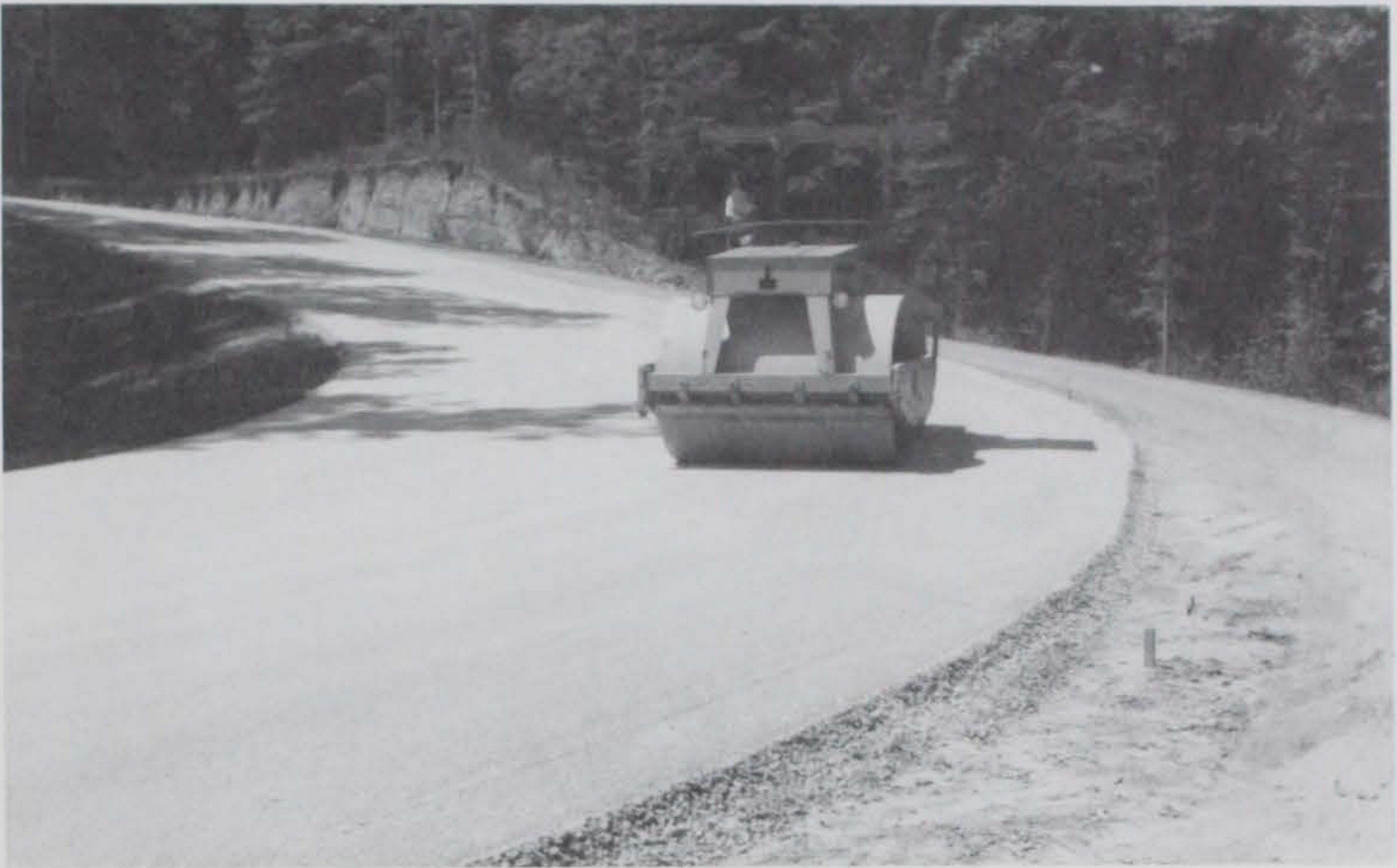
Figure 4. Compaction of the aggregate base material
