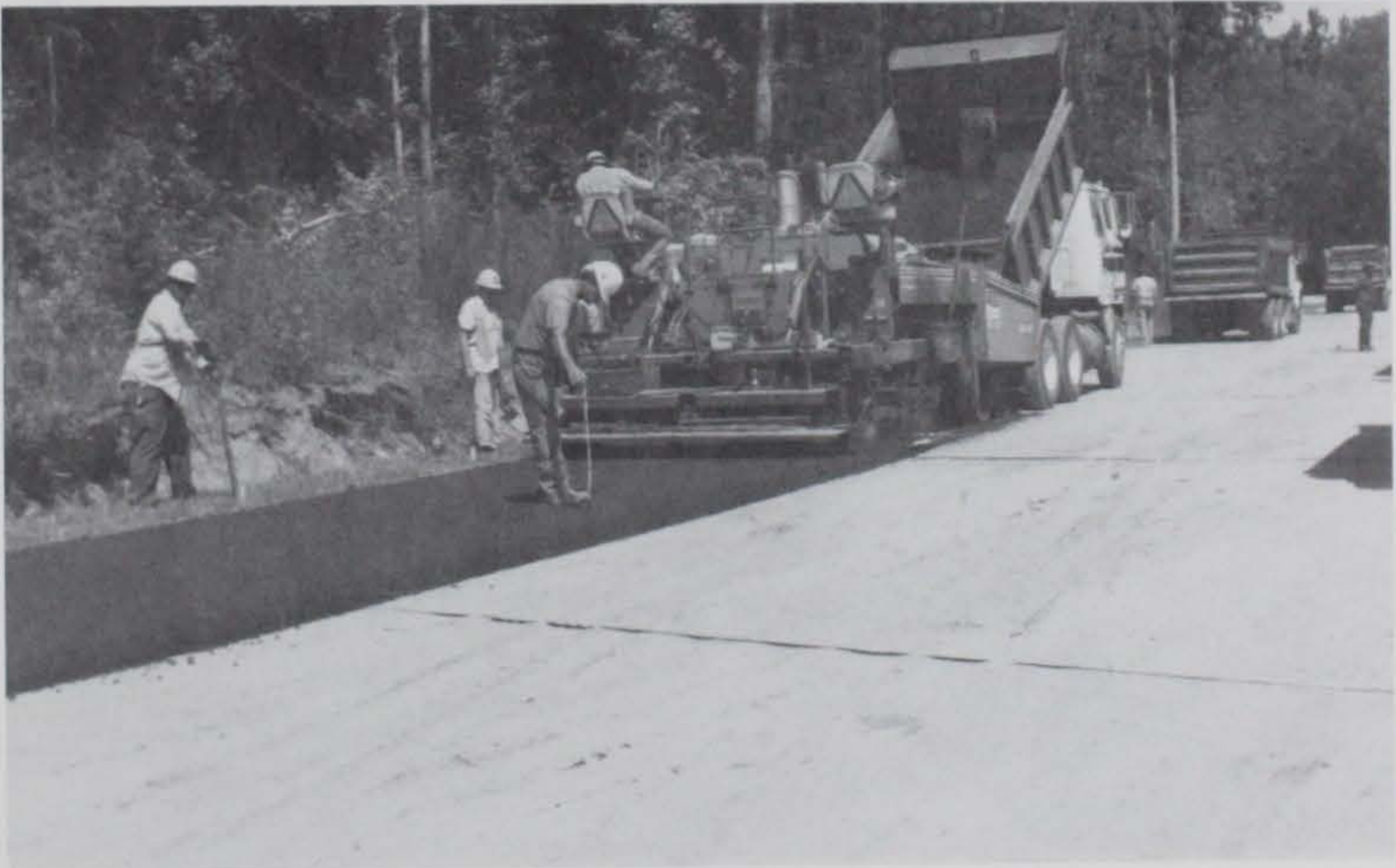
Figure 5. Placement of the asphalt concrete
