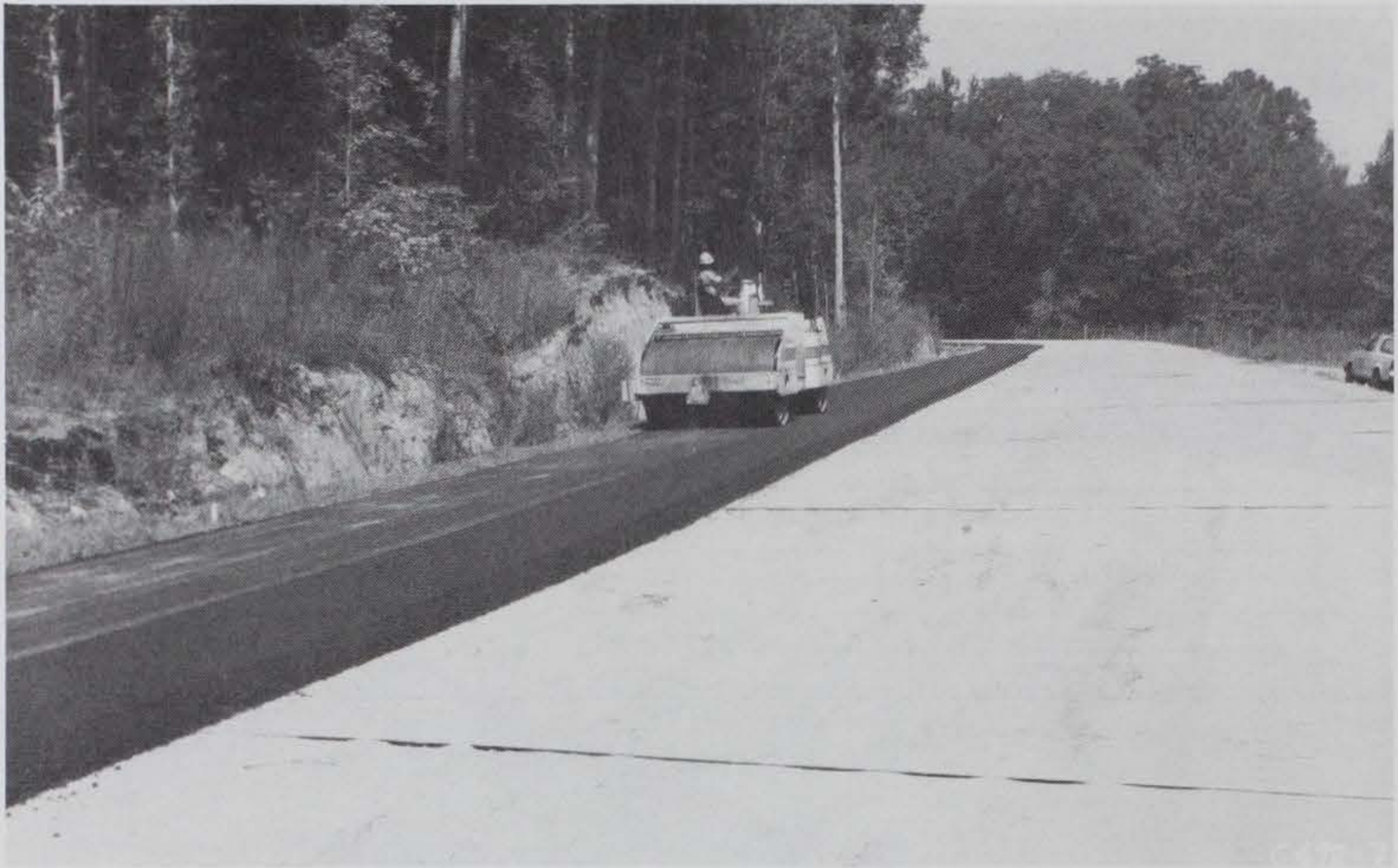
Figure 6. Breakdown rolling of the hot asphalt mix
