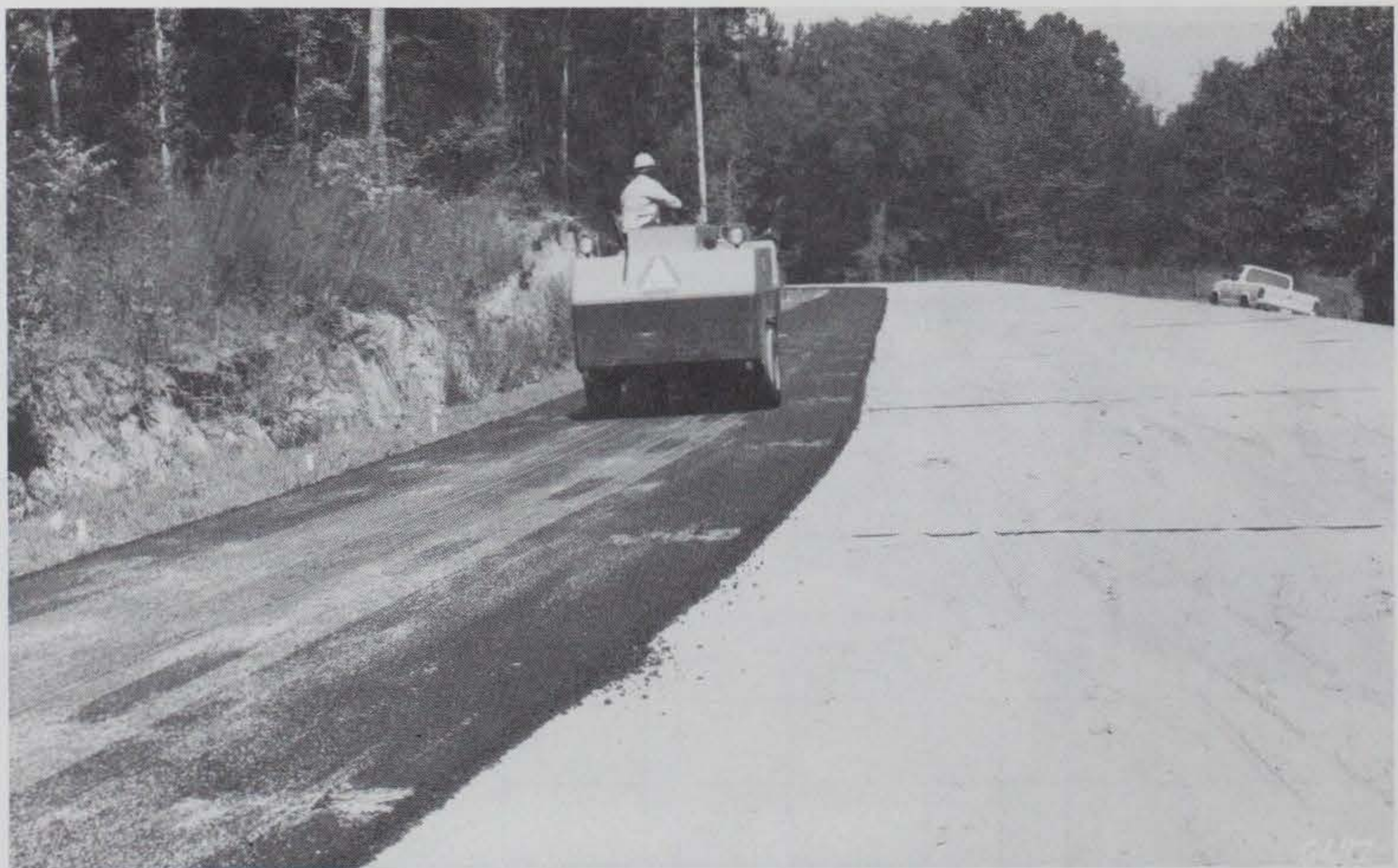
Figure 7. Compaction of the asphalt pavement
