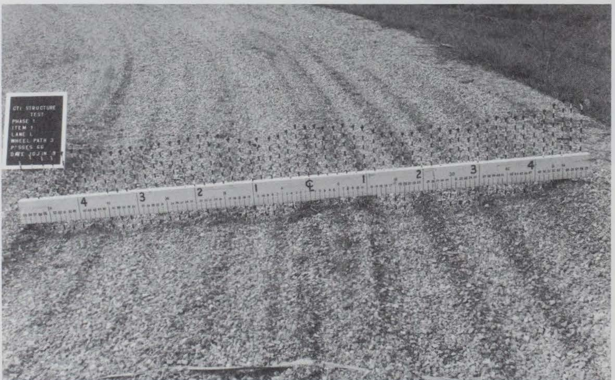
Figure 16. Low-tire-pressure lane, section 1, failure after 66 passes
